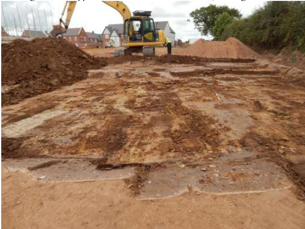
Figure 43: Stripped area on western side of Area 5, looking south
