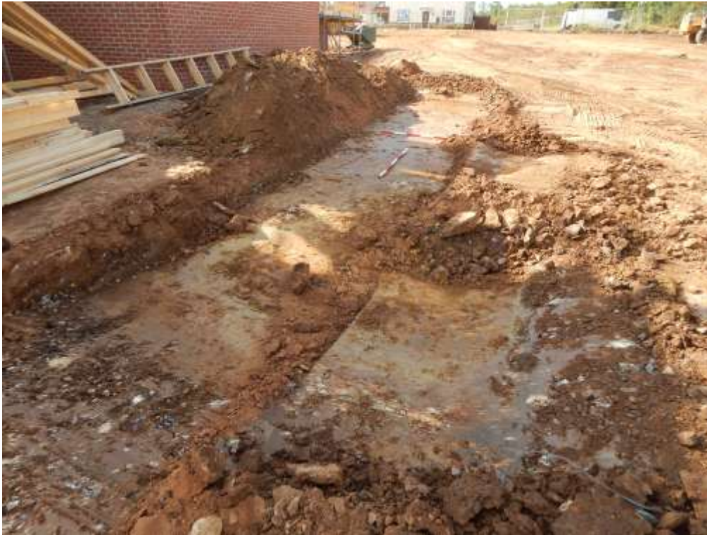
Figure 42: Stripped area on eastern side of Area 5, looking south-east
