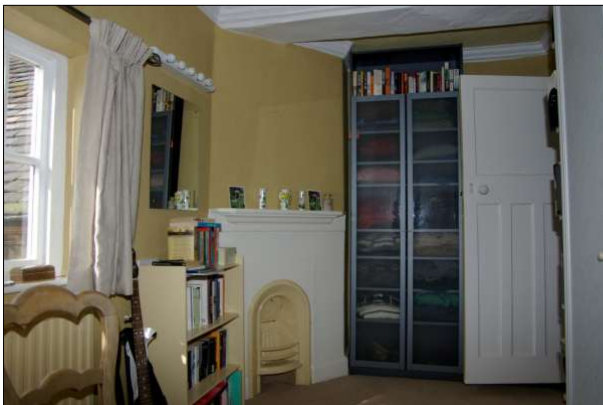
Figure 41. As above with cast-iron register plate fire-place, looking north.
