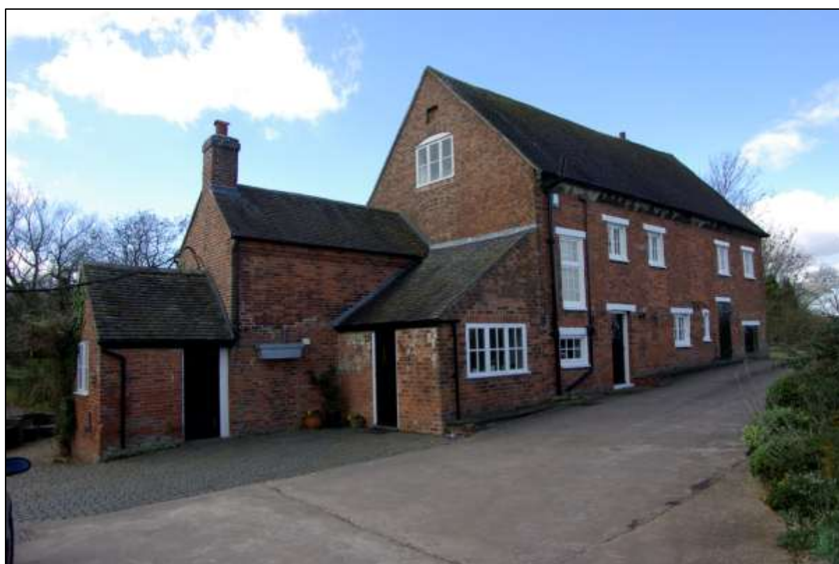
Figure 20. Front elevation, looking north-west.
