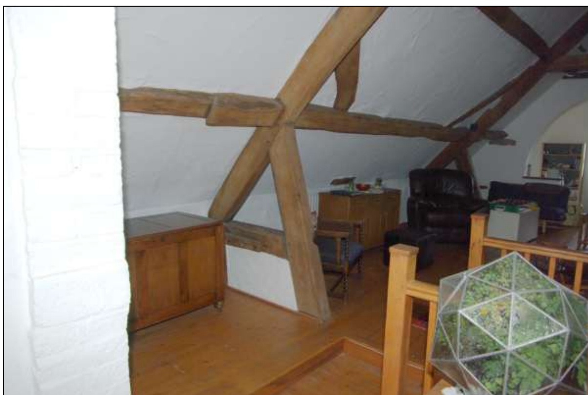
Figure 47. Interrupted tie-beam and wind-braces, looking south-east.
