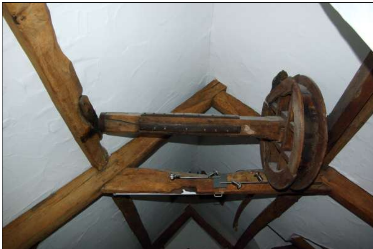
Figure 46. Timber pulley, part of sack hoist. Looking south.
