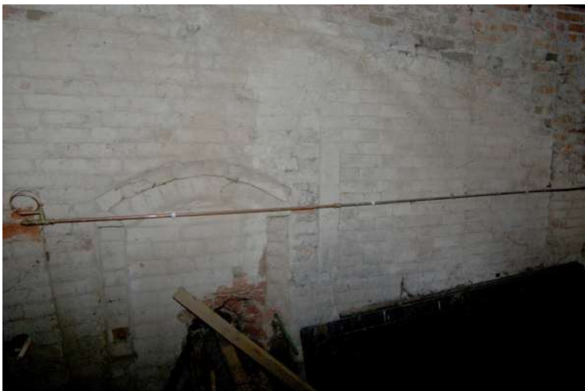
Figure 31. Axle for water-wheel and blocked openings in wheel-house wall, looking south.
