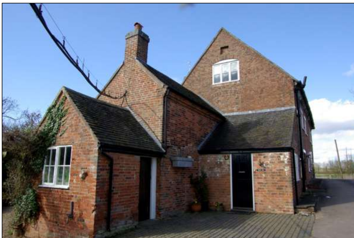
Figure 28. South-facing elevation, looking north.
