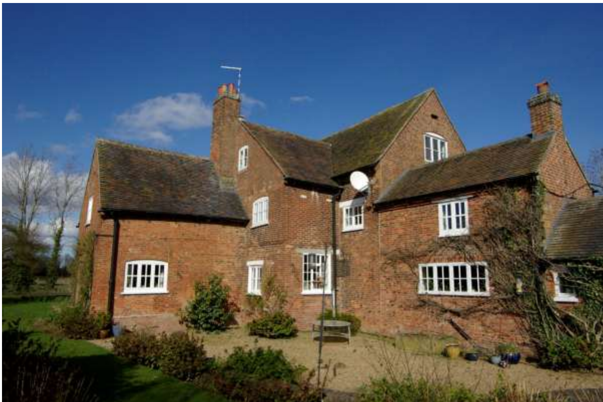
Figure 1. Temple Mill, rear elevation, looking south-west.
