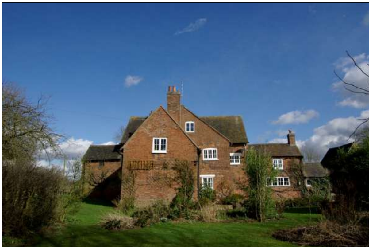
Figure 27. West-facing elevation, looking east.
