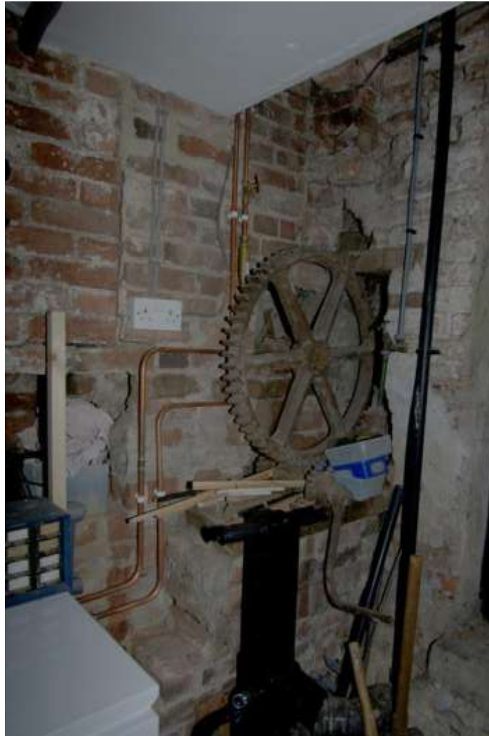
Figure 33. Turning wheel and handle for sluice-gate, in workshop, looking north-east.
