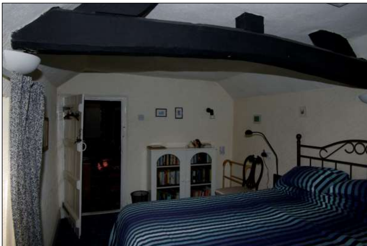
Figure 38. Bedroom over modern kitchen, with king-post roof truss, looking north.
