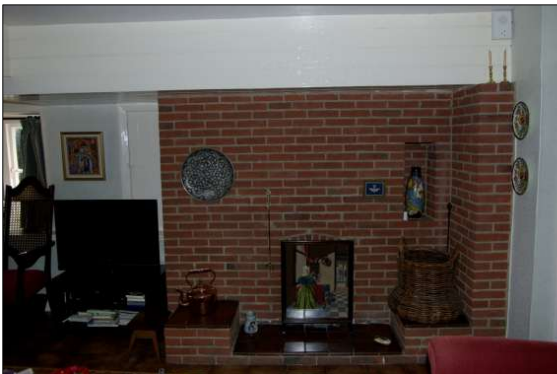
Figure 49. Brick fireplace of 1970, prior to removal, looking west.
