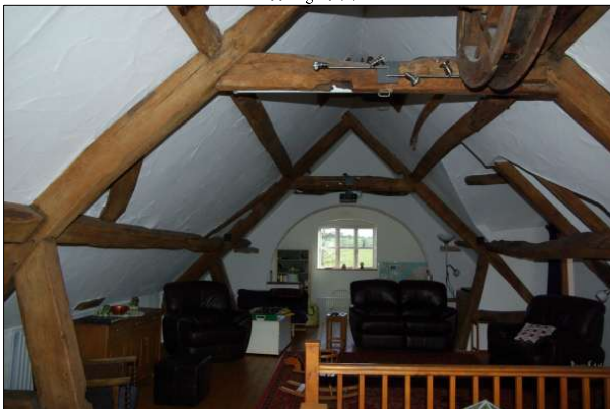
Figure 45. As above, looking south.
