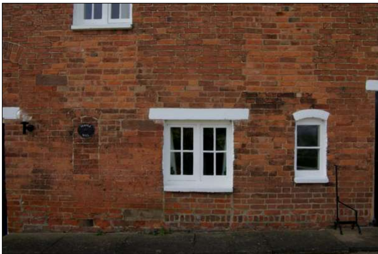
Figure 21. Front elevation, former doorway in central position, looking west.
