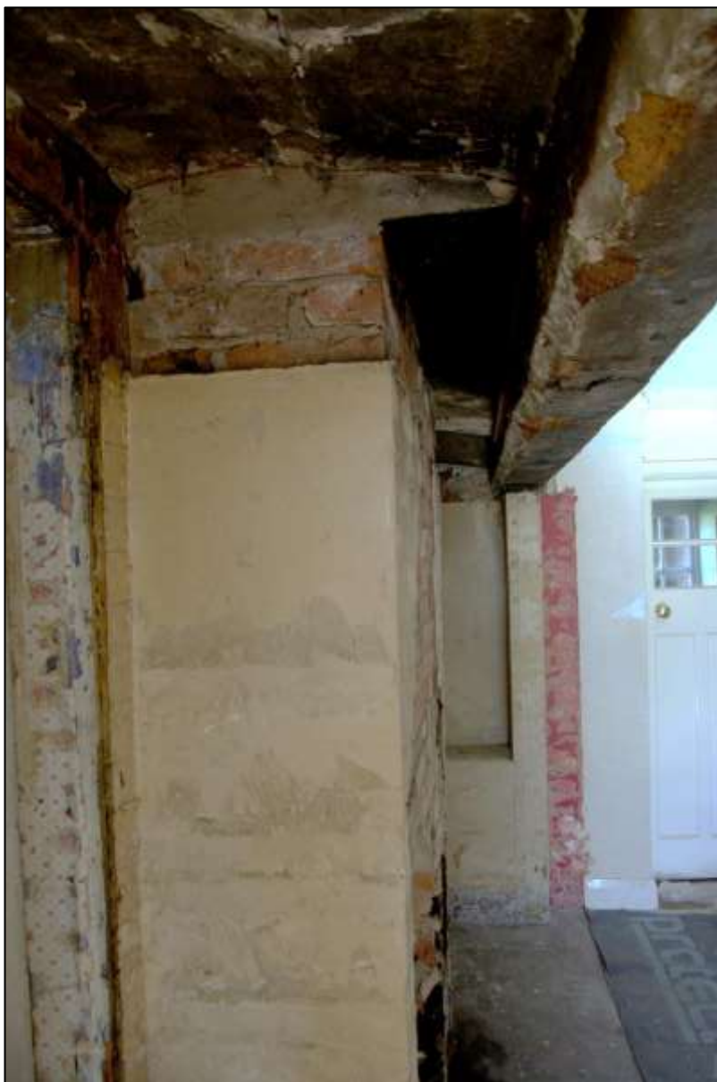
Figure 53. 19th-century brick stack, with 18th-century bricks and mortar infilling up to 18th century structural arch above. Looking north.
