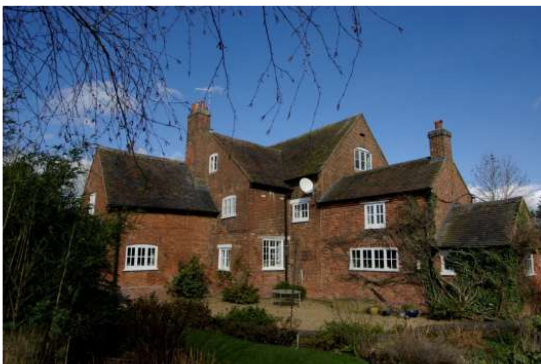
Figure 8. SW view of Temple Mill, present day.
