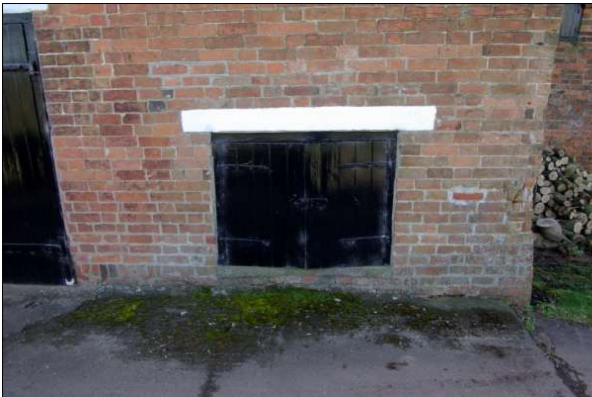
Figure 29. Shuttered access to wheel-house, looking west.
