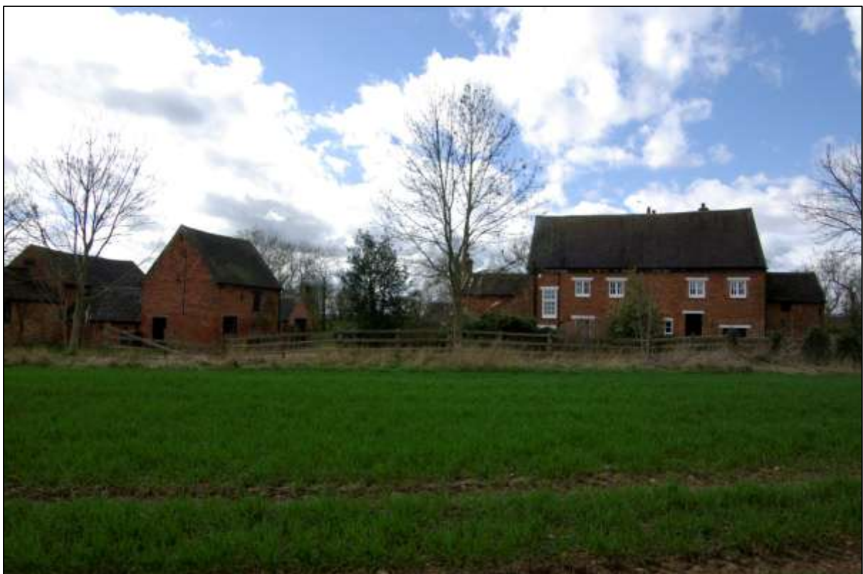
Figure 6. NE view of Temple Mill, present day.
