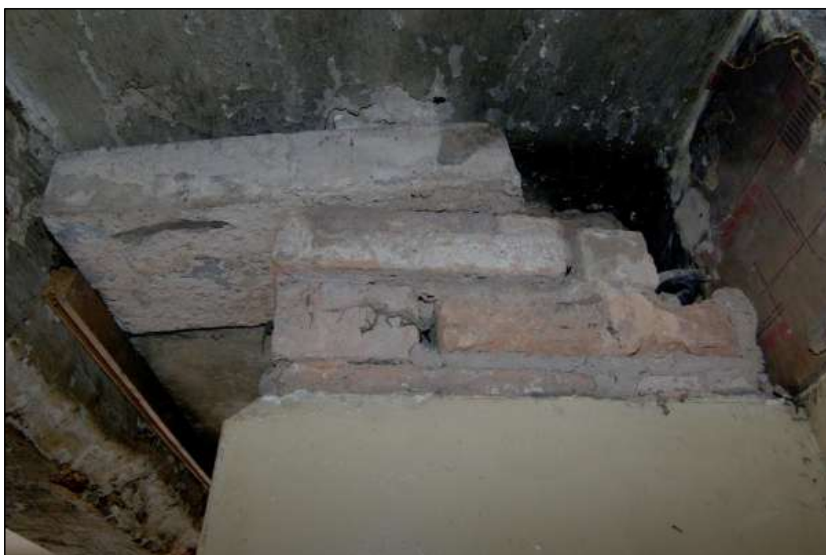
Figure 52. Roughly mortared 18th century brick infill between 19th century stack and 18th brick arch above. Looking south.
