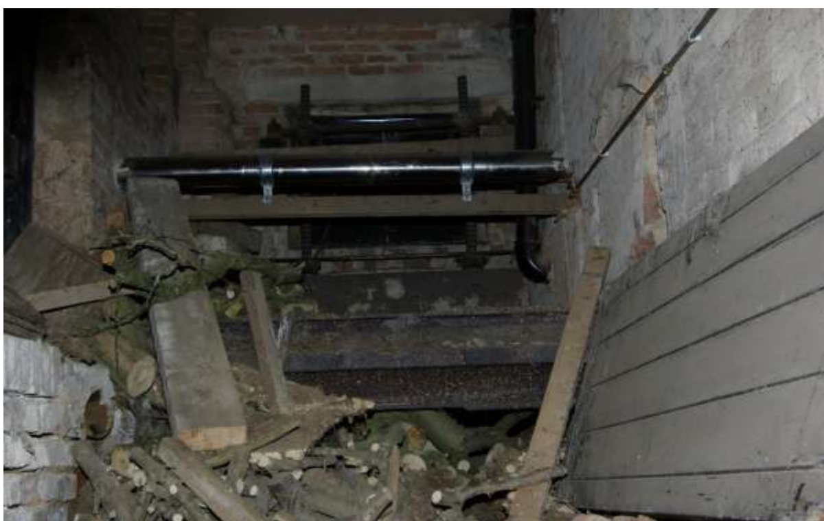
Figure 32. Wheel house, looking east towards axle and sluice gate.
