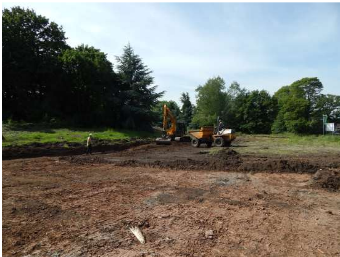
Plate 1: Work in progress stripping Area 2, looking south-west
