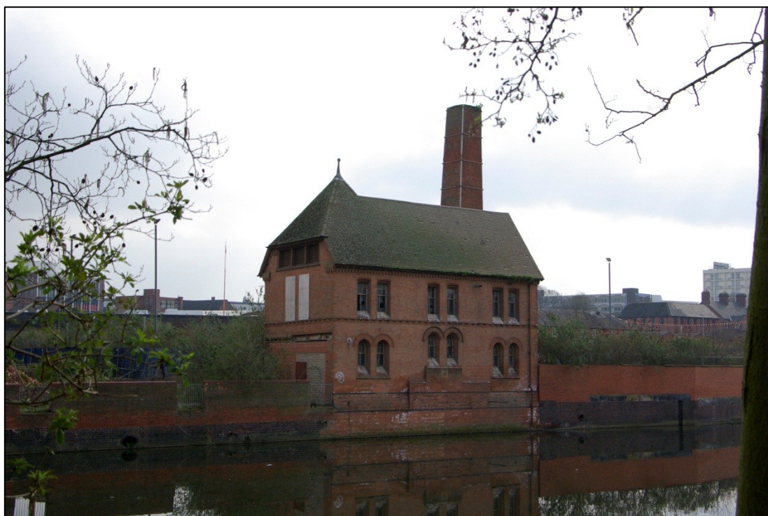
Figure 21. Pump House, looking south-east.
