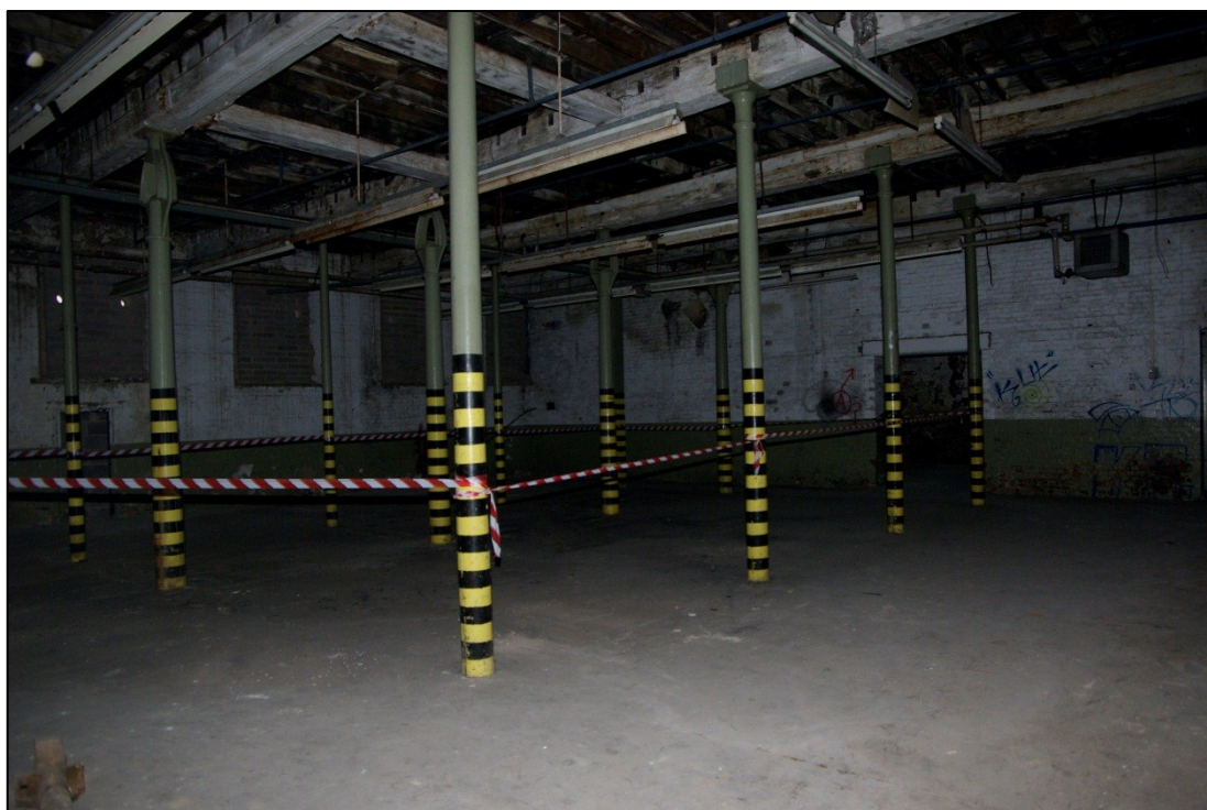
Figure 12. Friars Mill interior, ground floor. Looking north-west.
