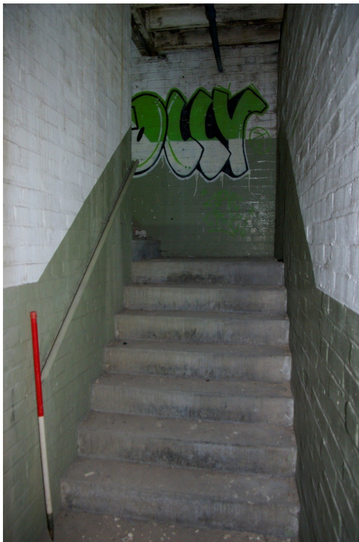
Figure 16. Friars Mill, first floor staircase, looking west.
