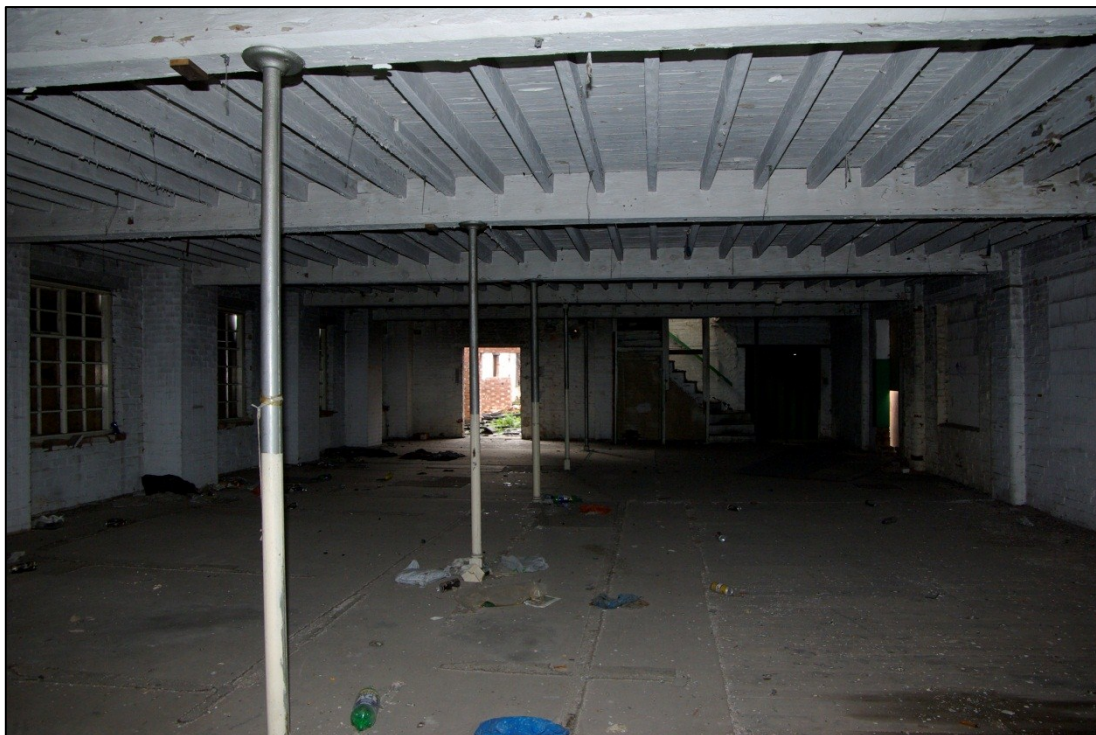
Figure 37. Bath Lane Mill interior, first floor, looking south.
