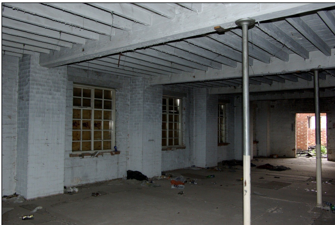
Figure 38. Bath Lane Mill, first floor, timber multi-pane window frames, looking south-east.
