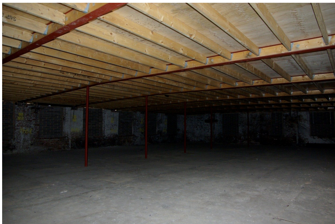
Figure 18. Friars Mill, second floor, looking north-west.
