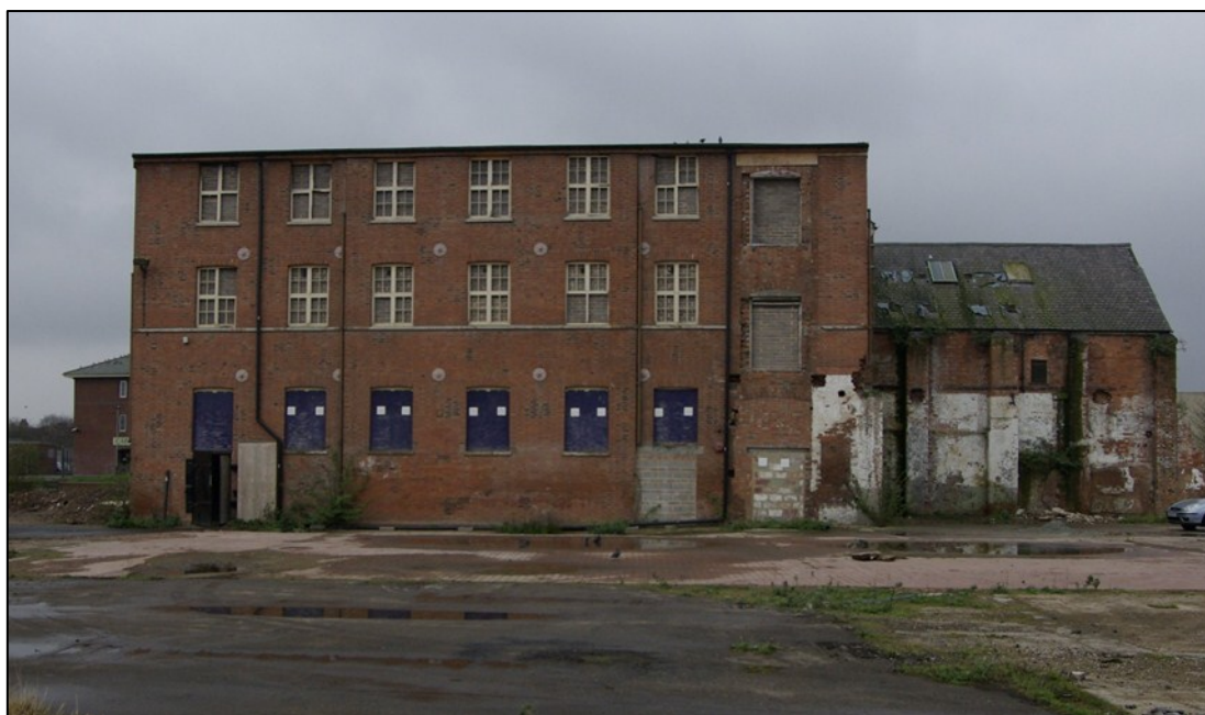
Figure 8. Friars Mill and Boiler House, looking west.
