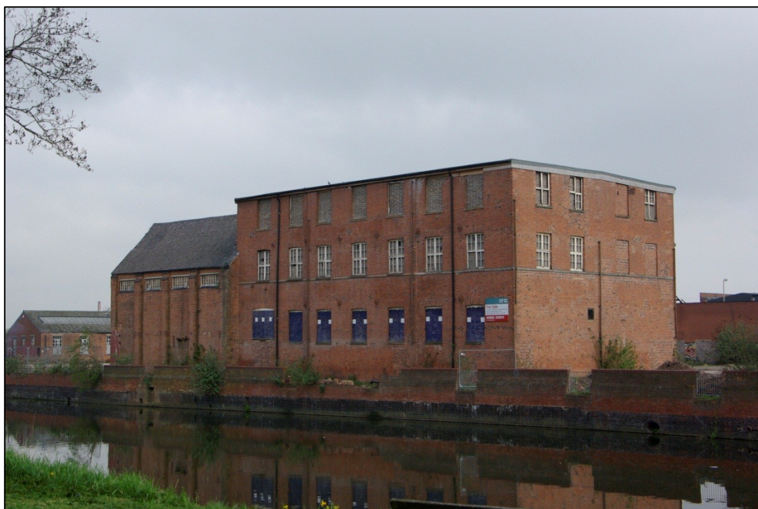
Figure 7. Friars Mill and Boiler House, looking north-east.
