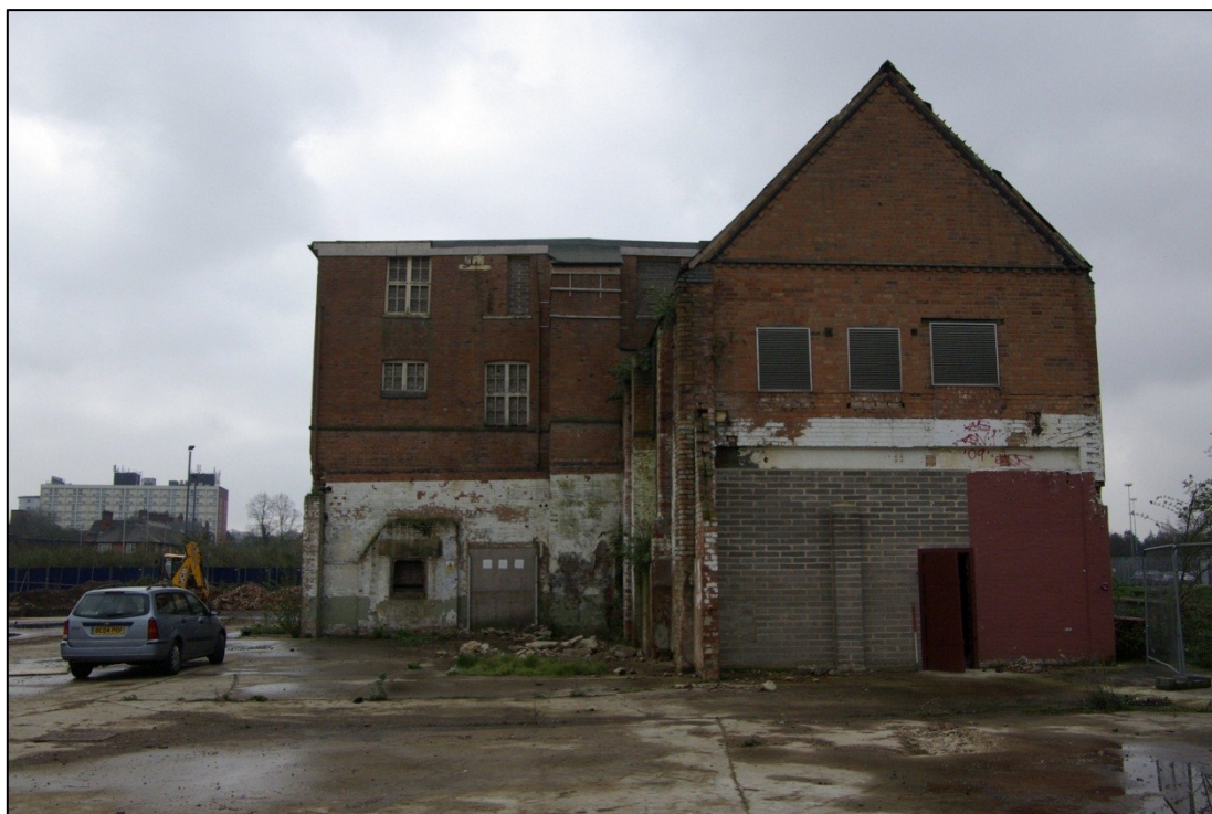
Figure 9. Friars Mill and Boiler House, looking south.
