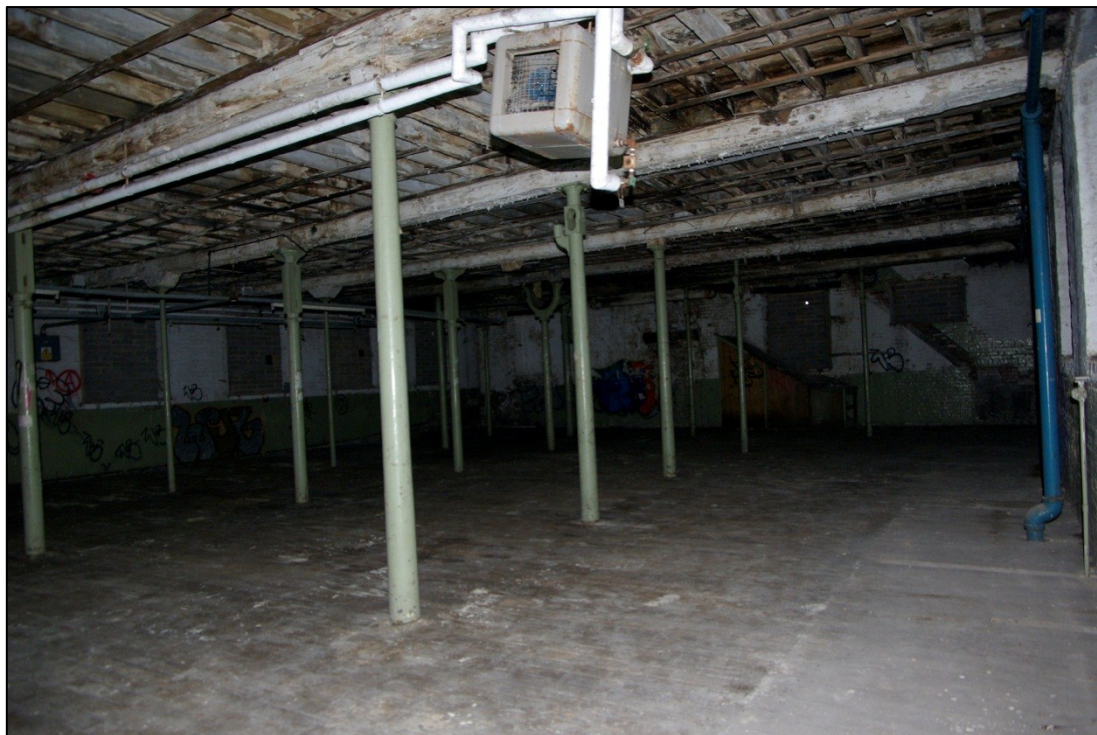
Figure 15. Friars Mill, first floor, looking north-west.
