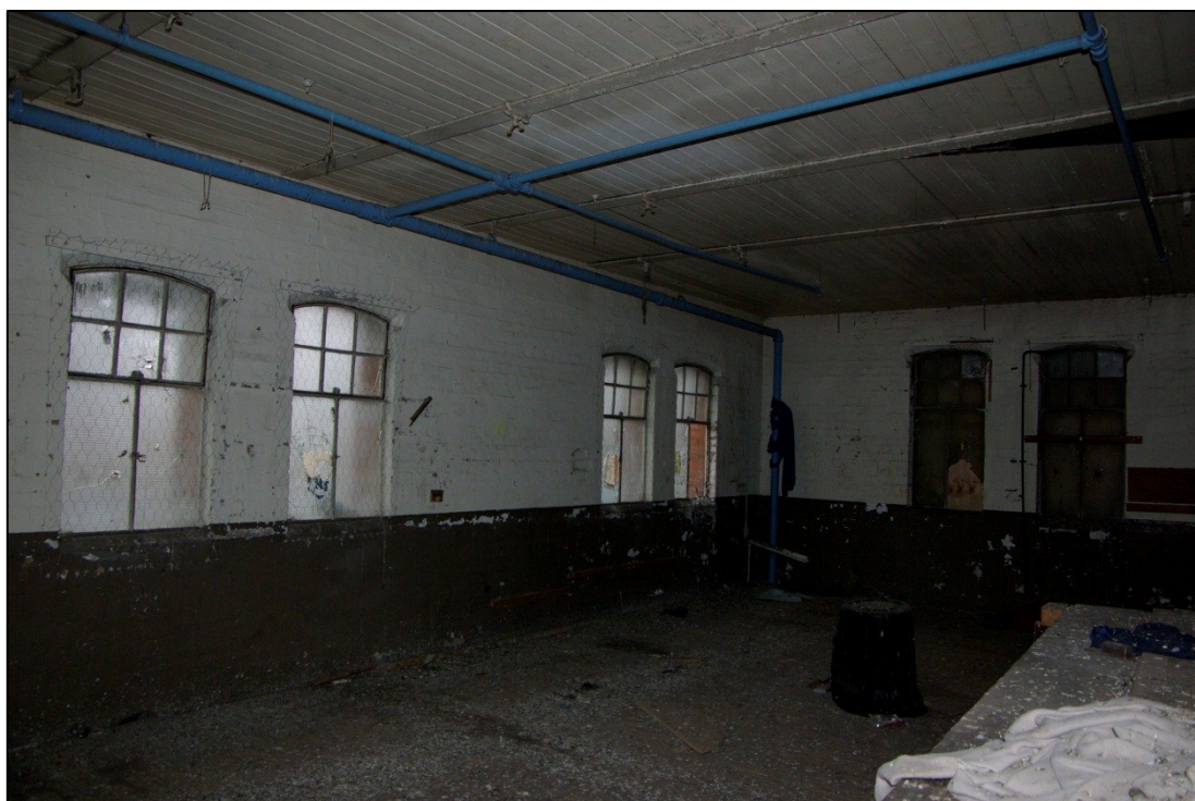
Figure 24. Pump House interior, first floor, looking north-west.
