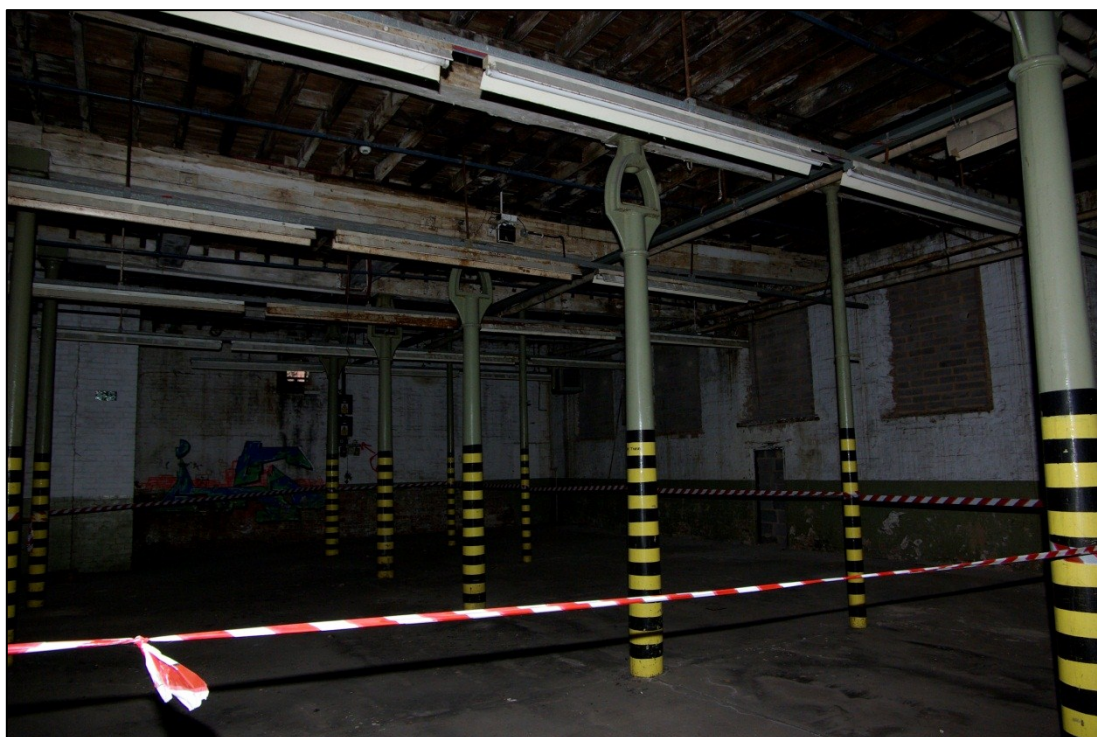
Figure 13. Friars Mill interior, ground floor, looking south-west.
