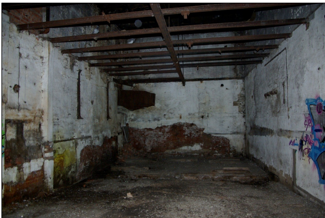
Figure 10. Boiler House interior, looking south.
