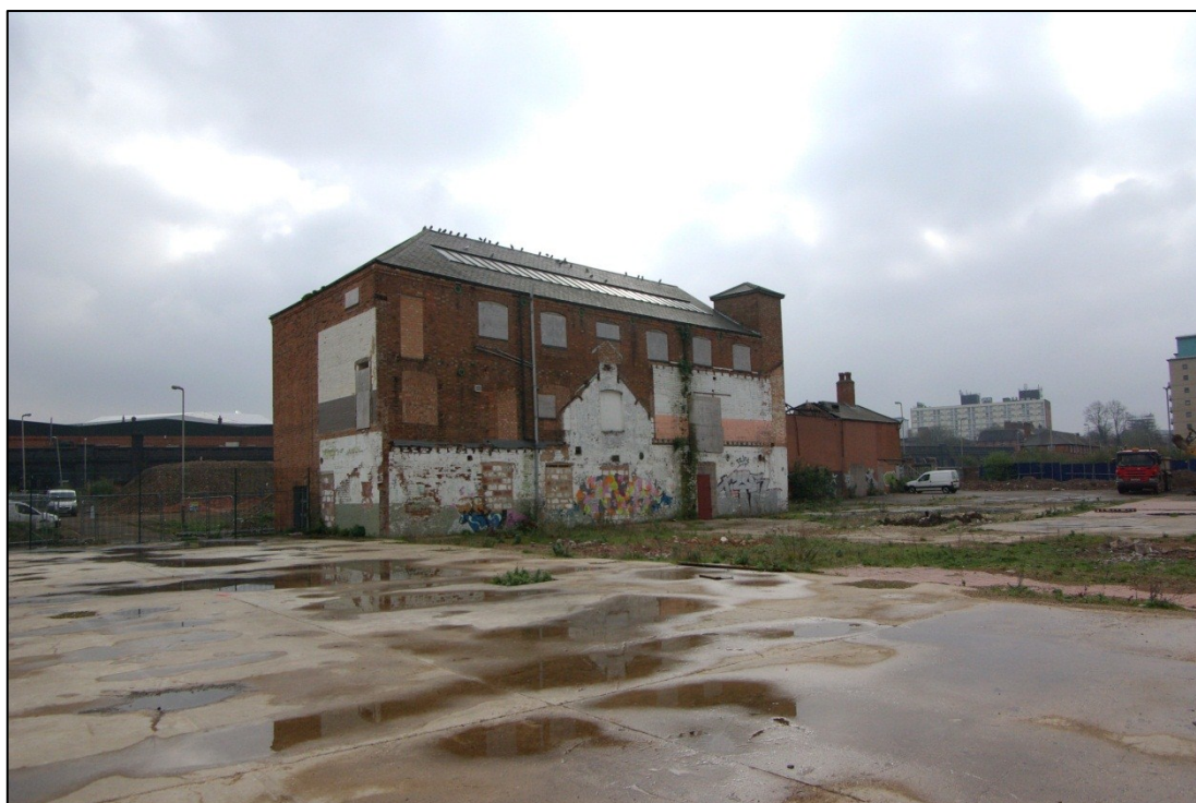
Figure 32. Bath Lane Mill, looking south-east.
