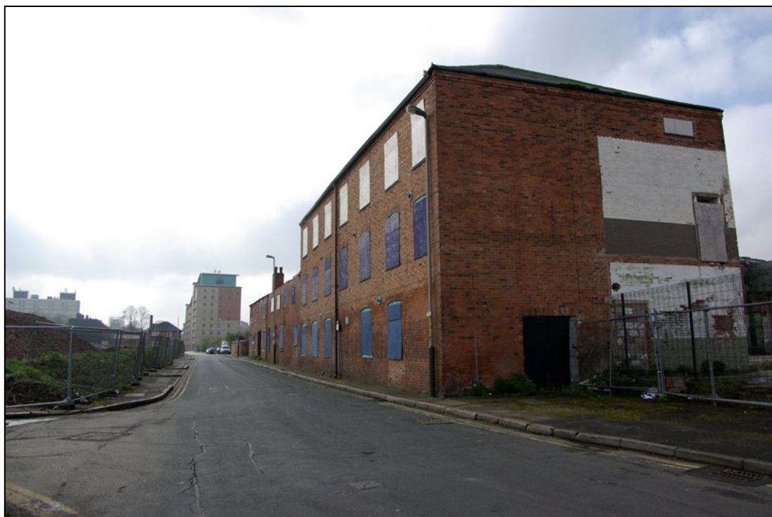
Figure 31. Bath Lane frontage, looking south.
