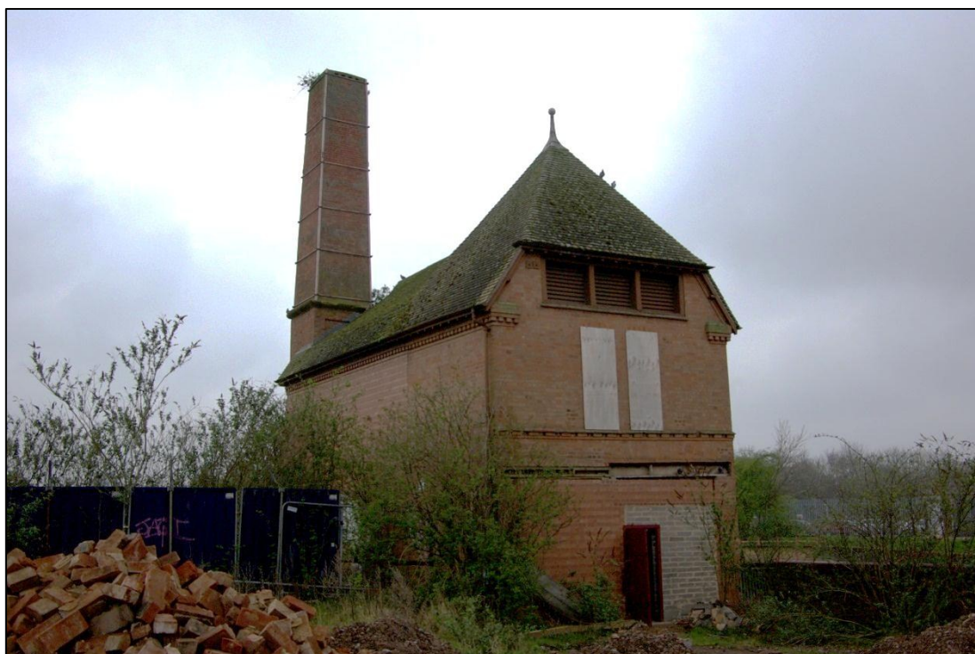
Figure 22. Pump House, looking south-west.
