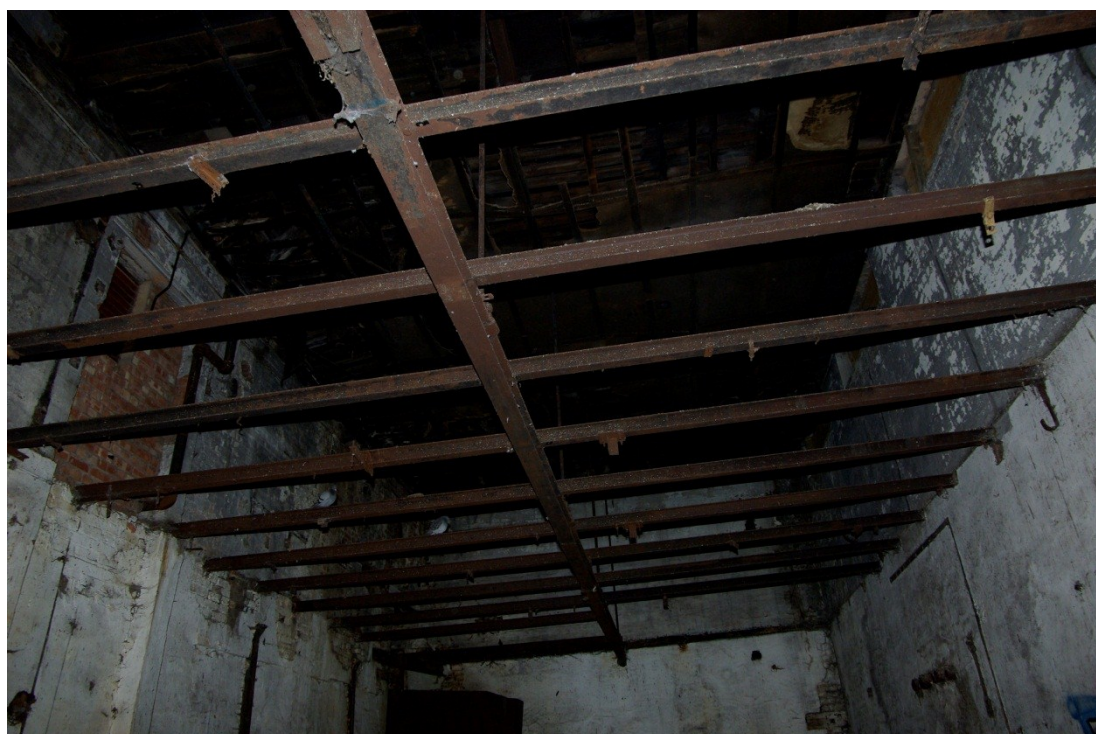
Figure 11. Boiler House, first floor ceiling structure, looking south.
