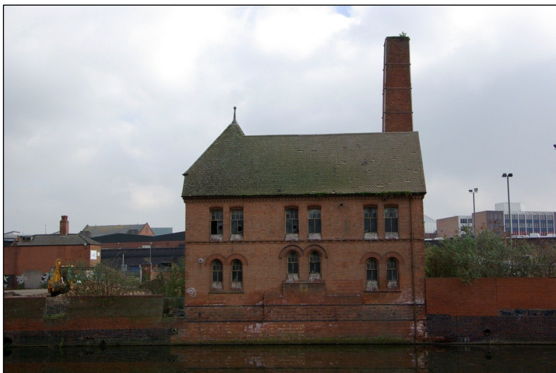
Figure 20. Pump House, looking east.
