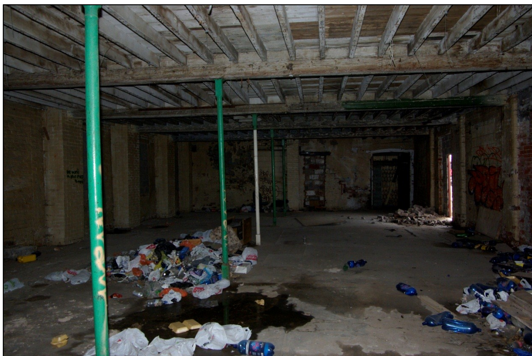
Figure 35. Bath Lane Mill, ground floor interior. Looking north.
