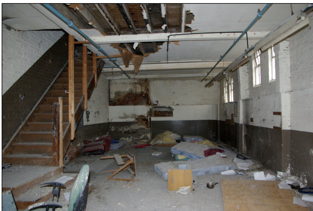
Figure 23. Pump House interior, ground floor, looking south.
