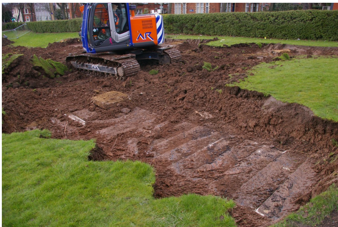
Figure 12 Exposed shelter roof, Tunnel F Looking north. Note capped ventilator shaft near to vehicle track.
