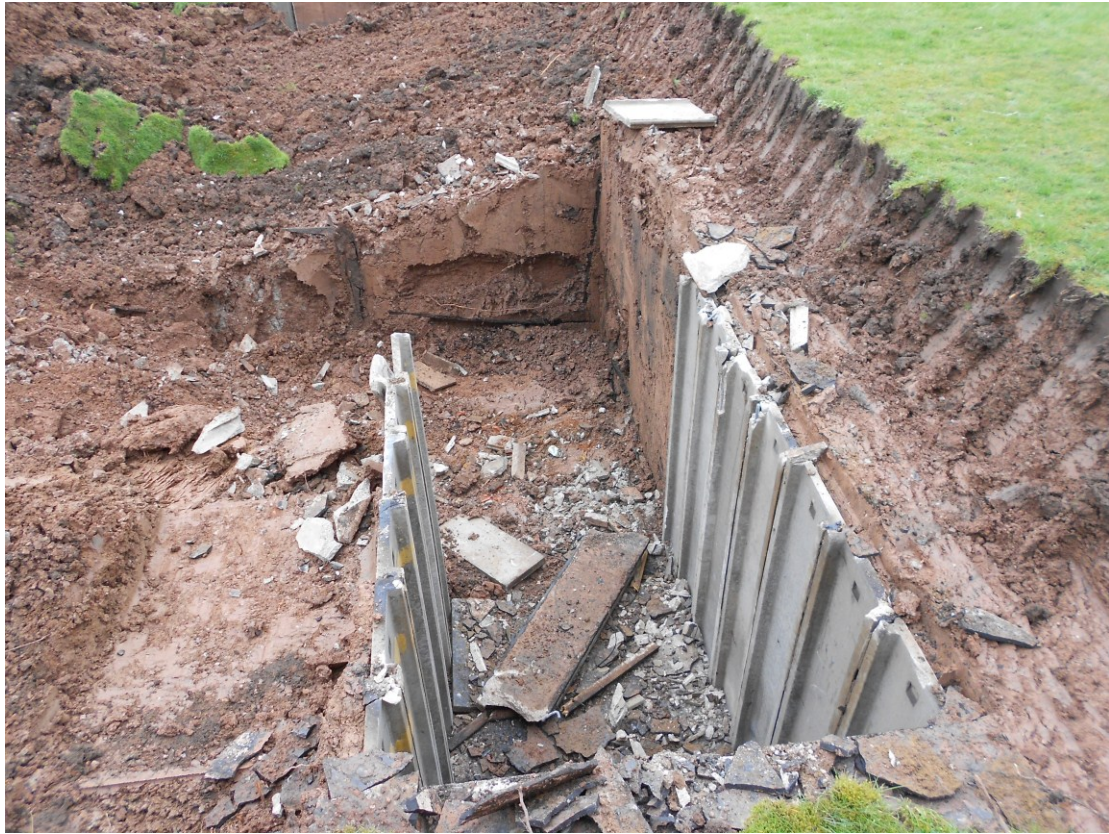
Figure 17 Tongue and groove joints on wall panels
