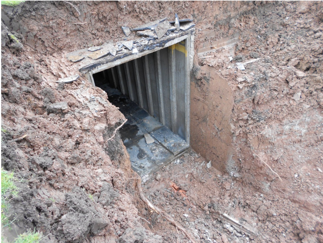
Figure 19 Tunnel E floor slabs near to University Road Looking south
