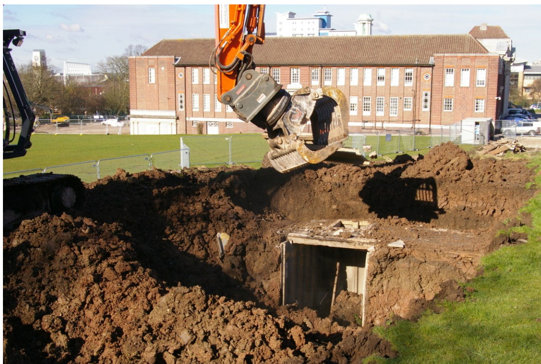
Figure 10 Demolition of Tunnel A Looking west
