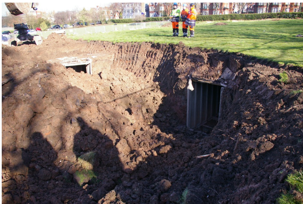
Figure 16 Partial demolition of Tunnel B Looking north
