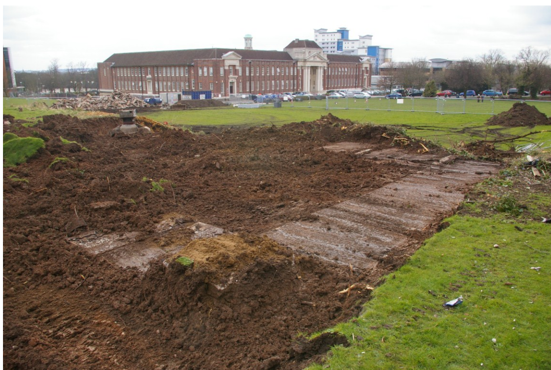
Figure 13 Tunnel D roof being exposed Looking west
