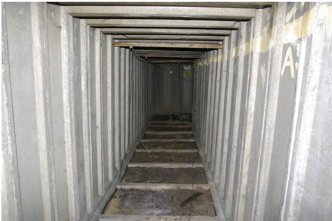
Figure 18 Tunnel A Looking south east. Note concrete spacers on floor
