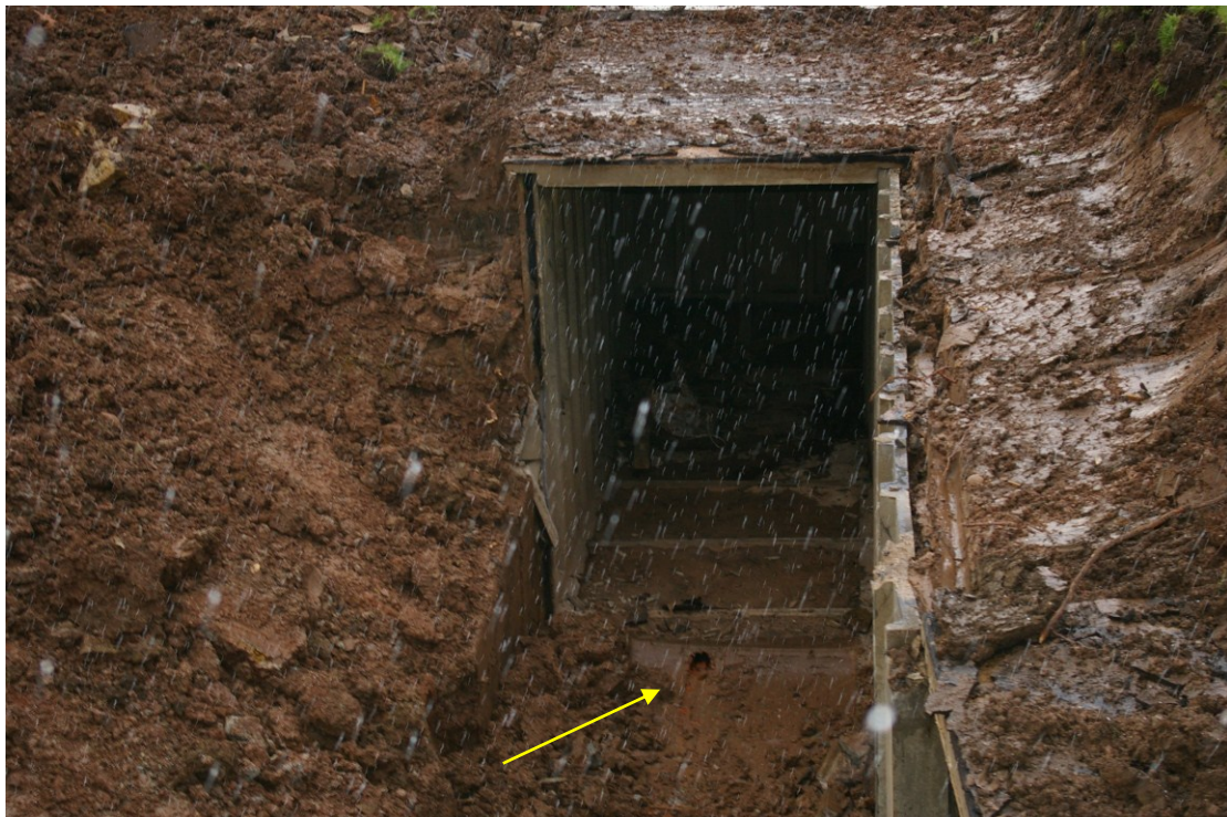
Figure 20 Drain in Tunnel F/G Looking north east
