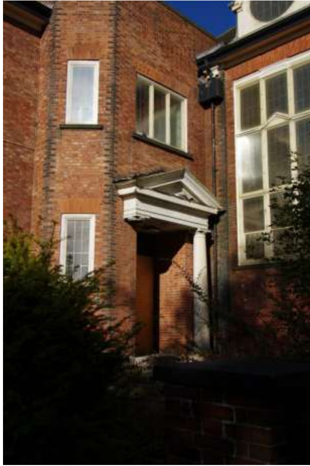
Figure 12 Detail of one of the entrance porches, looking north-west
