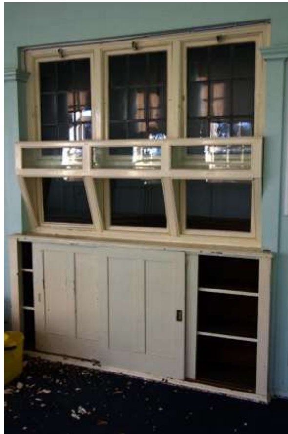
Figure 25 Example interior classroom windows, facing inward to corridor and Hall
