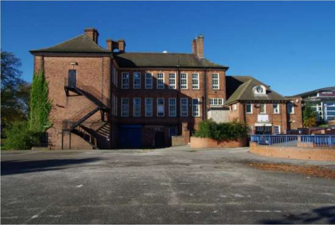
Figure 14 East elevation, looking west
