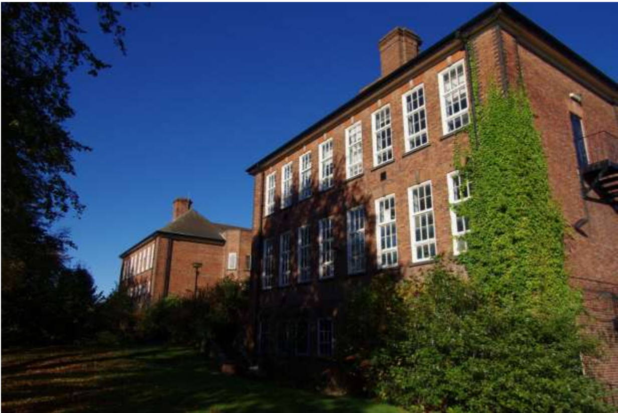
Figure 13 South elevation, showing advanced wings, looking north-west
