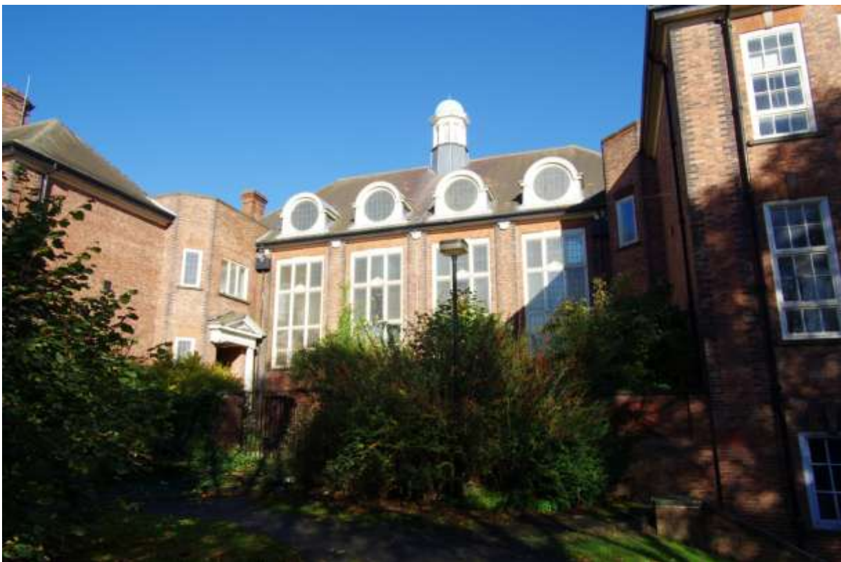
Figure 11 South façade, central, looking north
