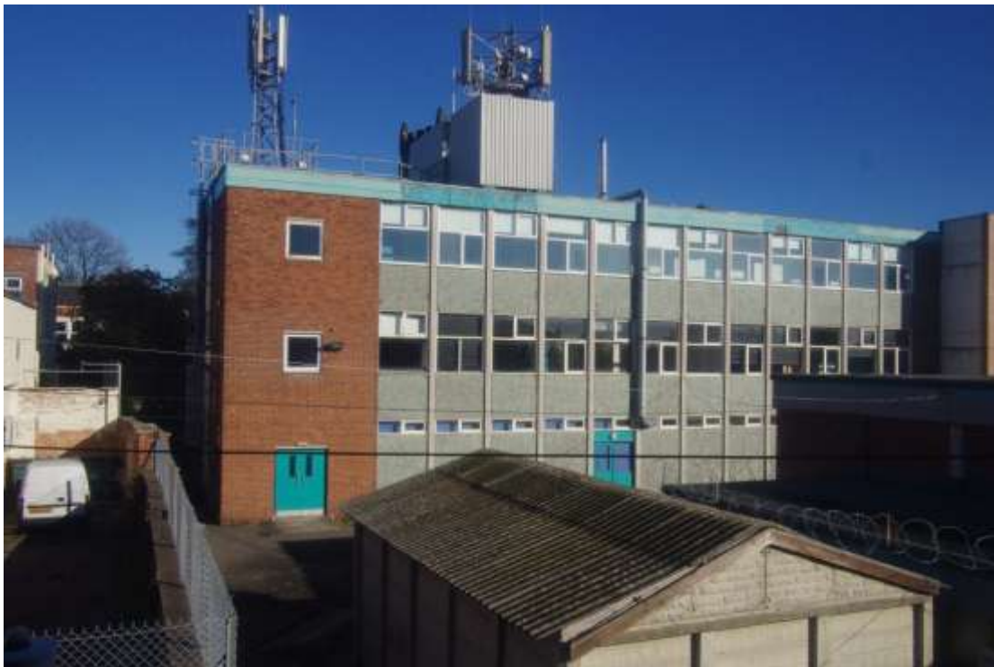
Figure 31 Science block, from the south
