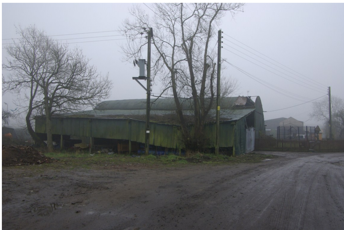
Figure 29 Metal barn to north-west of farmhouse and brick barn Looking east
