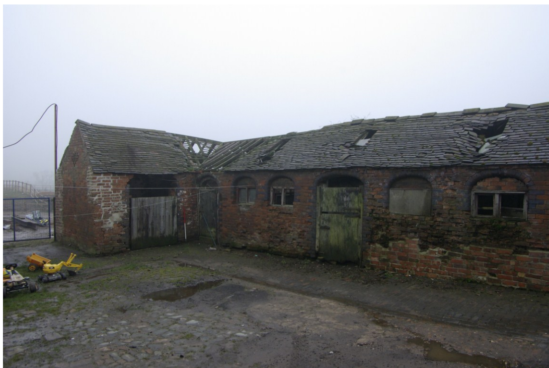
Figure 27 Stables, north-west facing elevation, east corner Looking south-east. 1m scale
