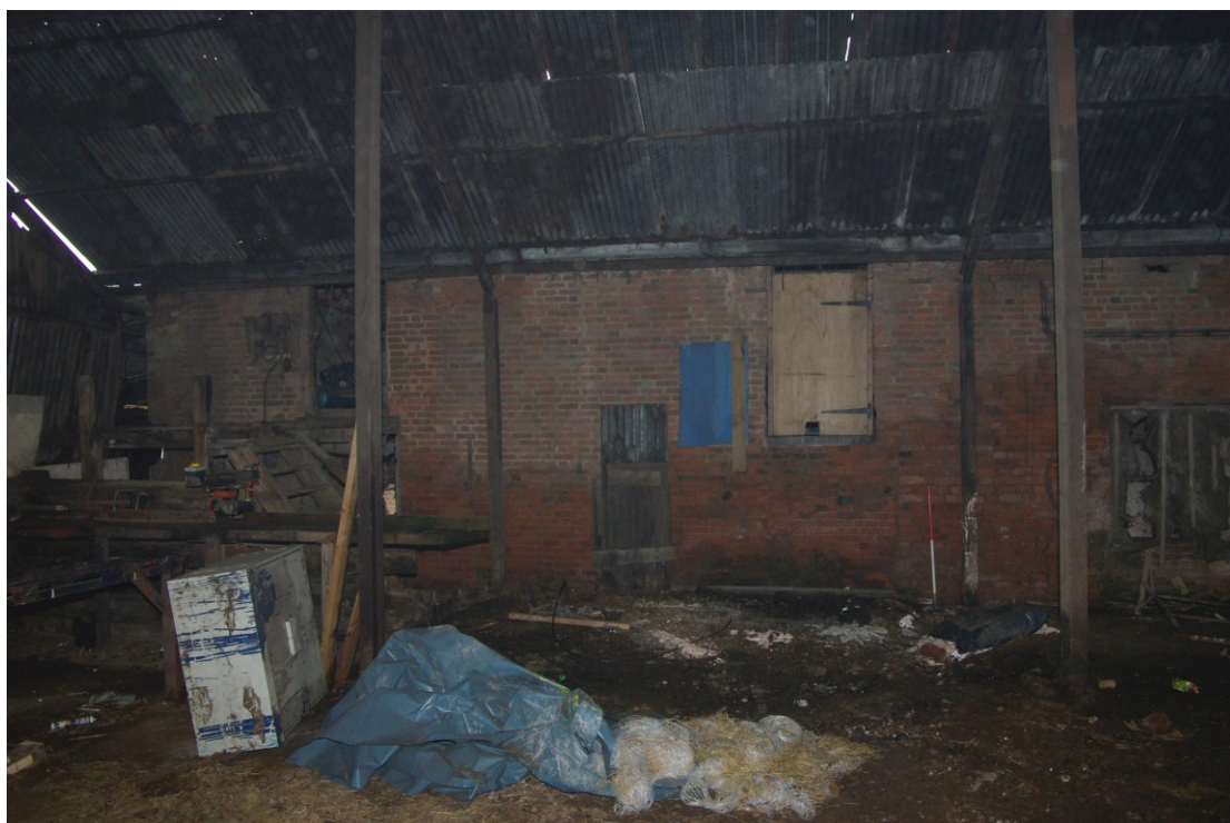
Figure 18 Barn range, north-west facing elevation Looking south-east
