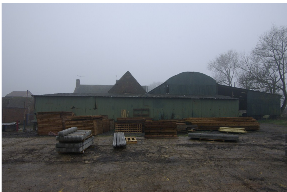
Figure 30 Metal barn to north-east of brick barn Looking south-west
