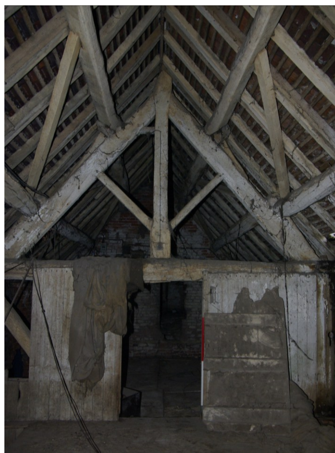
Figure 24 Barn, first floor, north-east room, roof structure Looking south-west. 1m scale
