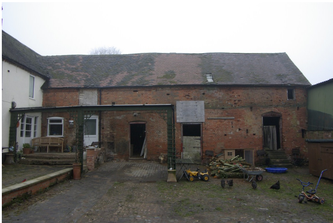
Figure 17 Barn range, south-east facing elevation Looking north-west. 1m scale
