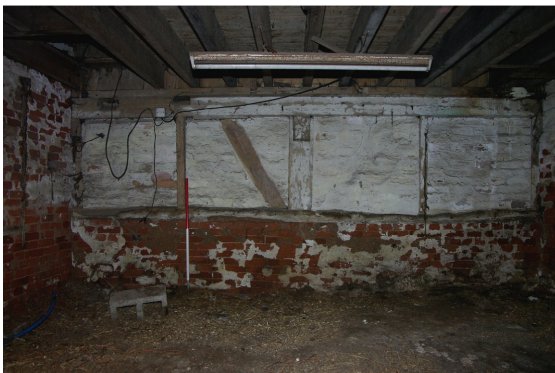
Figure 21 Barn, ground floor, north-east bay Looking south-west. 1m scale
