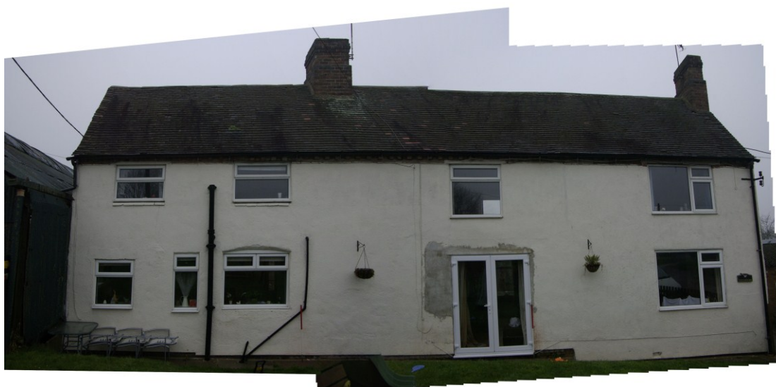
Figure 8 South-west facing elevation of the farmhouse Composite photograph. Looking north-east. 1m scales
