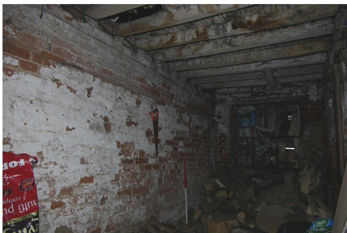
Figure 19 Barn, ground floor, south-west bay Looking north-west
