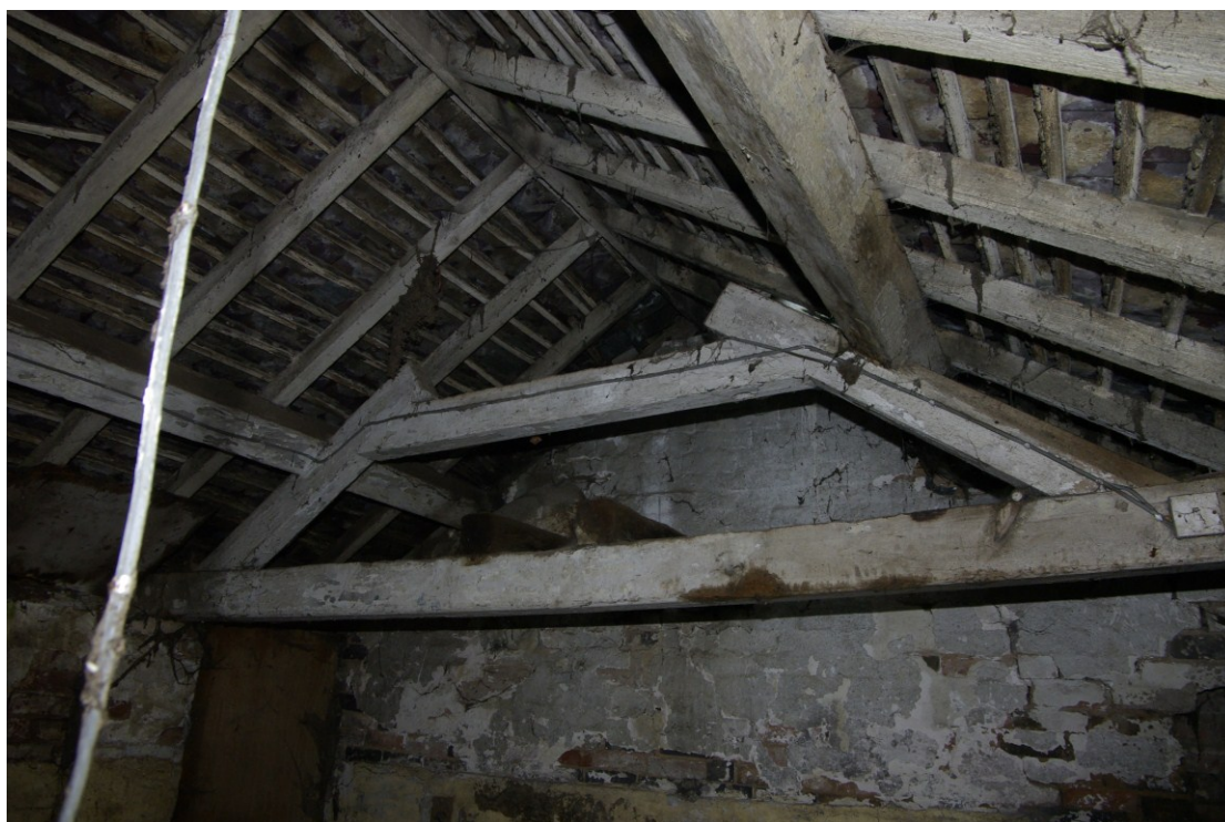
Figure 28 Stable, main roof detail Looking south
