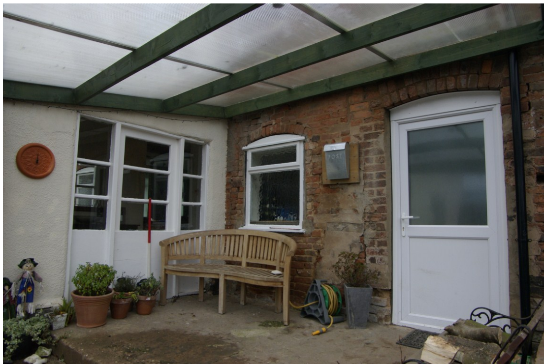
Figure 10 Former doorway in north-east facing elevation Looking west. 1m scale
