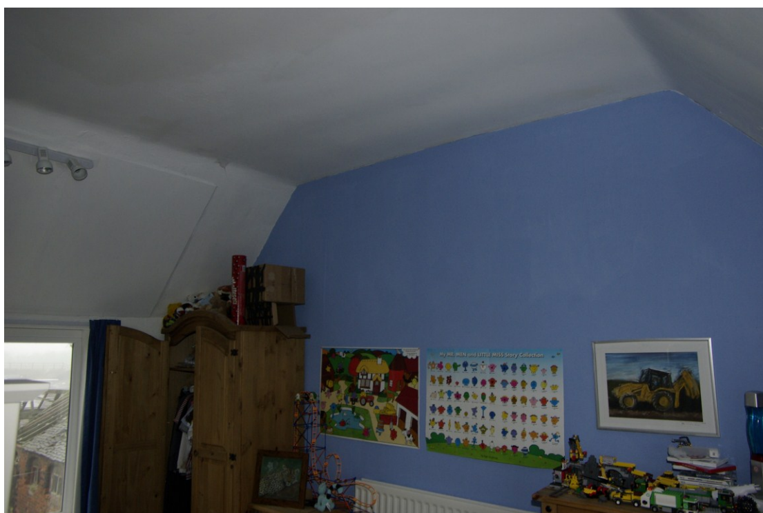
Figure 15 South-eastern bedroom gable end wall Looking east. Note boxed-in chimney breast
