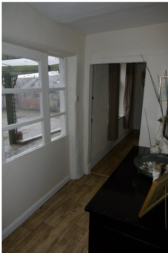
Figure 13 Possible porch area between living room and kitchen Looking east
