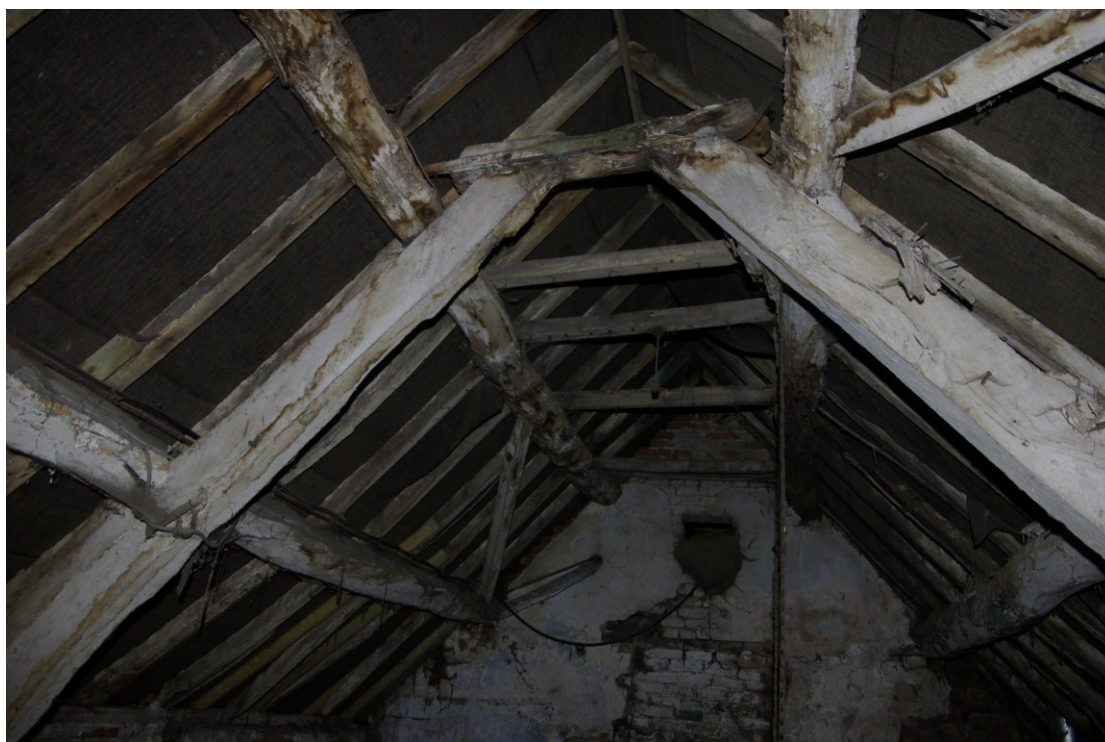
Figure 23 Barn, first floor, south-west room roof detail Looking south-west
