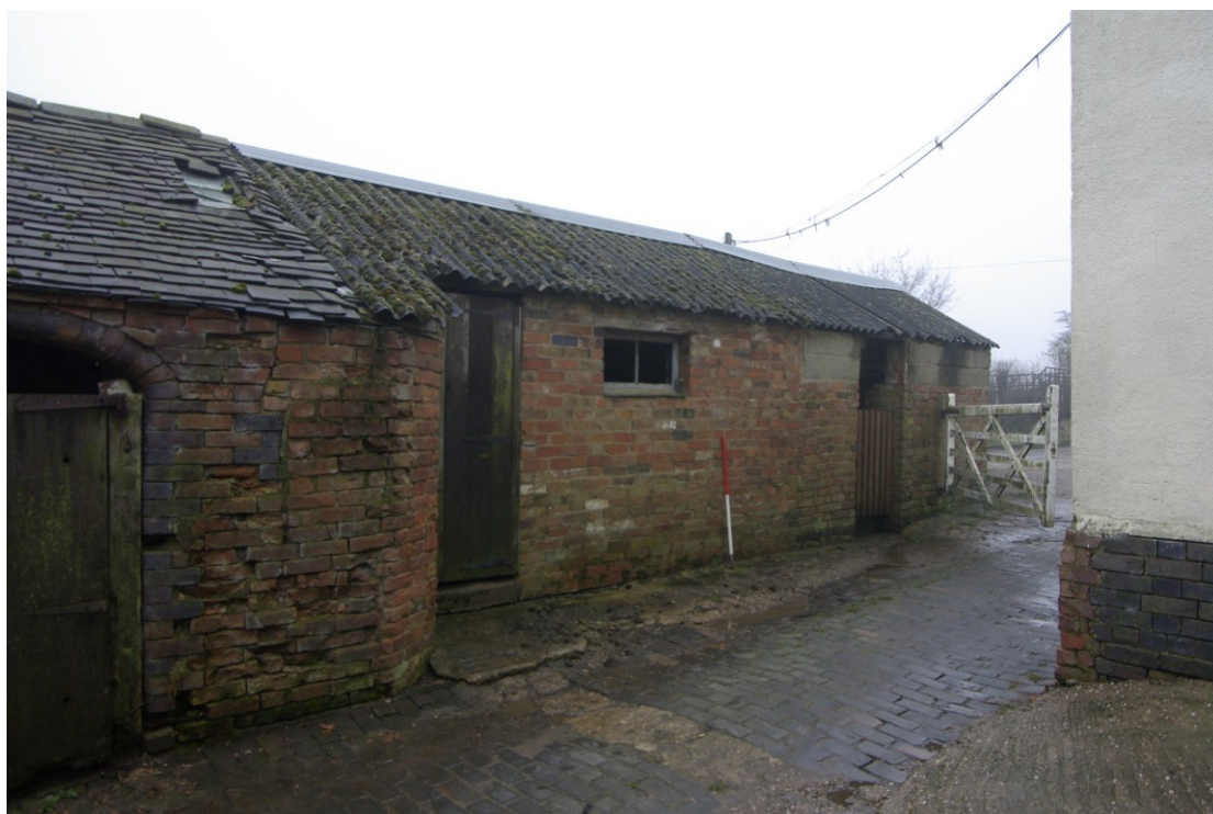
Figure 26 Stables, north-west facing elevation, south-east extension Looking south. 1m scale
