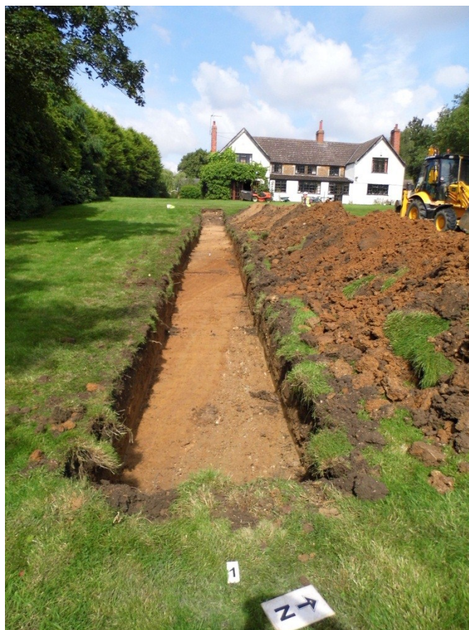
Figure 4: Trench 1: view looking north-west; 1m scale
