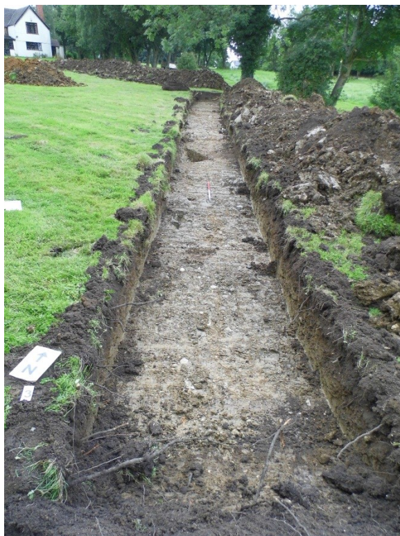
Figure 6: Trench 3: view looking north; 1m scale
