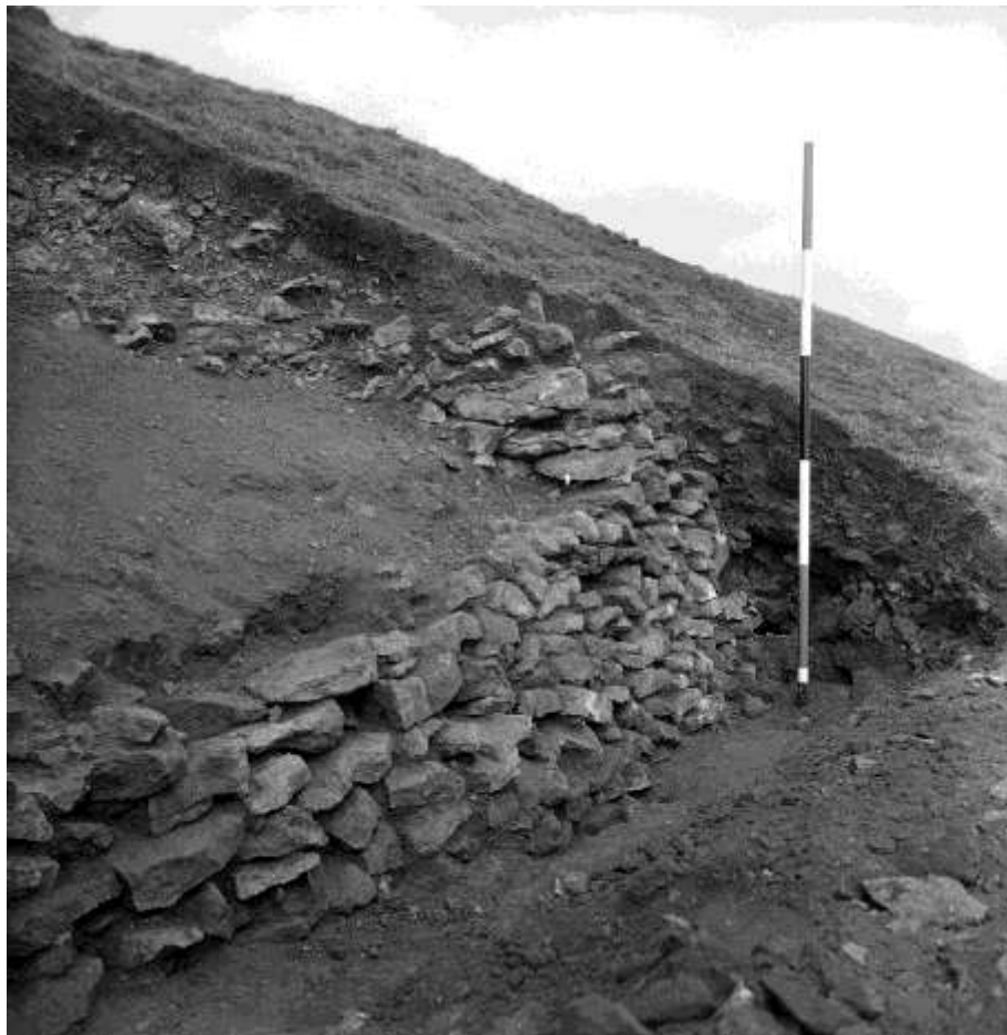
Figure 2. Excavation of the eastern rampart in 1960. revealing the drystone outer face of the rampart and dumped core materials behind.
