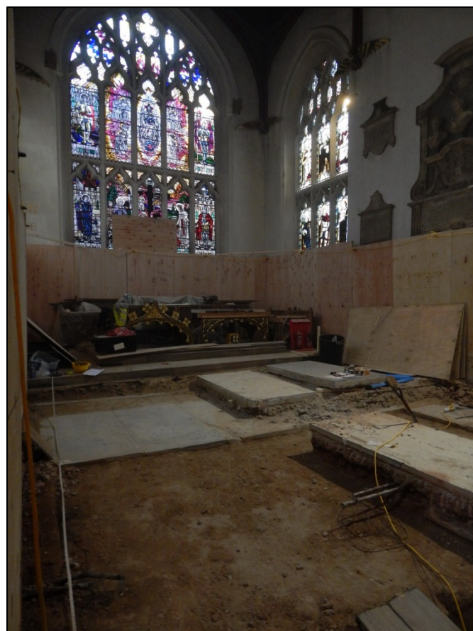
Plate 2 Removal of ledger stones
