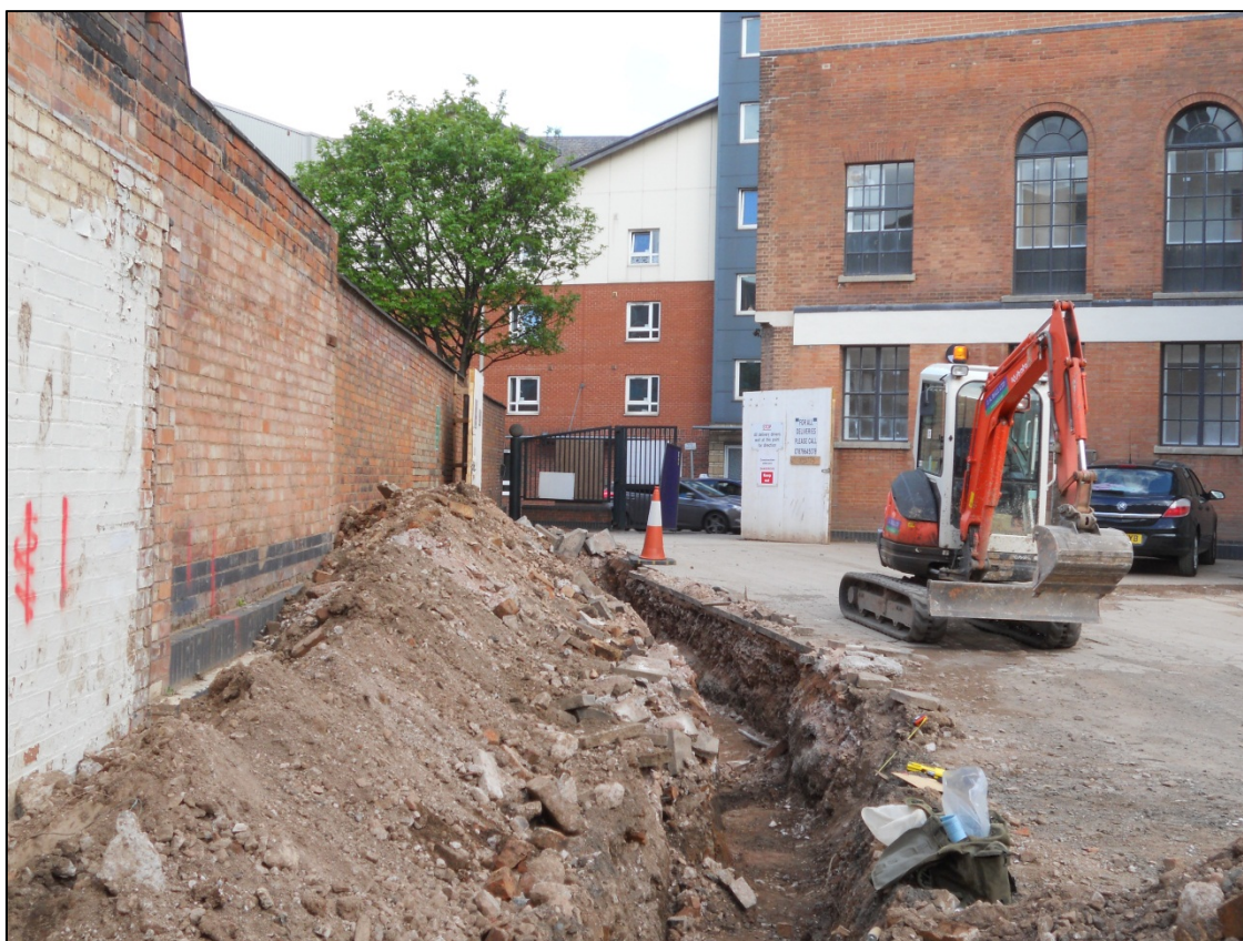
Figure 6: Area 1 service trench, looking north.
