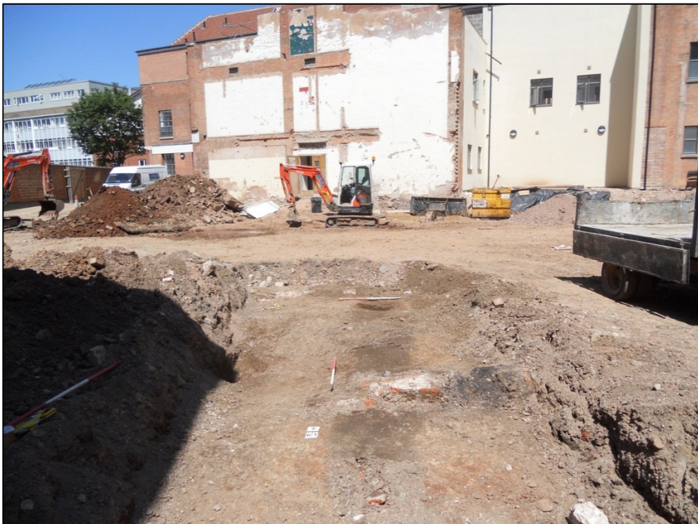
Figure 25: Area 3, Roman ditch [62], looking north.
