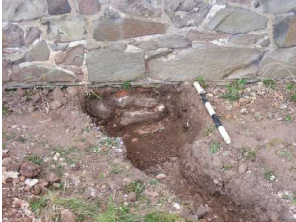
Figure 3: The western wall of the north aisle showing foundations
