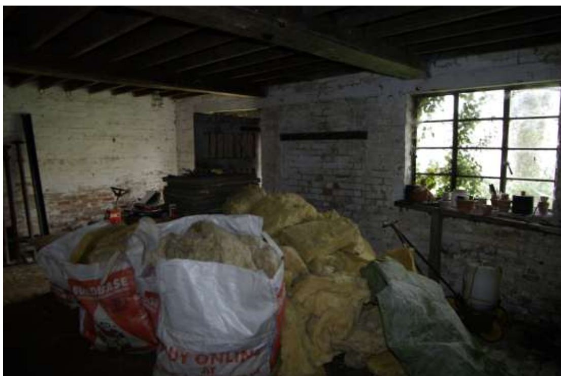
Figure 17 Ground floor, south room Looking south west
