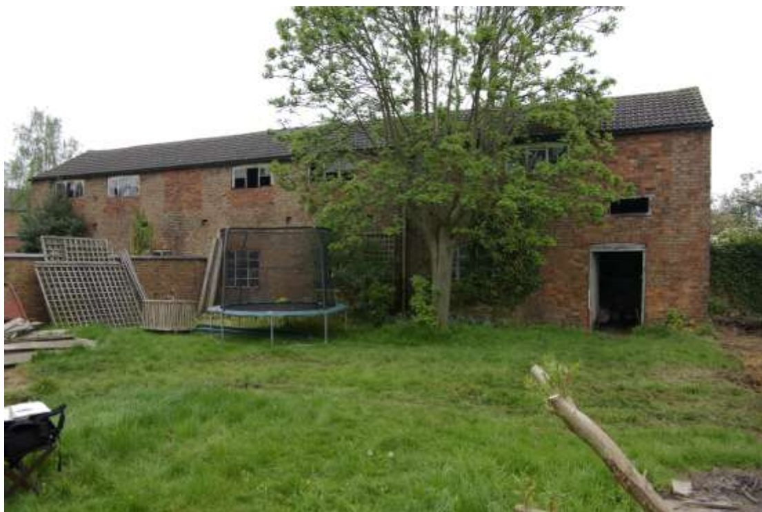
Figure 10 Building 2 West facing elevation Looking east
