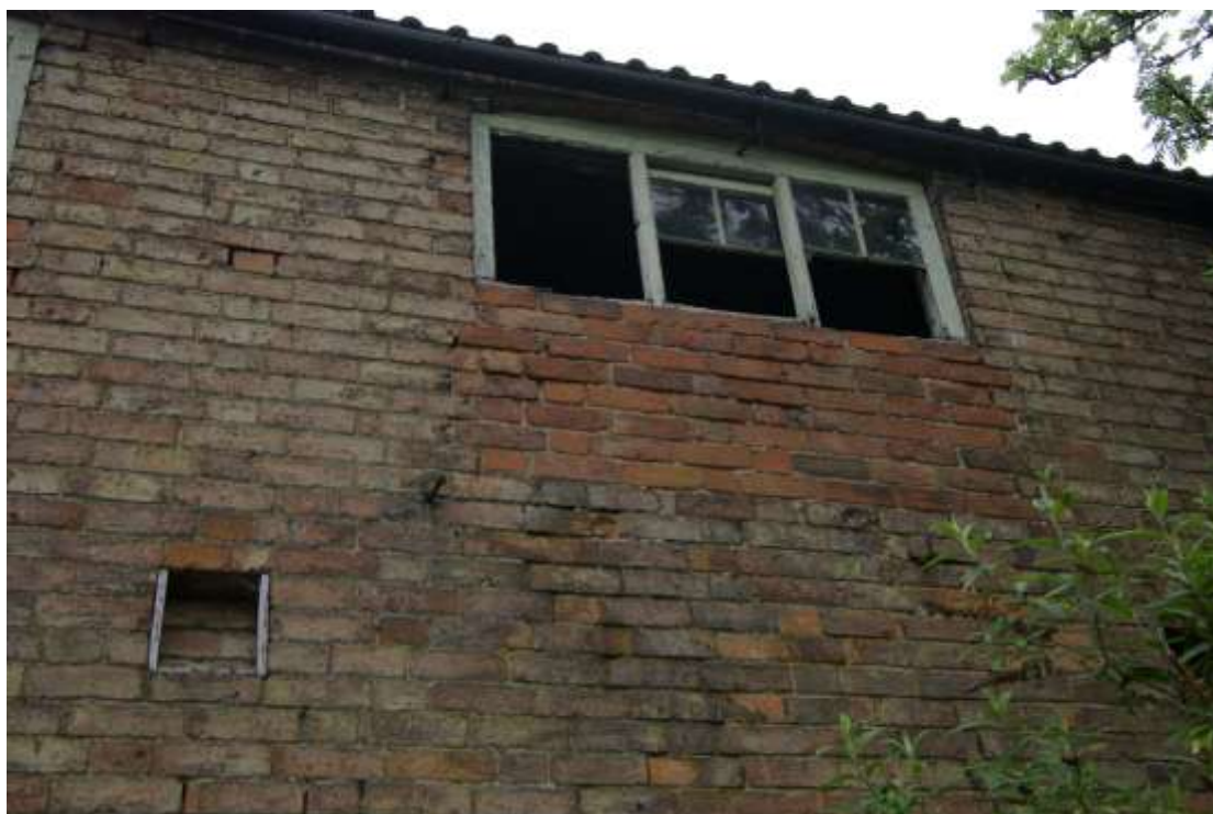
Figure 14 First floor window, west facing elevation
