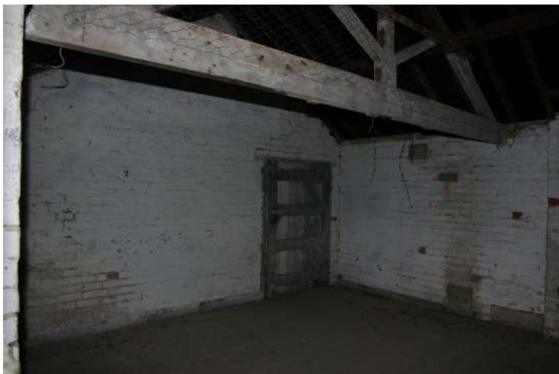
Figure 22 First floor, south room Looking north west
