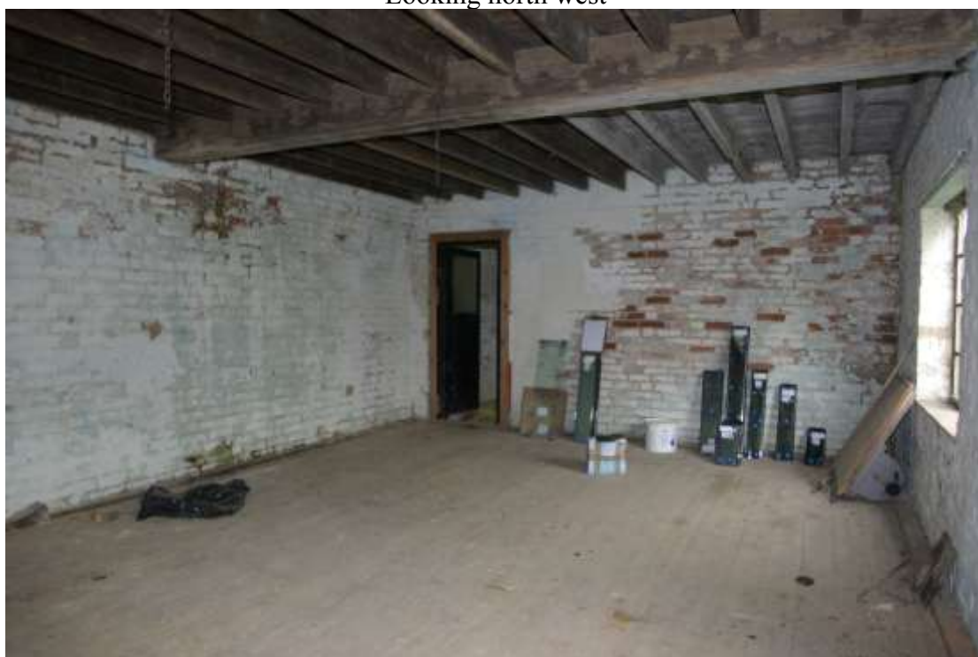
Figure 21 Ground floor, central room Looking south east
