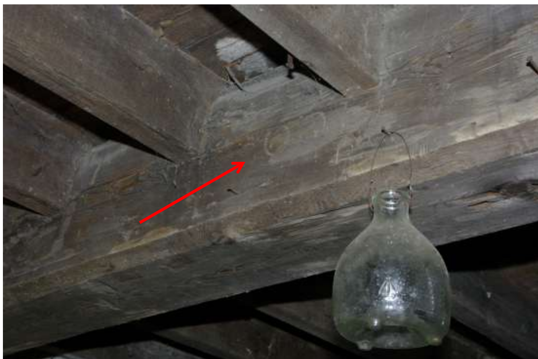
Figure 19 Ground floor, south room Possible spectacle marks (arrowed)
