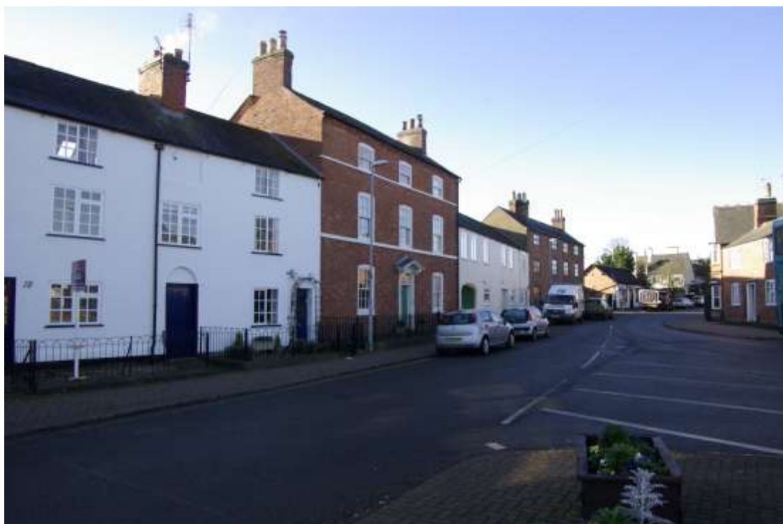
Figure 3 22 High Street Looking south west. Site entrance is under the archway between the two cars
