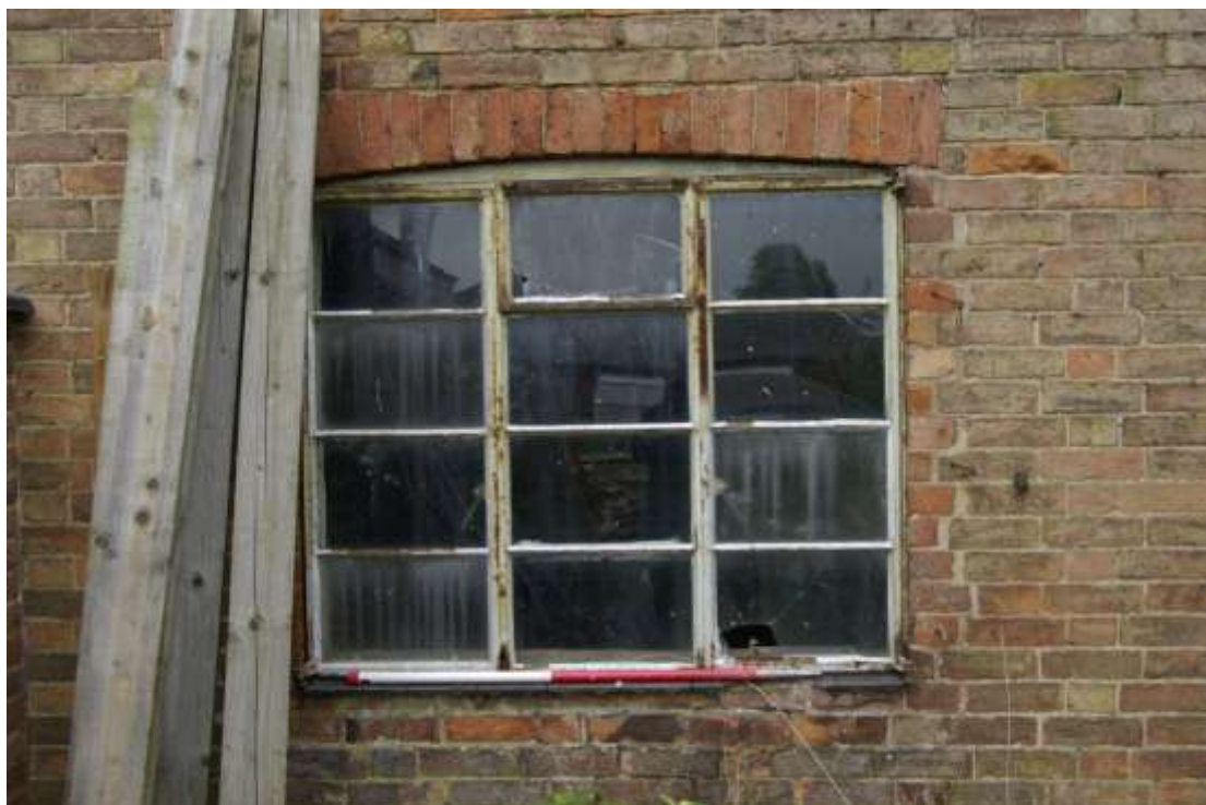
Figure 12 Ground floor window, west facing elevation Looking east. 1m scale
