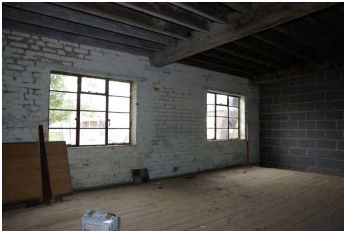
Figure 20 Ground floor, central room Looking north west
