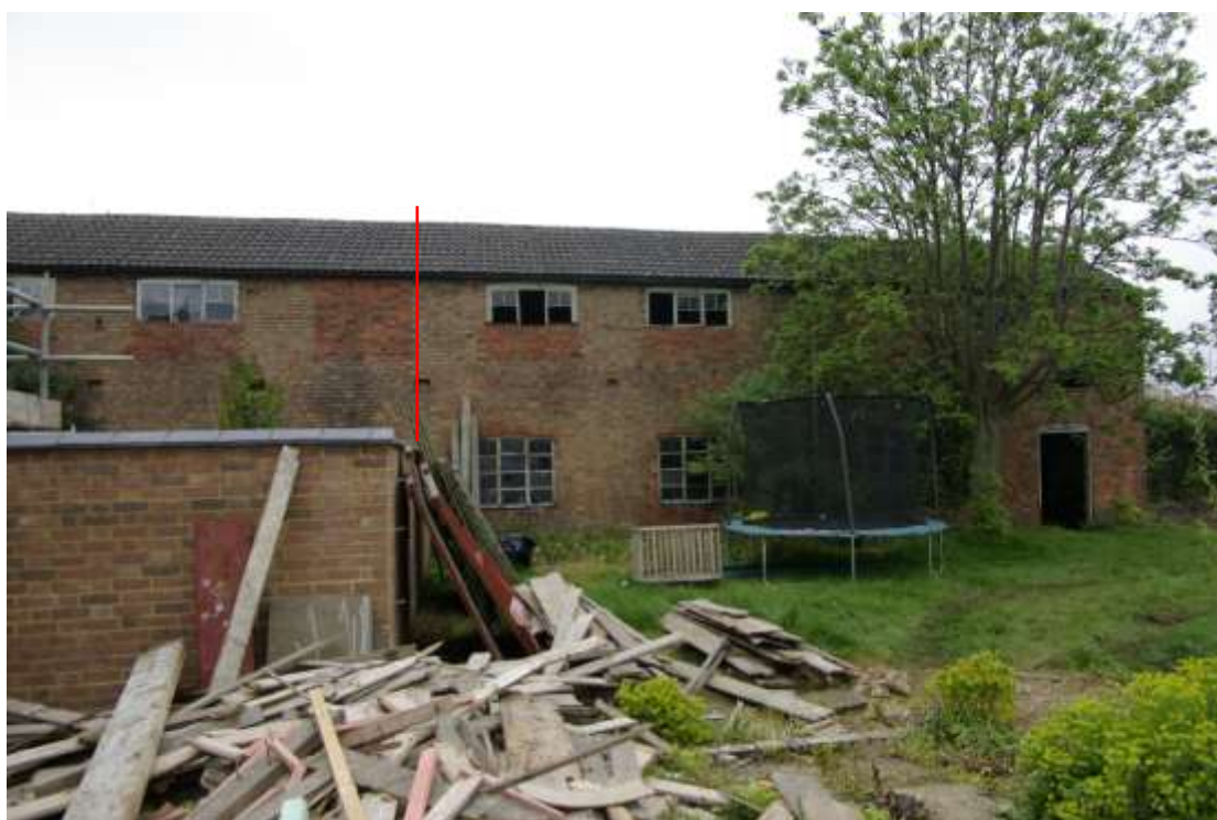
Figure 11 Building 2 West facing elevation Red line indicates dividing line between the two properties
