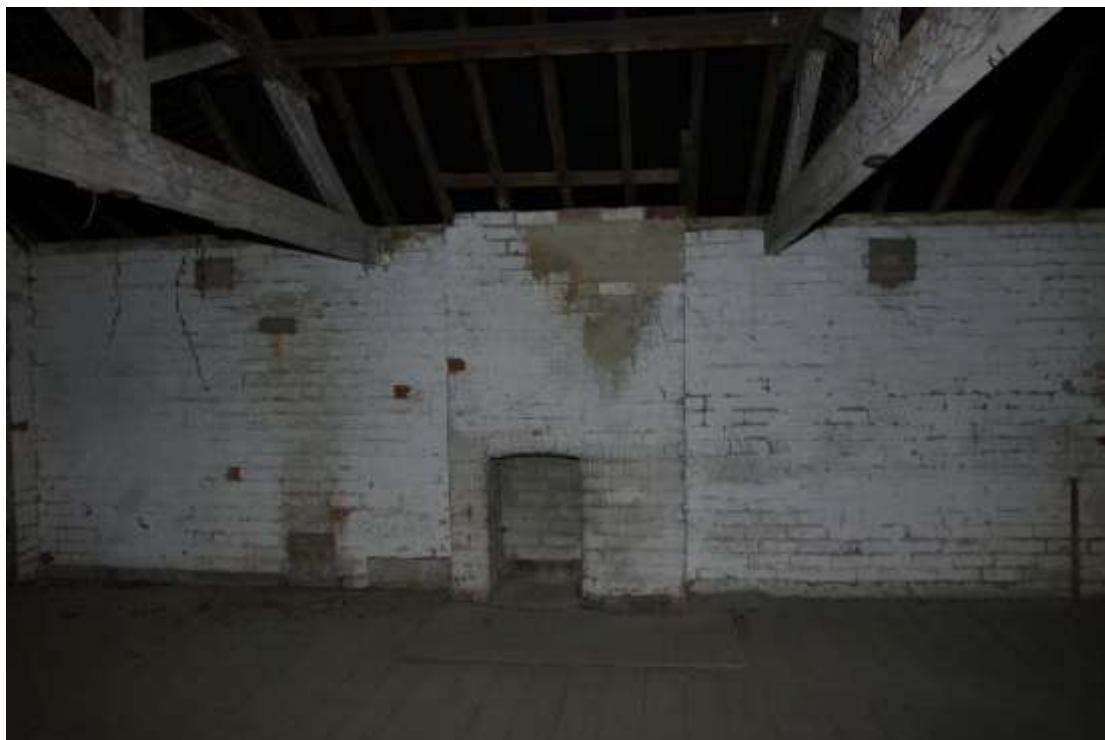
Figure 23 First floor, south room looking east
