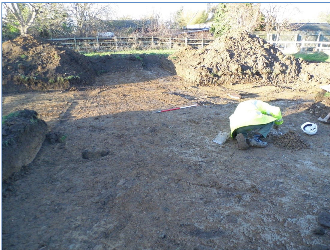
Figure 7 North part of site, looking north
