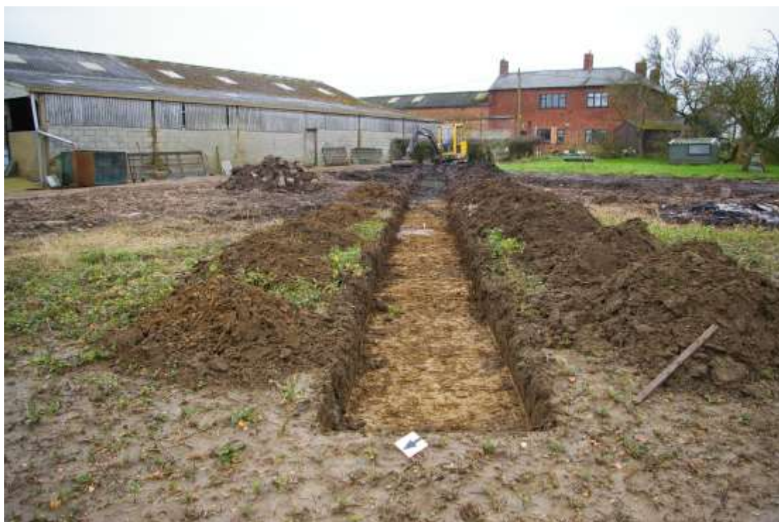
Figure 6 Post excavation photograph of trench Looking south east. 1m scale
