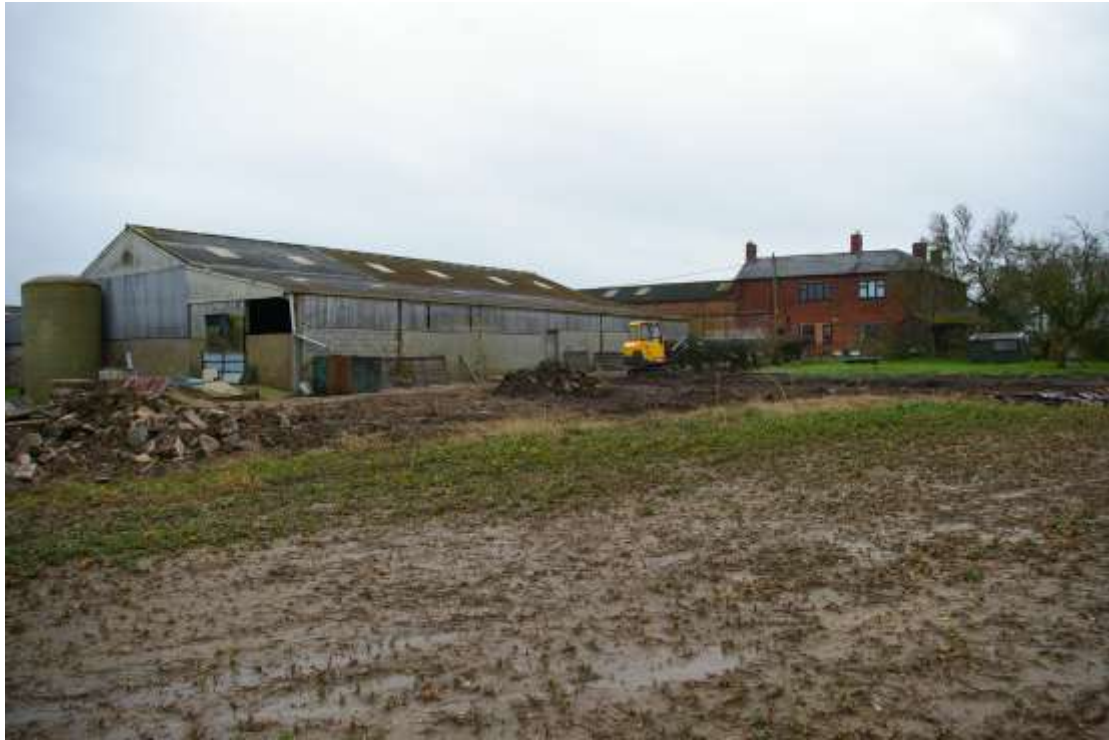
Figure 5 Evaluation area before excavation of trench Looking south east across undisturbed area to location of demolished buildings. Start of trench in immediate foreground
