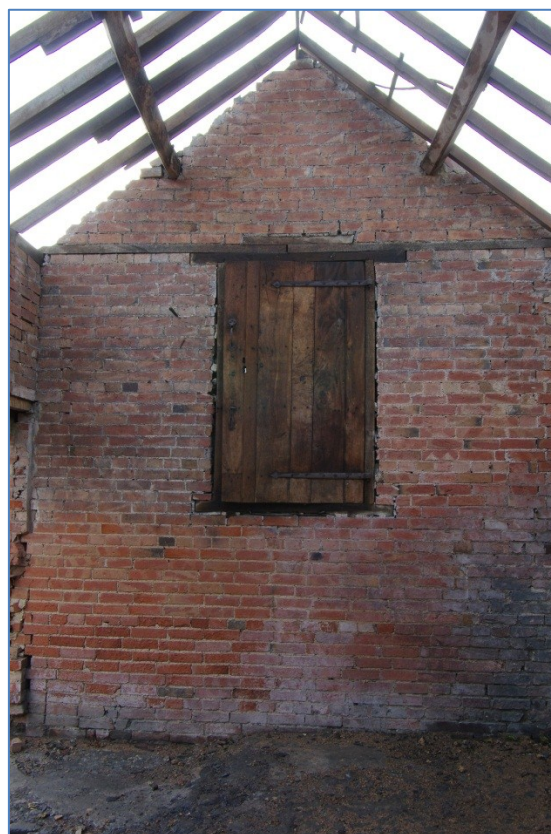
Figure 14 Barn B, garage 2, looking south to garage 1
