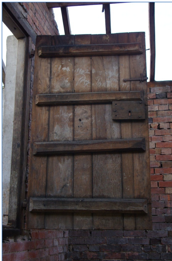
Figure 15 Barn B, garage 2, looking west
