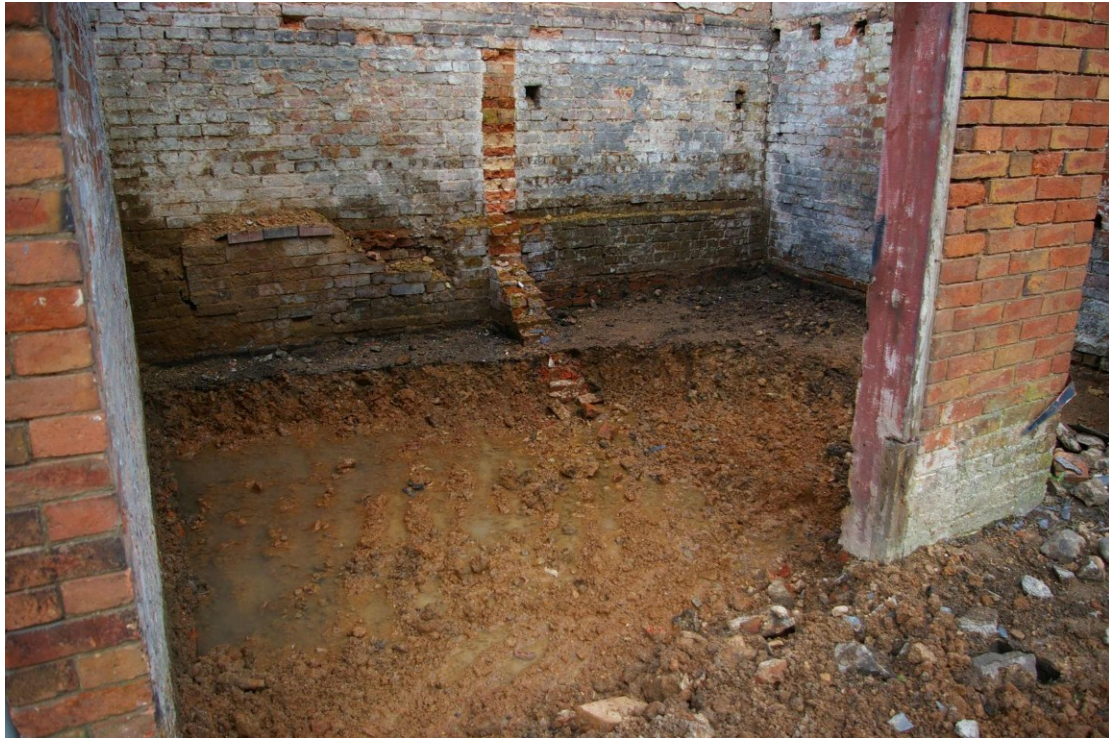
Figure 23 Barn B, Garage 1 partial floor reduction Looking west
