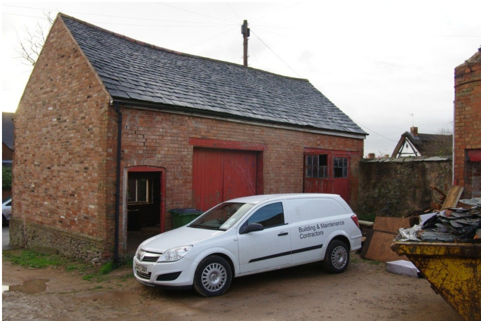
Figure 7 Barn A, looking south
