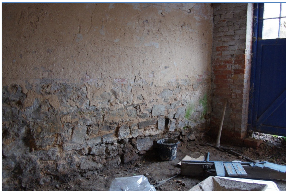
Figure 9 Barn A interior, south west bay, looking west
