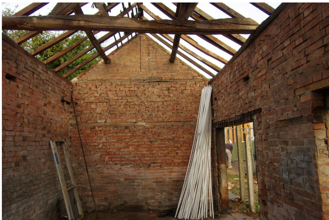
Figure 16 Barn B, garage 2, looking north to garage 3
