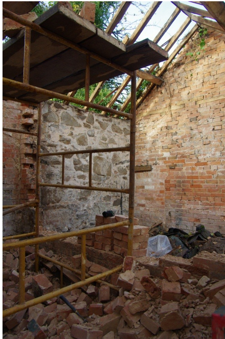
Figure 17 Barn B, garages 4-5, looking north west
