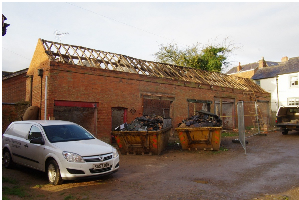
Figure 11 Barn B, looking west
