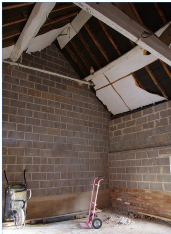
Figure 8 Barn A interior, NE bay, looking east
