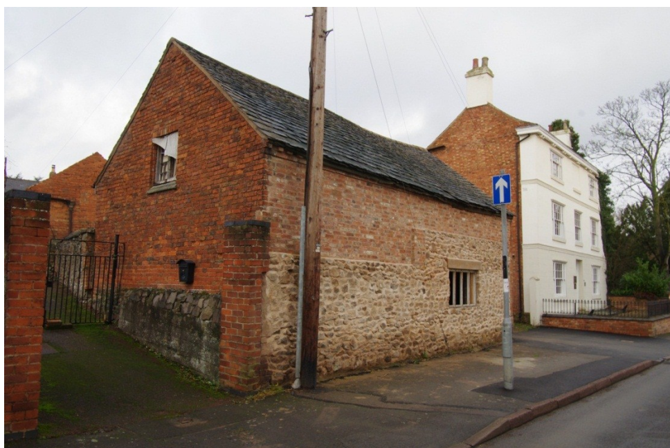
Figure 5 Barn A and 'The Cedars', looking north
