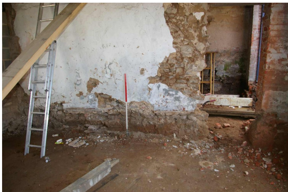
Figure 25 Reduced floor level and knocked-through doorway Looking west. 1m scale
