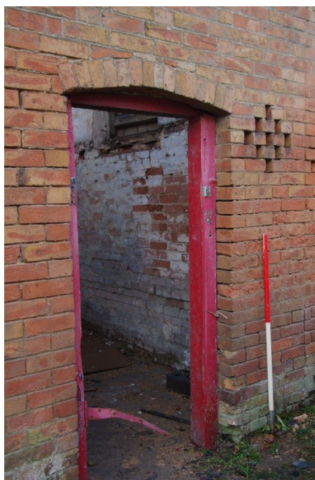
Figure 13 Barn B, detail of garage 1 door and vents, looking west
