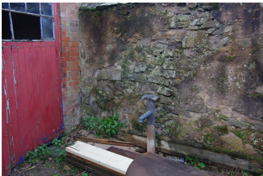
Figure 10 Pump in yard adjacent to Barn A
