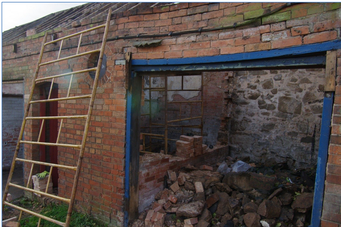
Figure 18 Barn B, garages 4-5, looking south west
