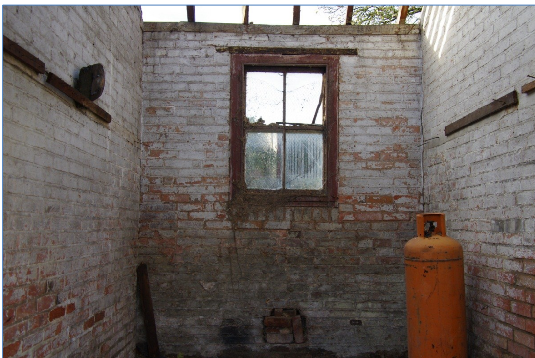
Figure 19 Barn B, garage 3, looking west
