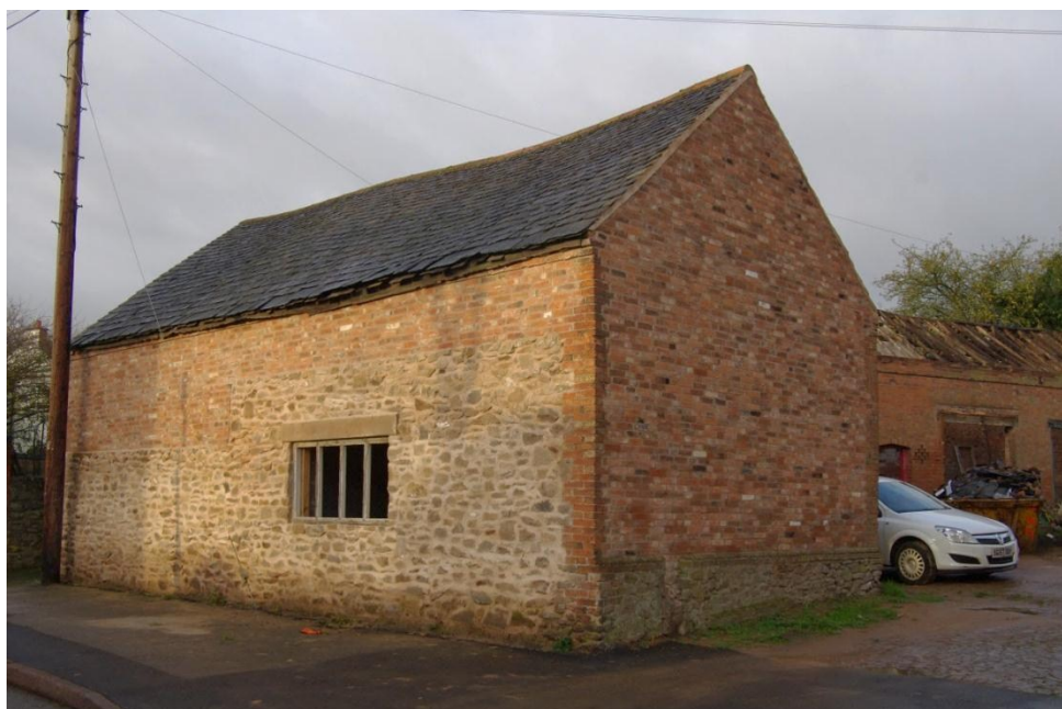
Figure 4 Barn A, looking west
