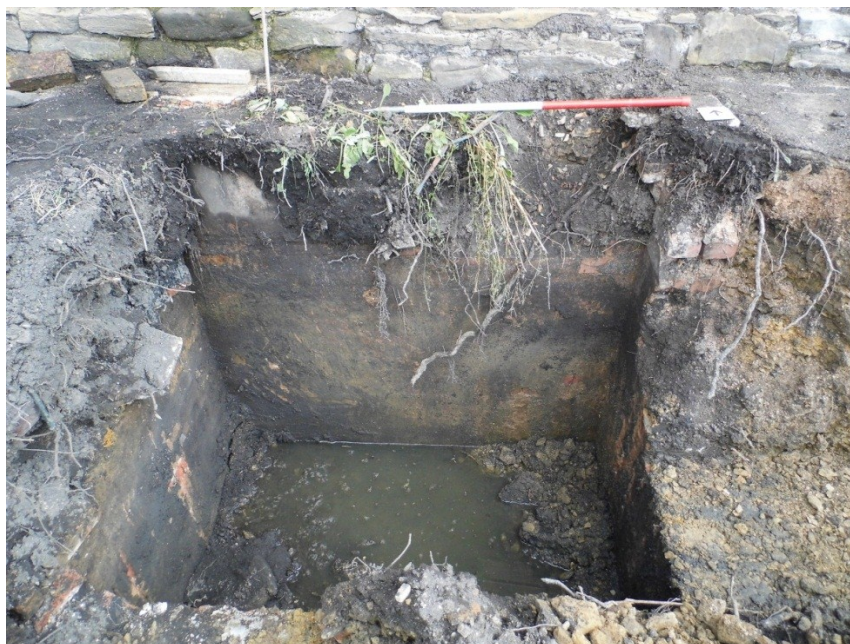
Figure 8: Brick lined sump/tank, looking north
