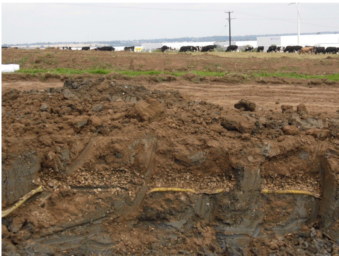
Figure 10. Trench in Area 5 showing made up ground.
