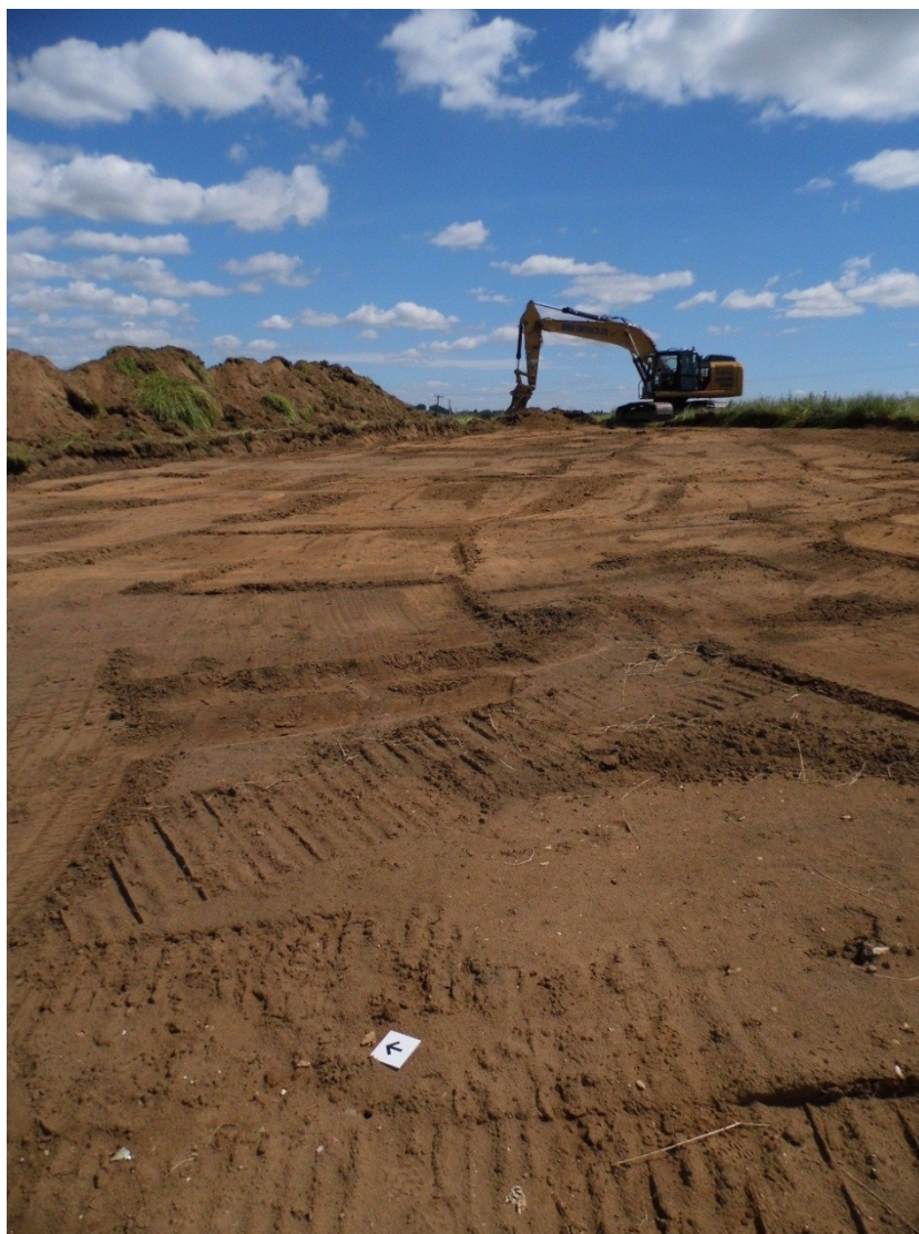
Figure 10. Area 4, Stripped area of Turbine 1.
