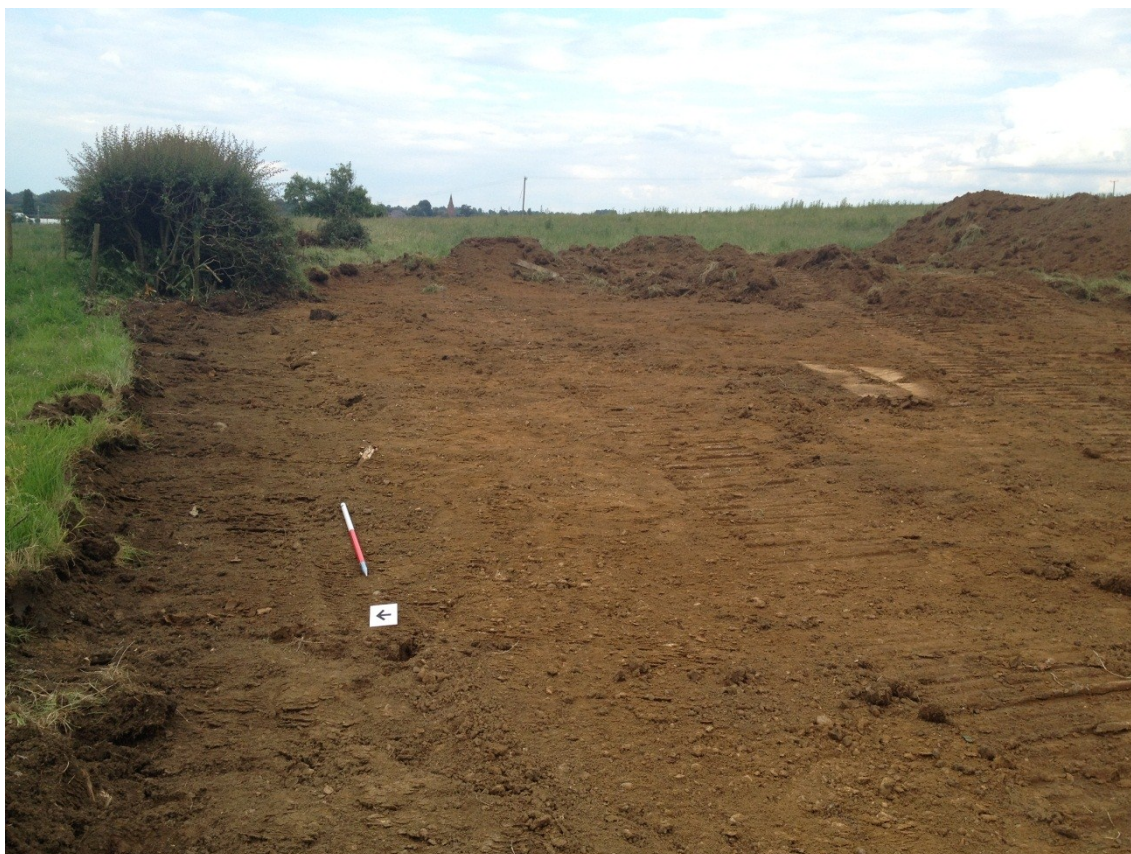
Figure 9. Area 3, Stripped area of the substation.
