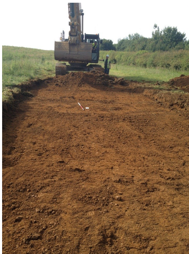
Figure 7. Area 2, Topsoil stripped onto natural subsoil.
