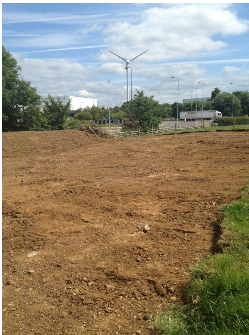
Figure 6. Area 1, Disturbed made-ground.
