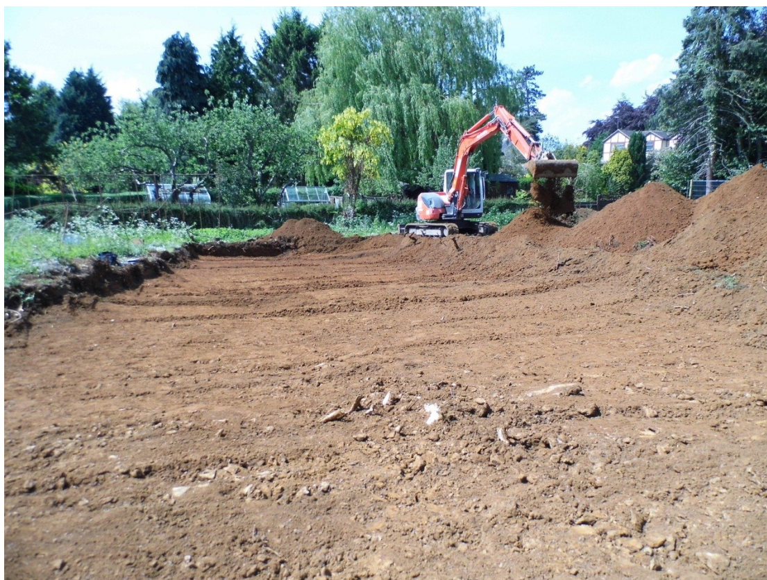
Figure 5. Excavation area, looking west.
