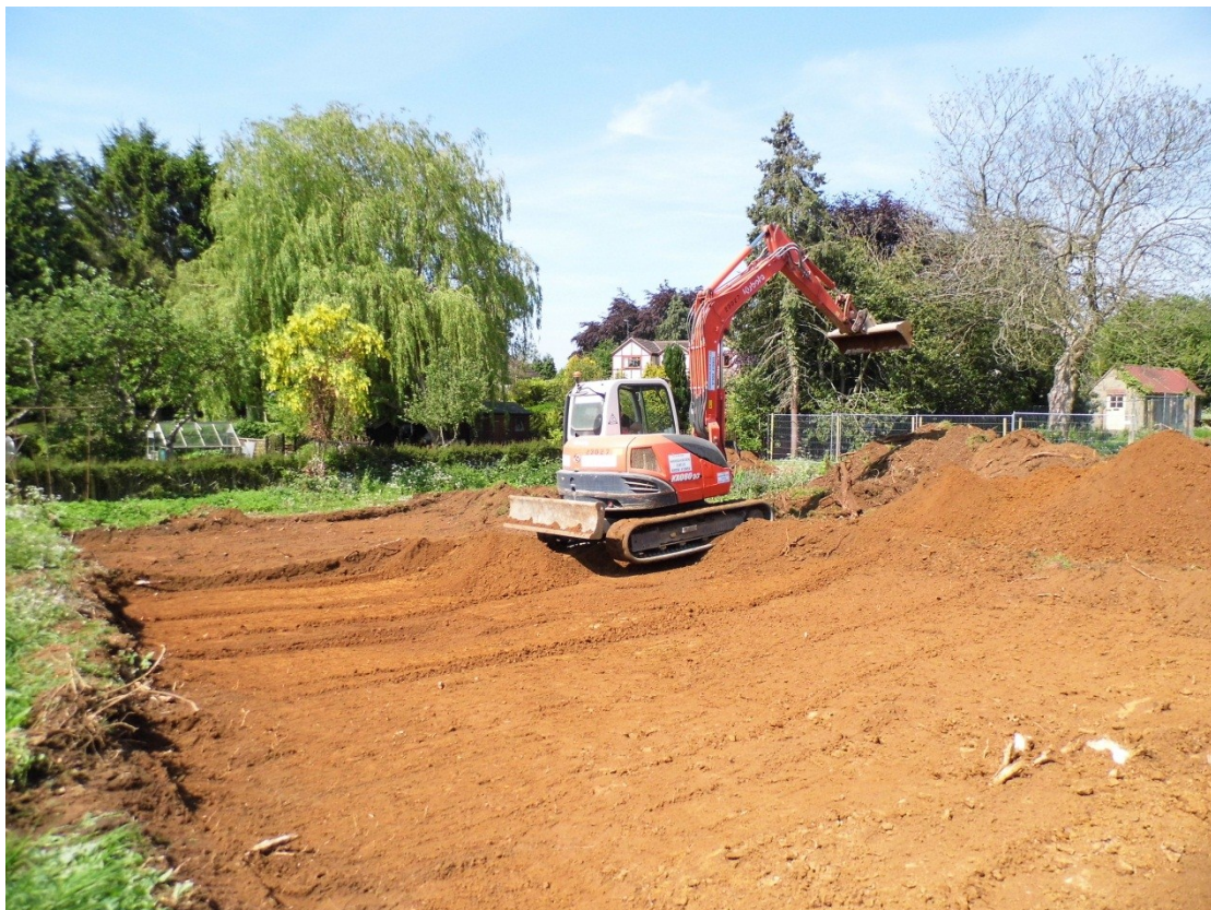
Figure 4. Excavation area, looking north-west.
