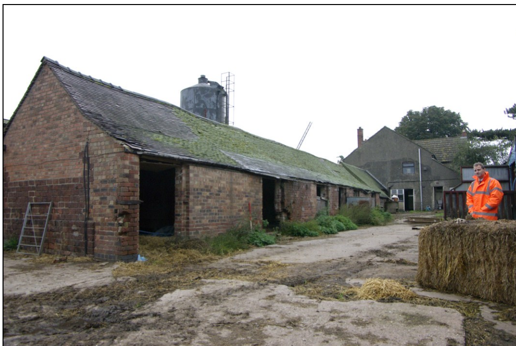
Figure 17. Loose-boxes with rebuilt frontage, looking north.
