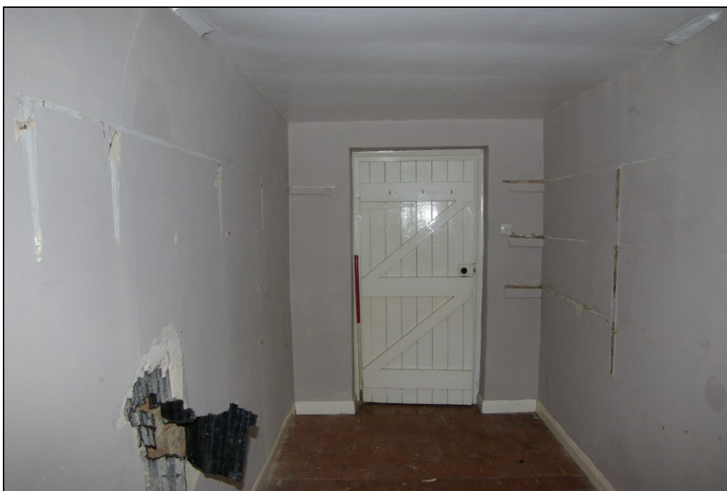
Figure 30. Pantry, with ledged and braced timber matchboard door, looking north-west.
