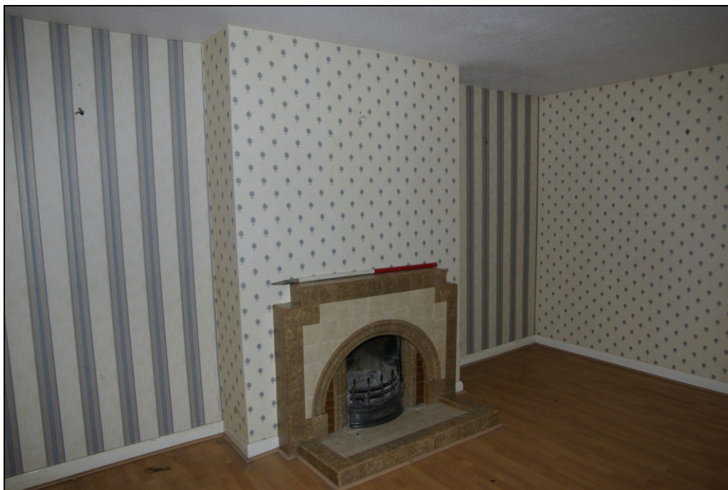
Figure 31. 1930s fireplace in parlour. Looking south.
