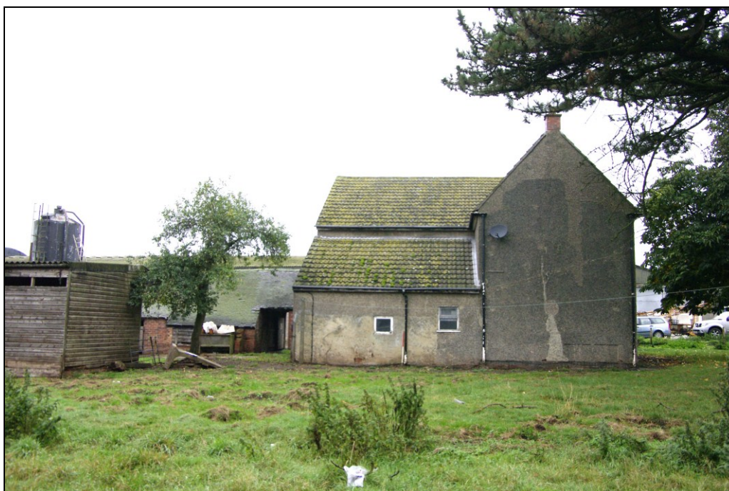
Figure 23. South-east facing elevation of house, looking north-west.
