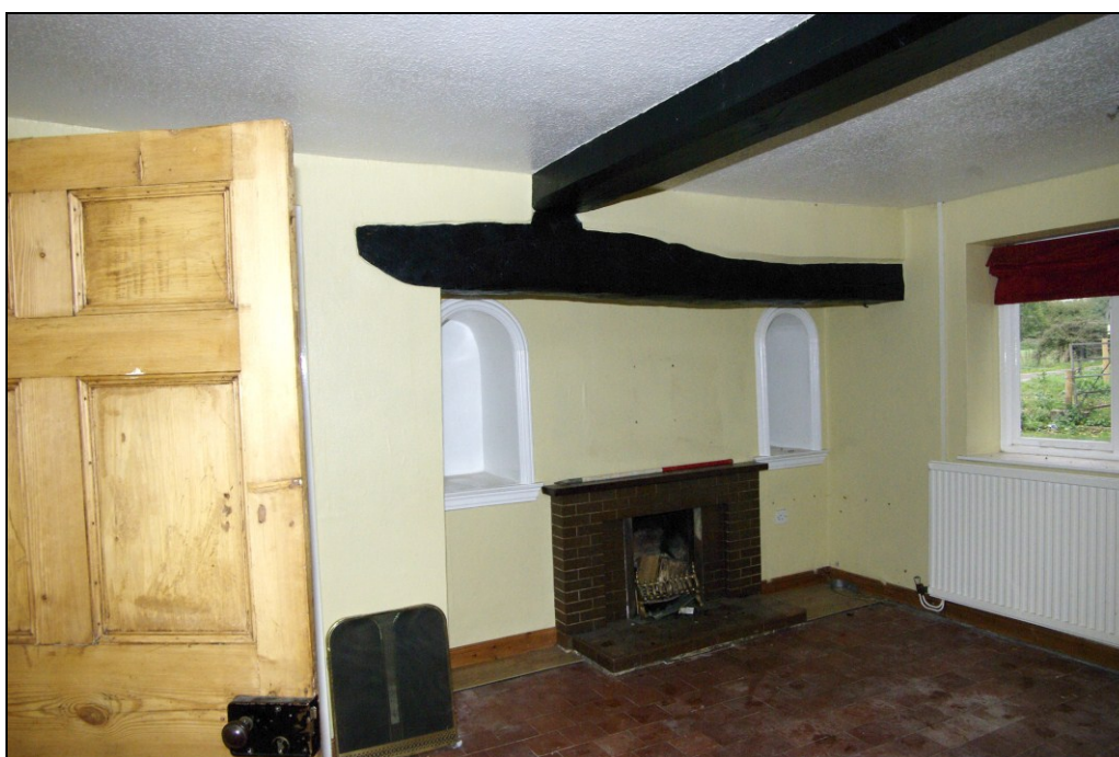
Figure 28. Original sitting kitchen, with chamfered and stopped axial beam and timber bressummer beam. Looking north.
