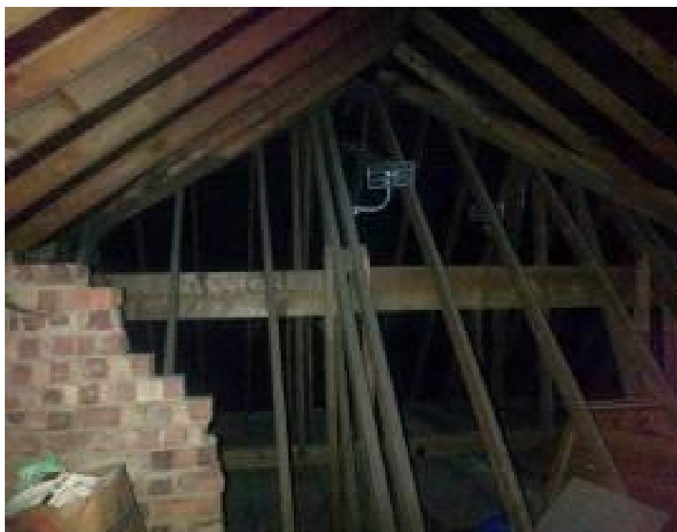
Figure 44. Modern roof structure over farmhouse, looking north-west.
