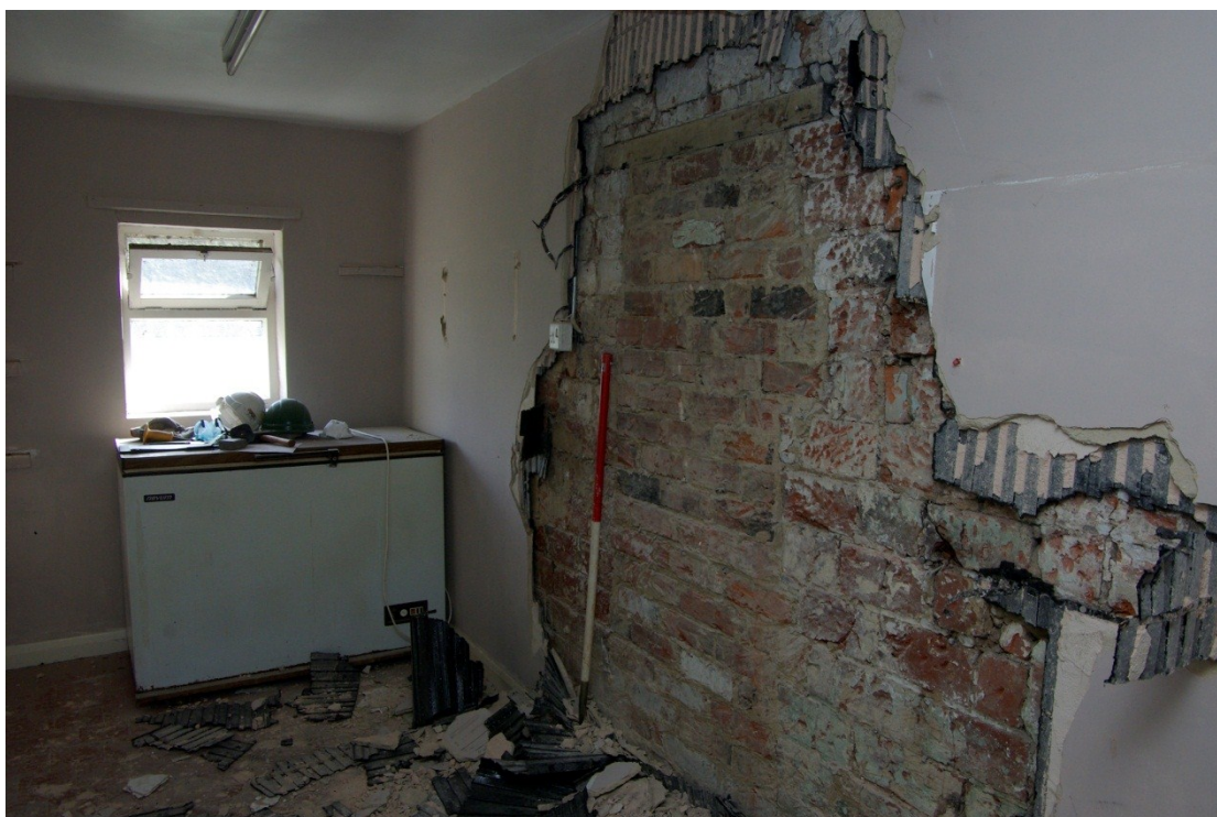
Figure 39. Blocked doorway between pantry and larder, looking south-east.
