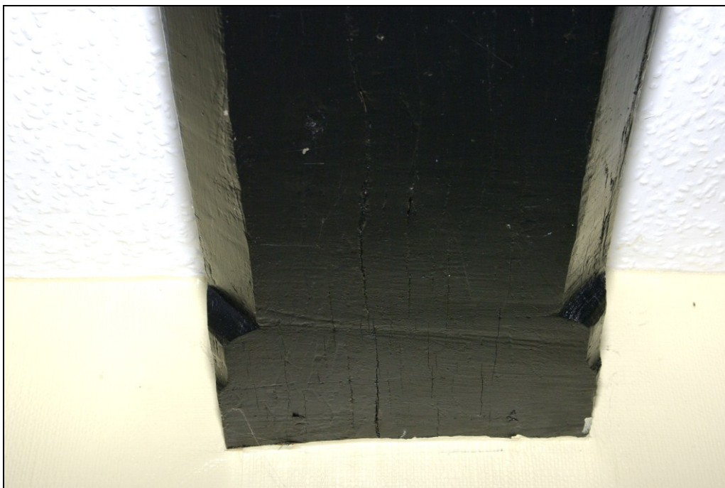
Figure 29. Detail of chamfered and stopped axial beam. Looking south-east.
