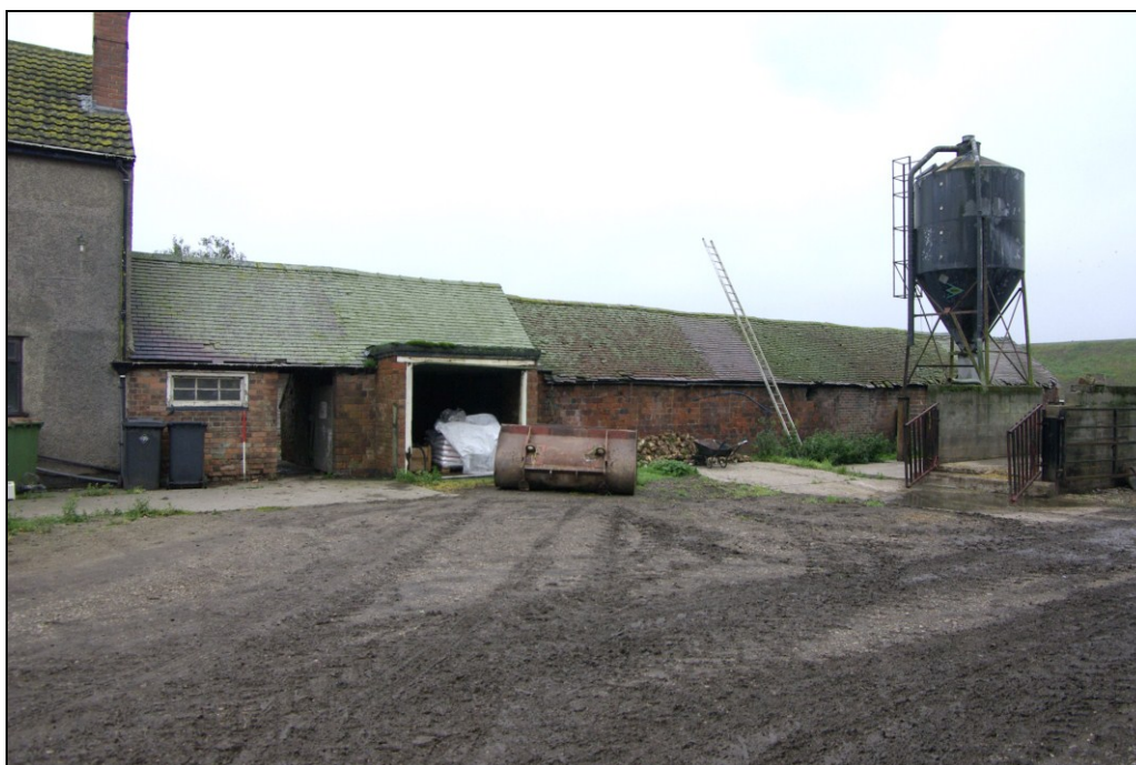
Figure 12. Outbuildings and rear of loose-boxes. Looking south.
