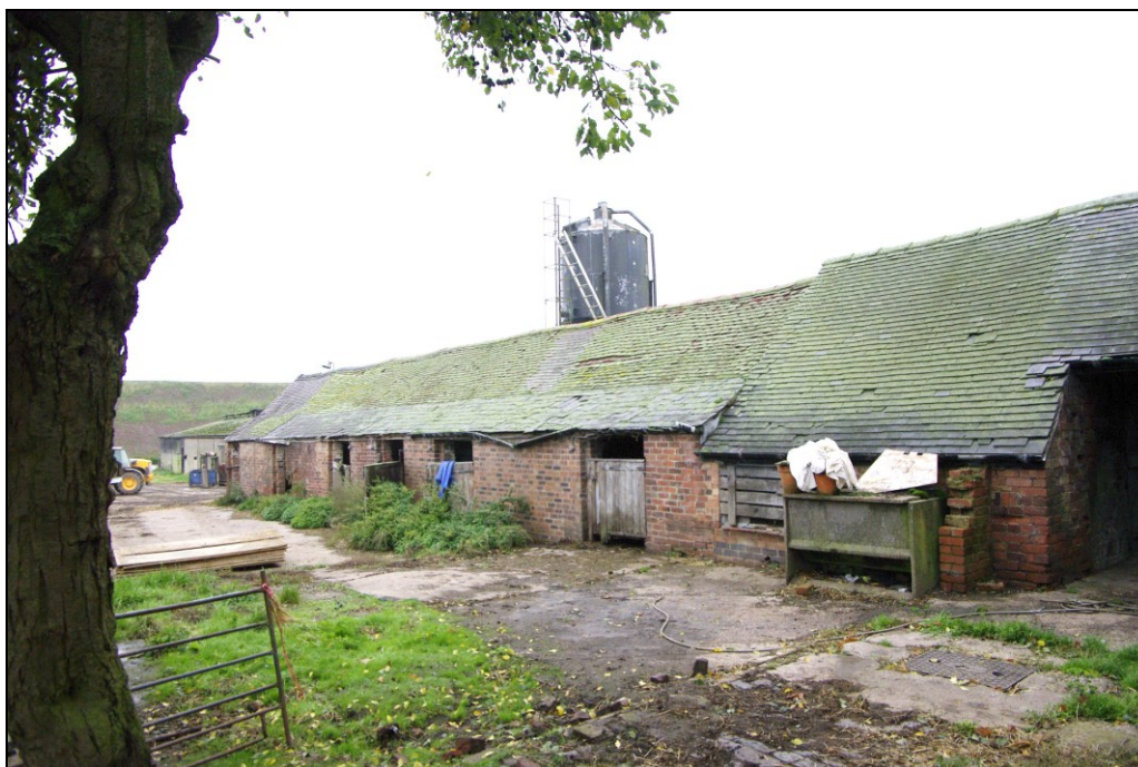
Figure 19. Loose-boxes looking south-west.
