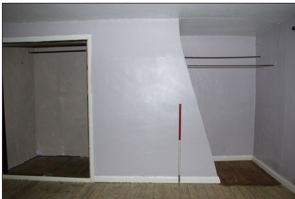
Figure 34. Chimney stack in first floor bedroom, looking north-west. One metre scale
