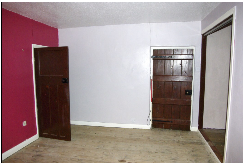
Figure 35. Timber plank and batten door to rear bedroom, with 1930s panelled door to landing on left-hand side, looking south-west.
