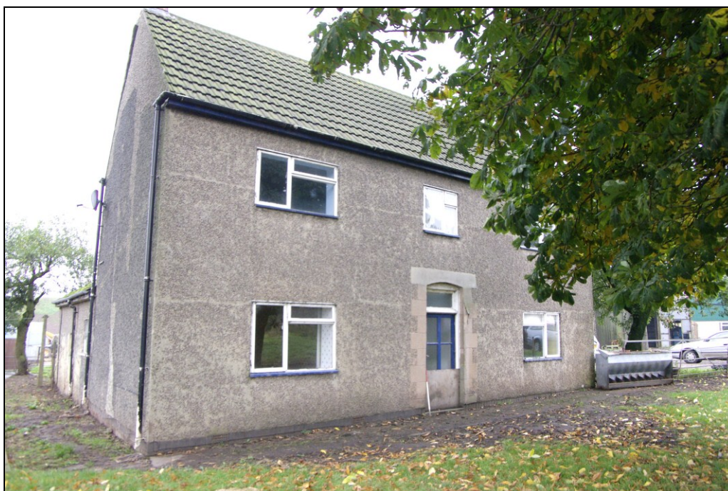
Figure 24. Principal, north-east facing elevation of house, looking west.
