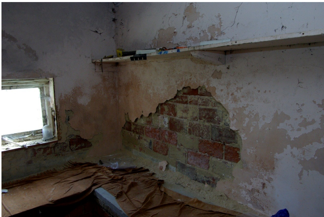
Figure 41. Jumb bricks to external wall of larder, looking south-west.
