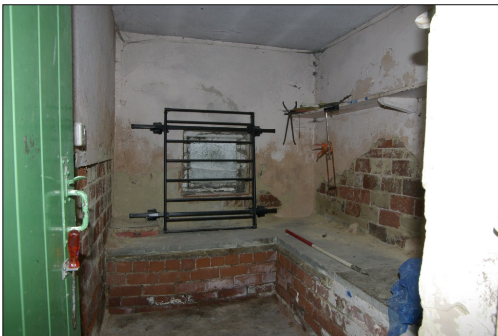
Figure 26. Larder, with brick and concrete slab thrall, looking south-east.
