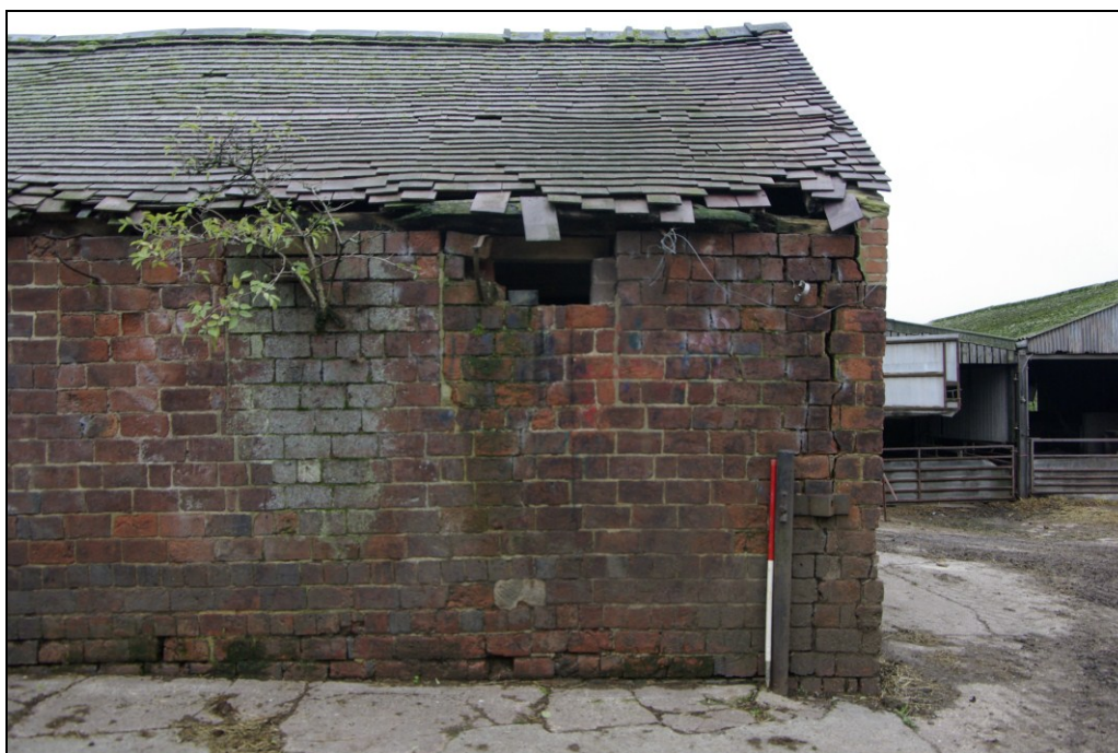
Figure 14. Detail of rear of loose-boxes, constructed with 'jumb' bricks, looking south-west.
