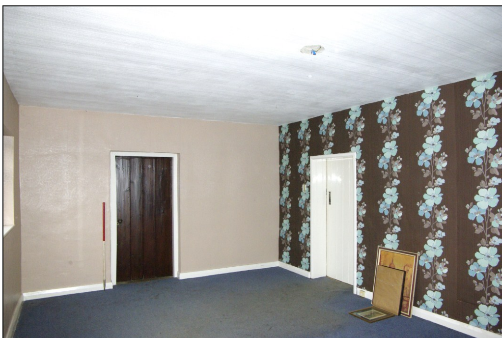
Figure 36. Pair of plank and batten doors in rear bedroom, looking north-east.
