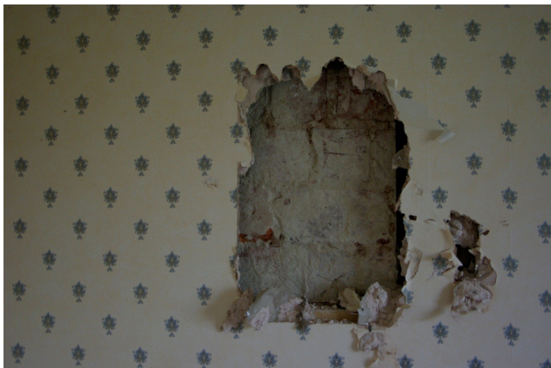
Figure 43. Jumb bricks to front room, looking north-west.
