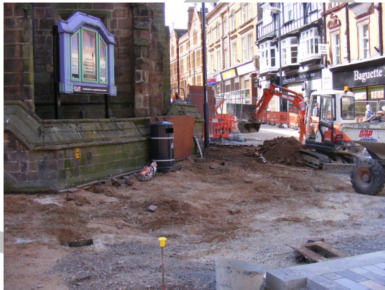
Figure 4: View across northern part of excavated area, looking north-west
