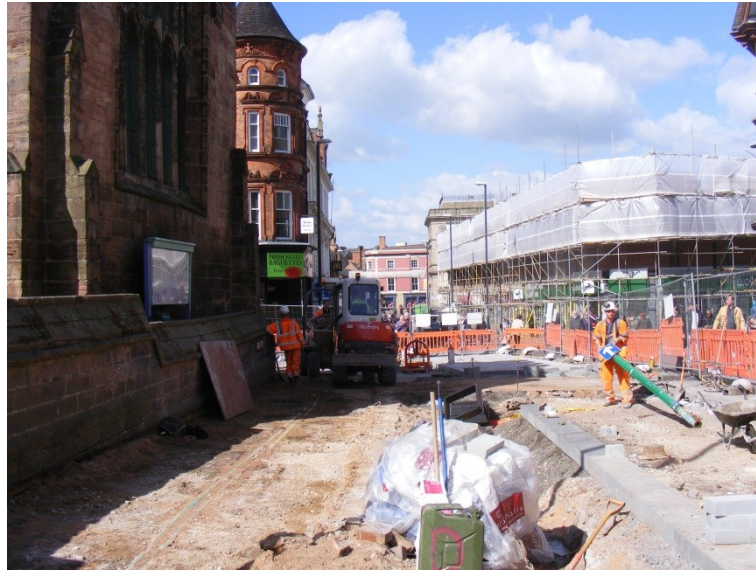
Figure 3: General view across excavated area, looking north
