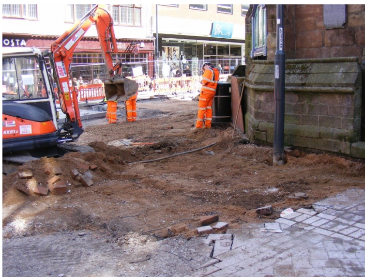
Figure 8: Formation level on the north side of the church
