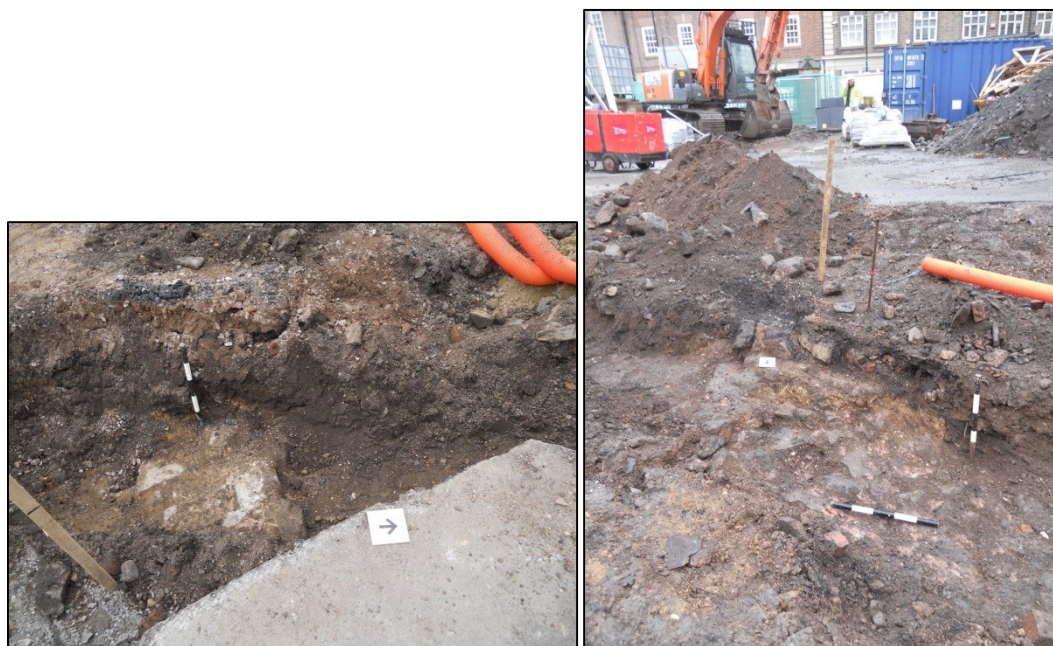
Plate 9 Hospital West Wing Foundations north wall (05)
