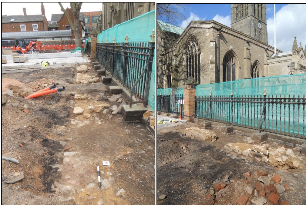
Plate 11 Wyggeston's Hospital east wall foundation Plate 12 Wyggeston's Hospital east wall foundation
