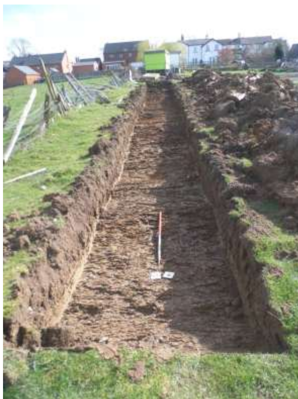
Figure 6: Trench 6; general view looking south (1m scale)
