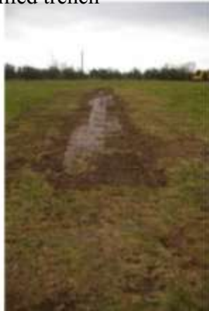
Typical backfilled trench
