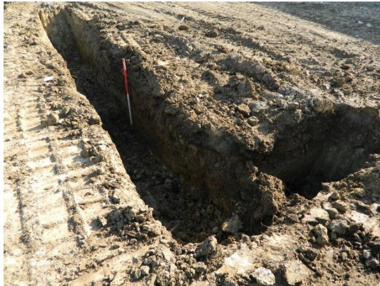
Figure 6 Foundation trench looking north-east 1m scale
