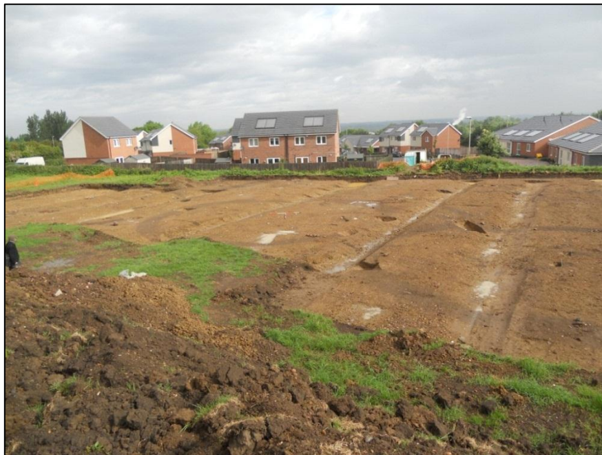
Plate 2: View of central stripped area looking north illustrating the corrugated effect from removing the furrows and showing ring gullies of Enclosure B (right) and Roundhouse 4
