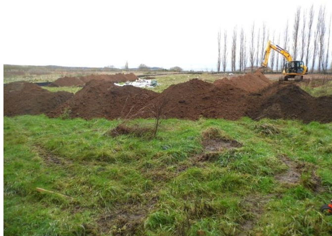
Plate 1: Work in progress on trench 3
