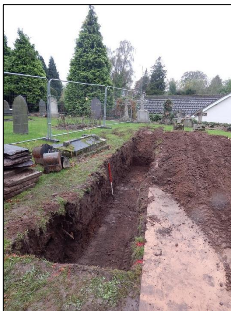
Figure 6: Drainage trench looking west
