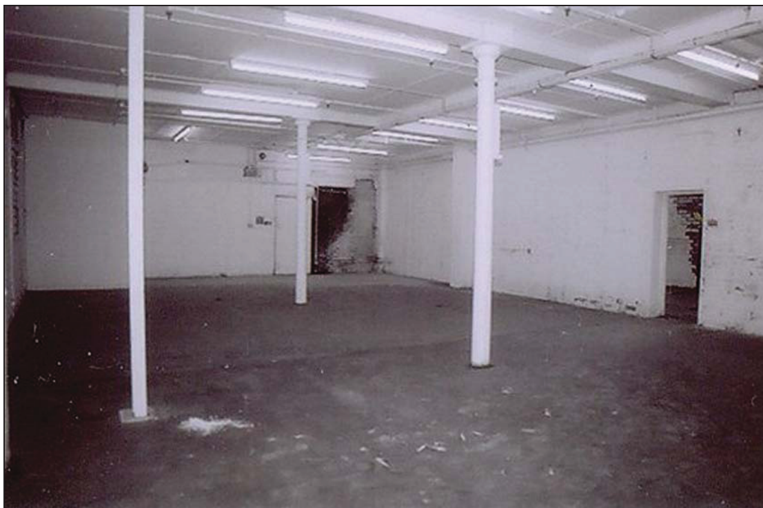
Plate 15 25 Bede Street, ground floor. Looking southwest
