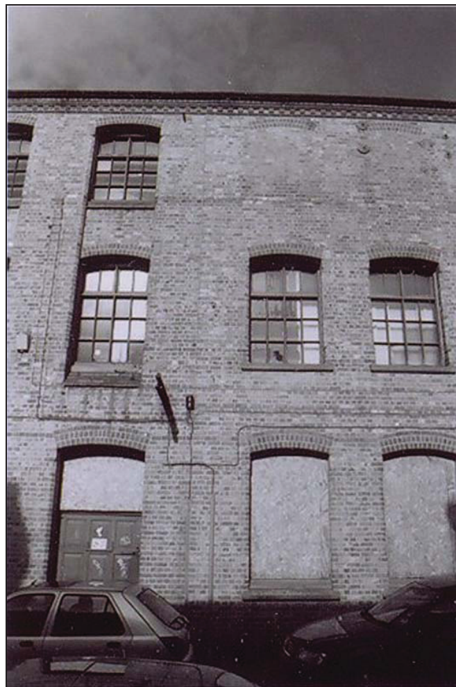
Plate 4. Interface between no.s 25 and 27 Bede Street (27 is on the left hand side). Looking northwest
