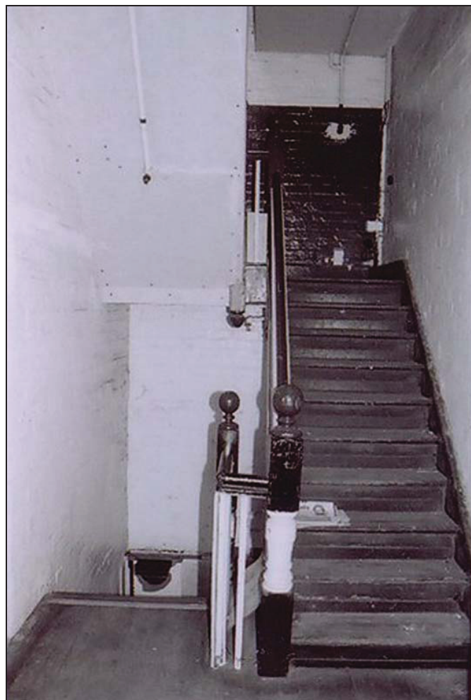
Plate 6. 27 Bede Street. Staircase from 1 st to 2 nd floor. Looking northwest.
