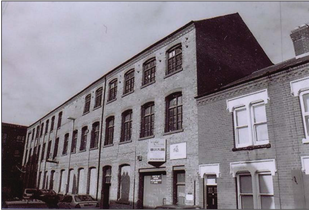
Plate 3. 25 Bede Street. Looking west
