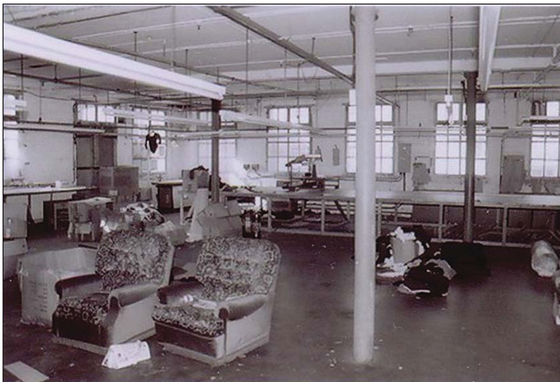
Plate 11. 27 Bede Street, 1 st floor. Looking west.
