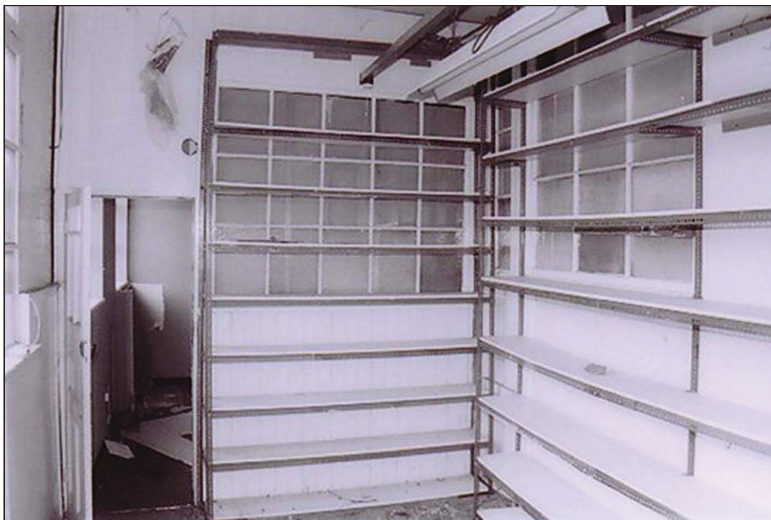
Plate 18. 25 Bede Street, 1 st floor office. Looking southwest.
