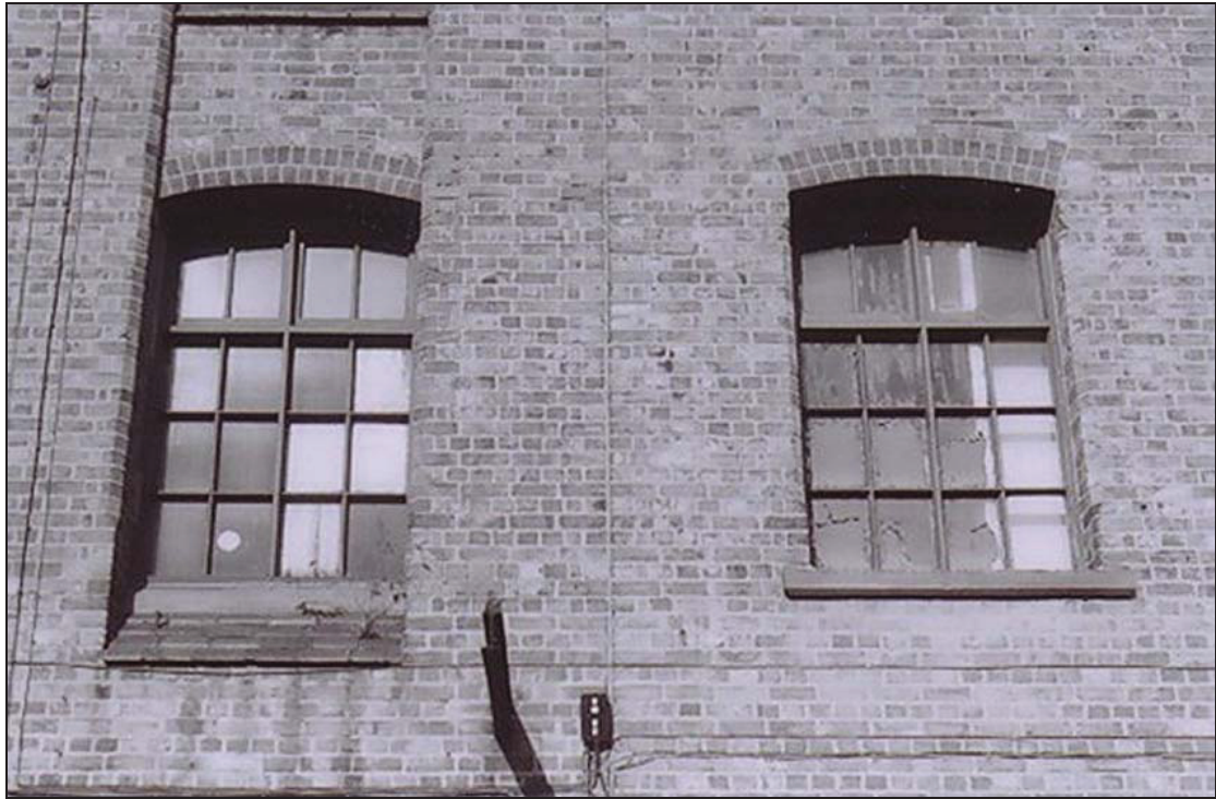
Plate 5. 1 st floor window details (27 is on left hand side). Looking northwest.
