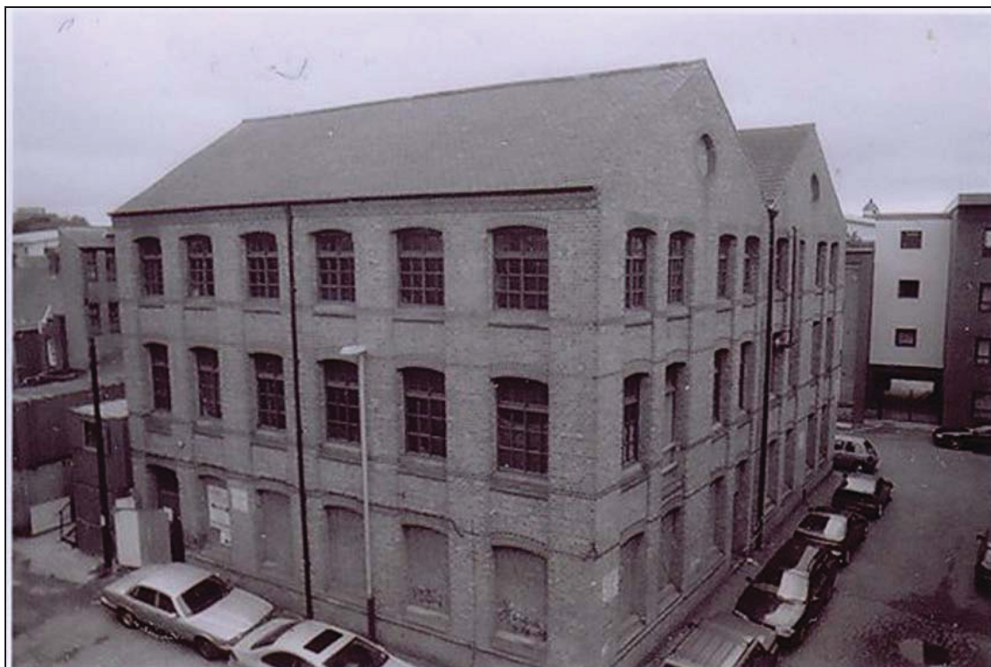
Plate 1. 27 Bede Street. Looking east (taken from fire-escape of adjacent building)
