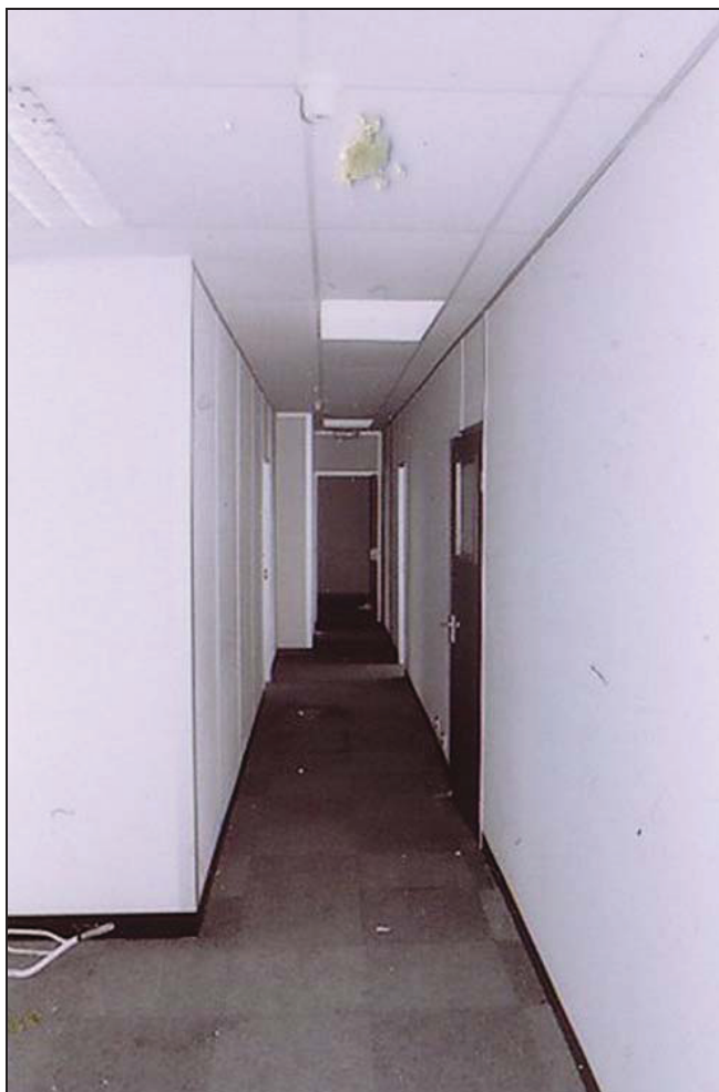
Plate 17. 25 Bede Street, 1 st floor corridor. Looking northeast.
