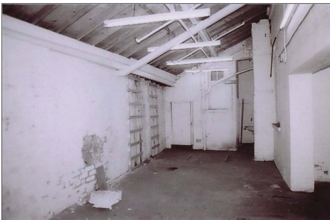
Plate 16. 25 Bede Street, former yard area. Looking northeast
