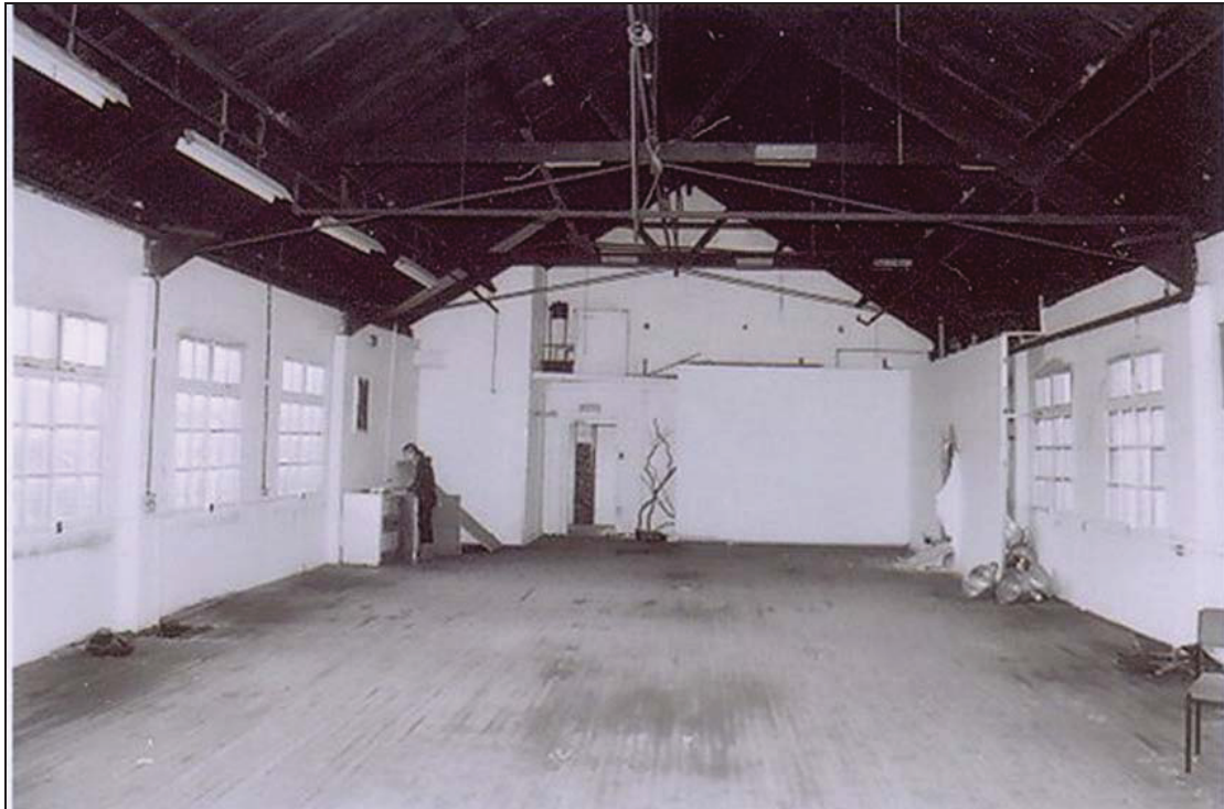
Plate 19. 25 Bede Street, 2 nd floor. Looking southwest.
