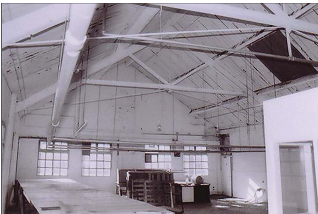
Plate 12. 27 Bede Street, 2 nd floor. Looking southwest.
