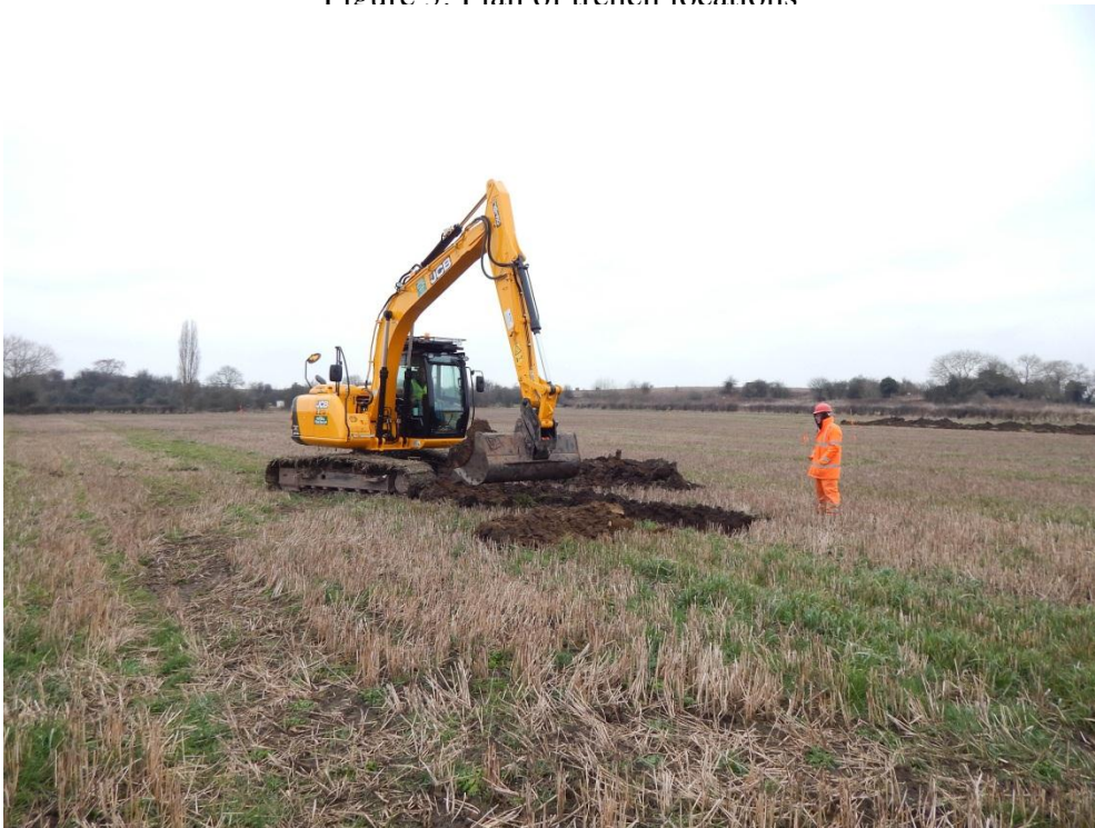
Plate 1: Work in progress, looking north
