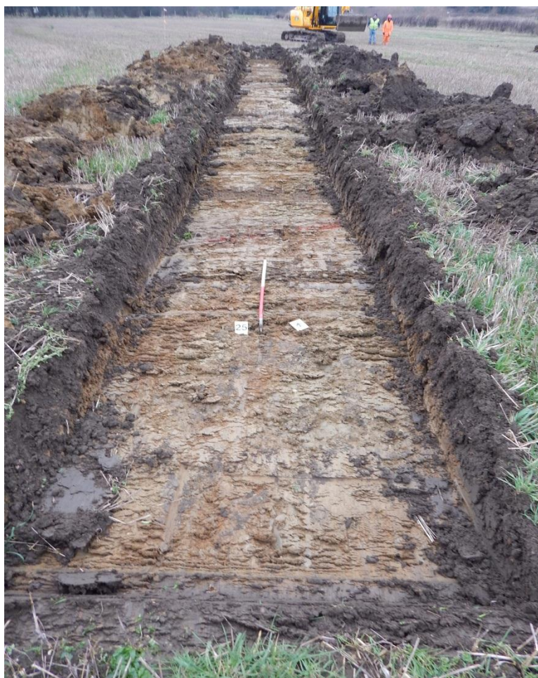
Plate 4: Post-excavation view of Trench 25, looking north-east
