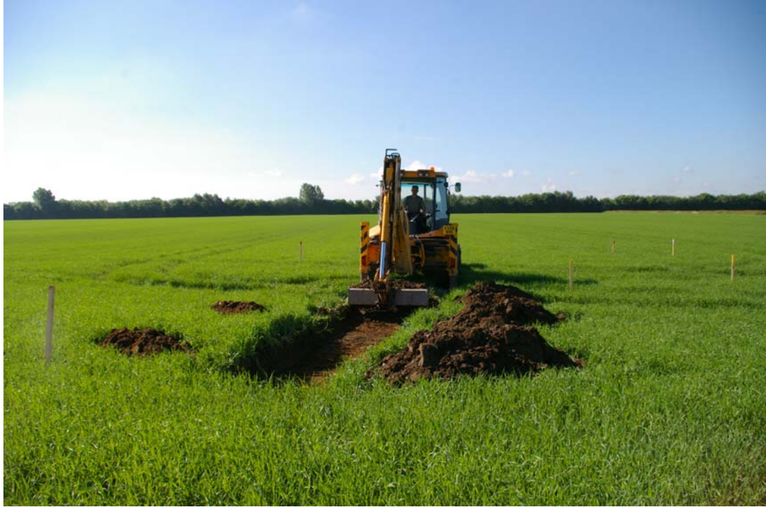
Plate 6: Work in progress, Trench 25, looking south
