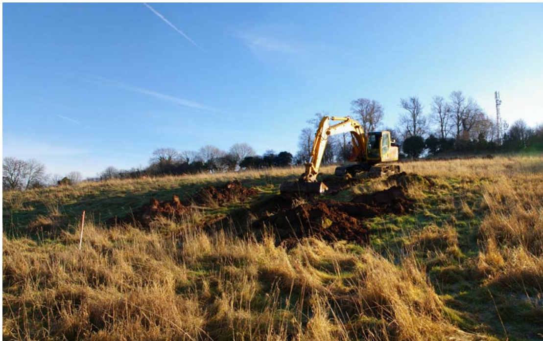
Plate 2: Work in progress on Trench 7, looking south-east
