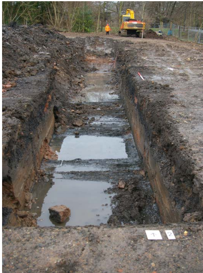
Plate 3: Post excavation view of Trench 2, looking north
