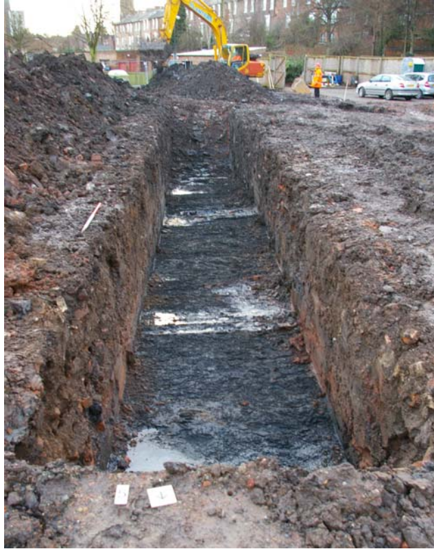
Plate 7: Post excavation view of Trench 5, looking south
