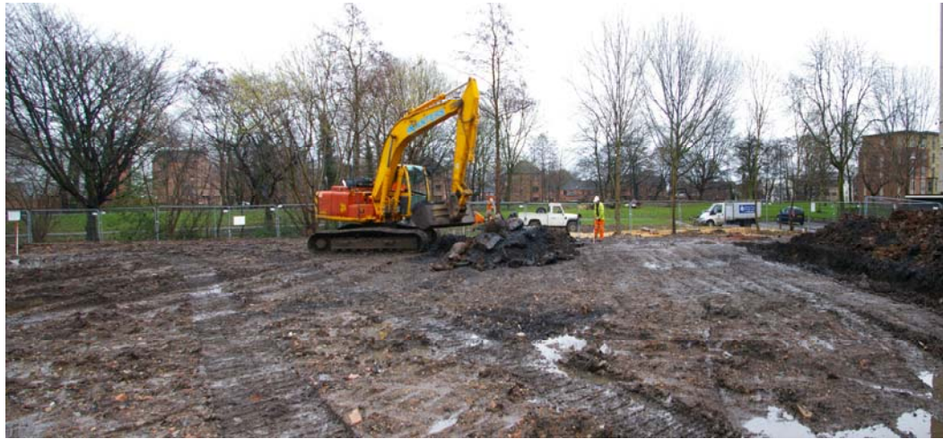
Plate 1: Work in progress on Trench 2, looking east
