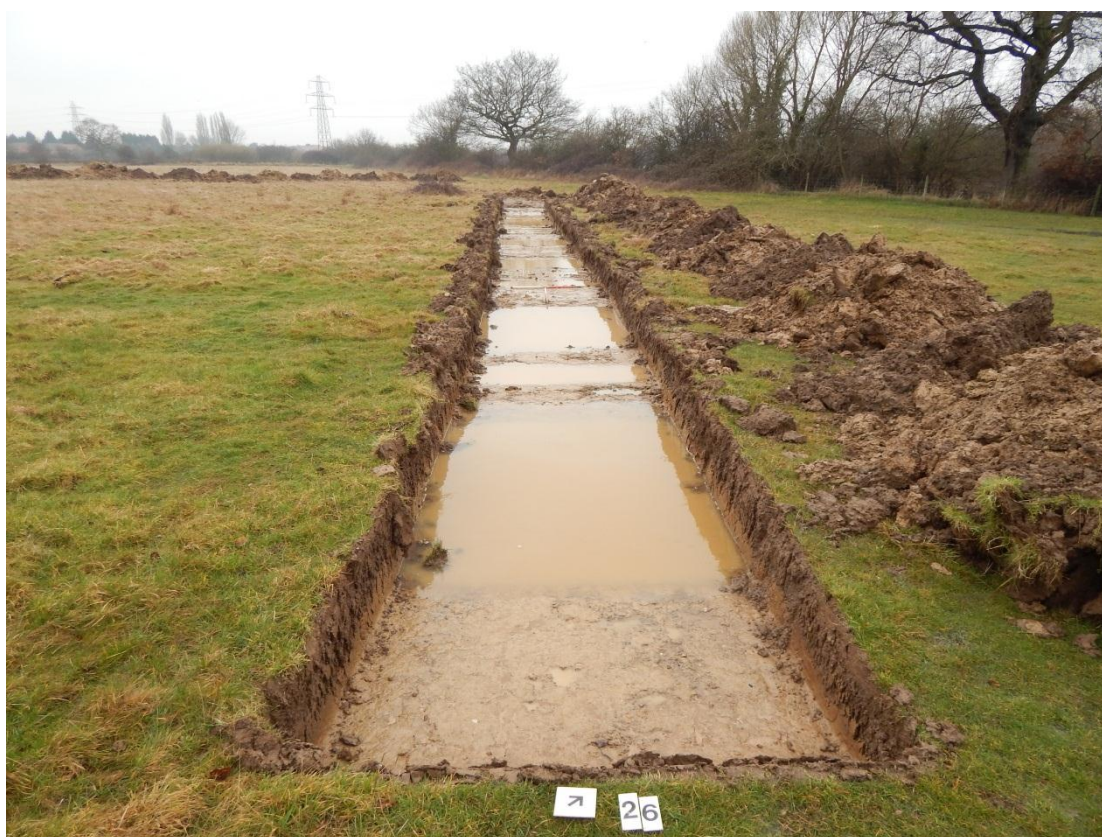
Plate 14: Trench 26, post excavation, looking north-west
