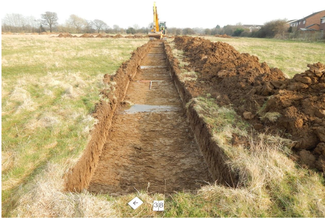
Plate 20: Trench 38, post excavation, looking north-east
