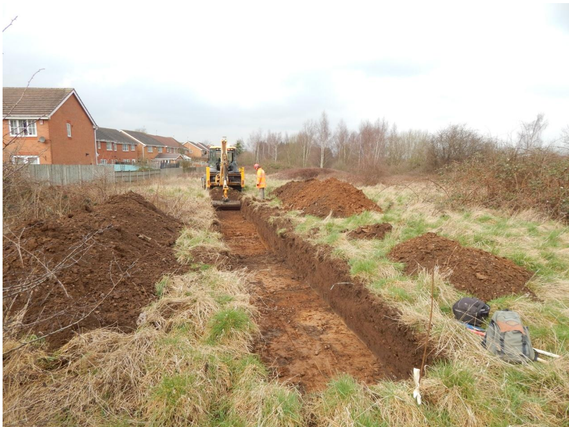
Plate 21: Work in progress in Field 6 on Trench 40, looking west
