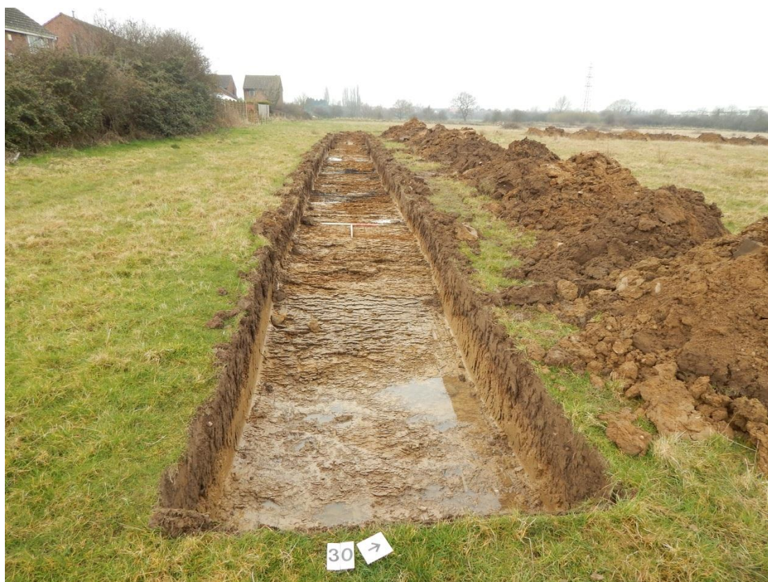
Plate 16: Trench 30 post excavation, looking west
