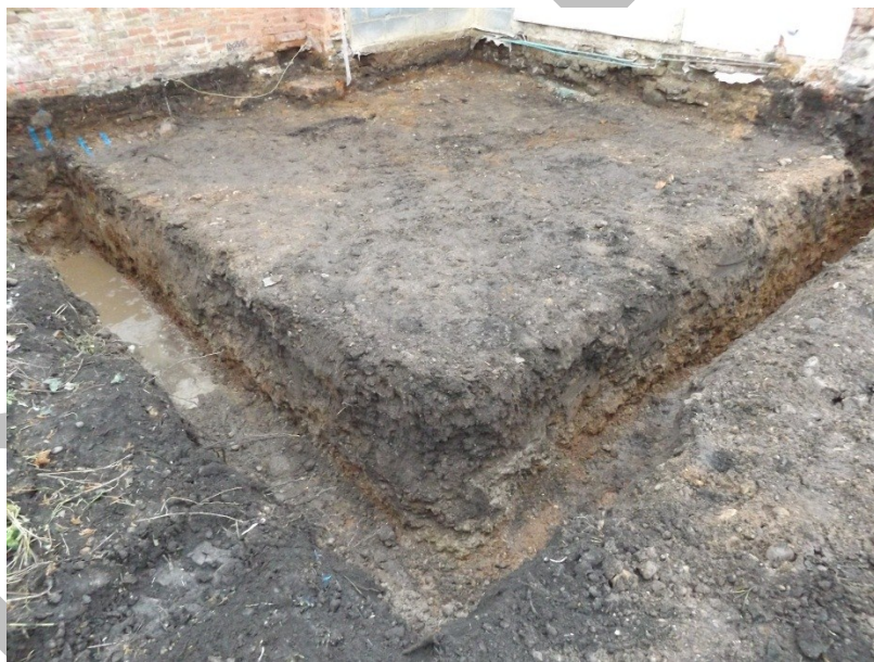
Figure 5. Completed foundation trenches, looking north.
