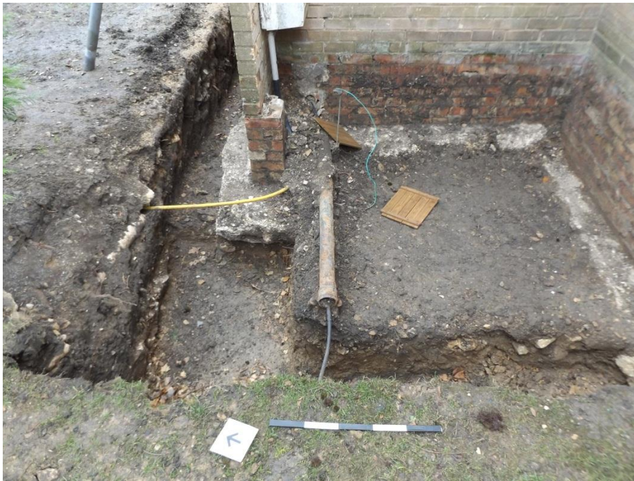
Figure 7. Concrete and made ground in the northernmost foundation trench.
