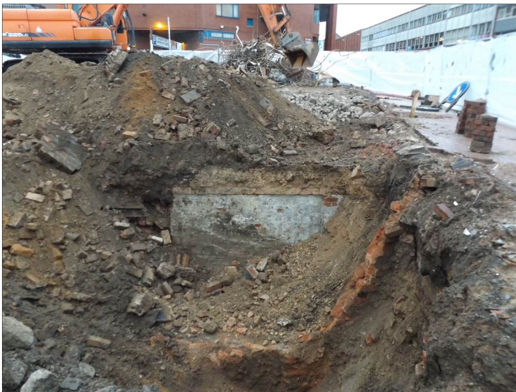
Figure 4: Watching brief area facing South
