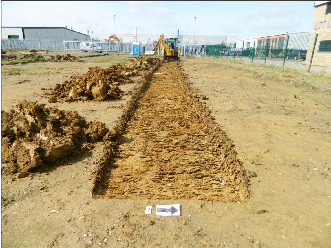
Plate 2: Trenching works being carried out, Trench 7
