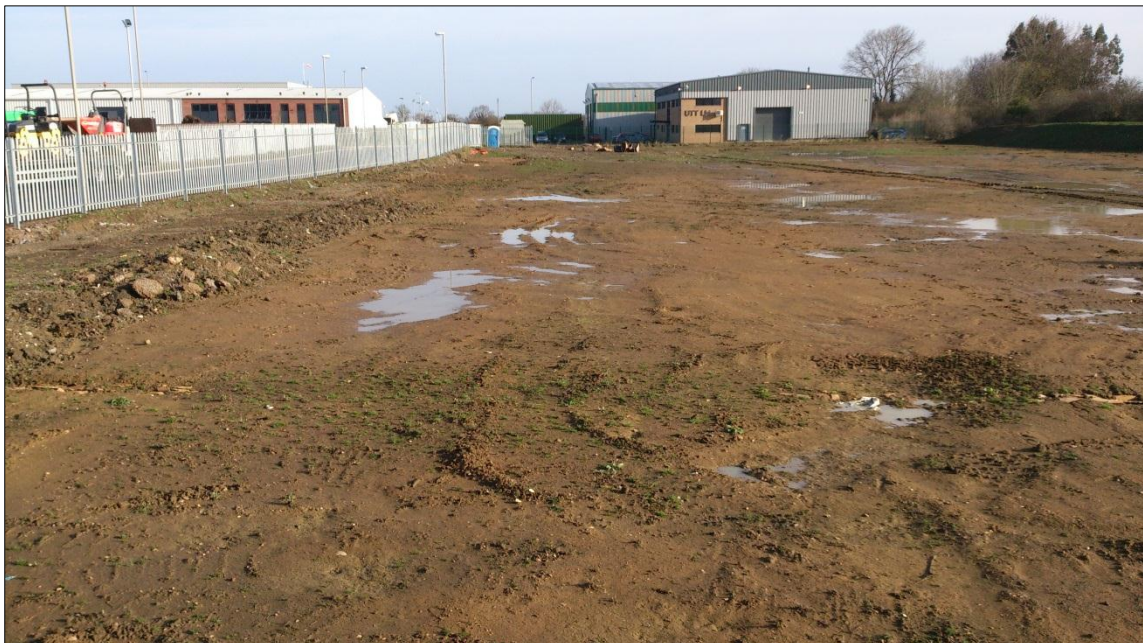
Plate 1: Site area prior to trenching works, looking north
