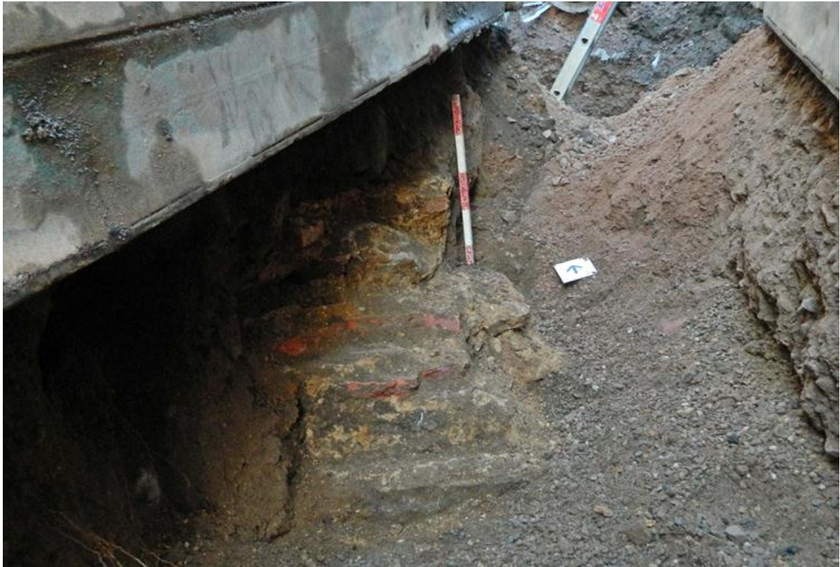
Figure 13 Wall-build (4) to north of Fosse Way metalling.
