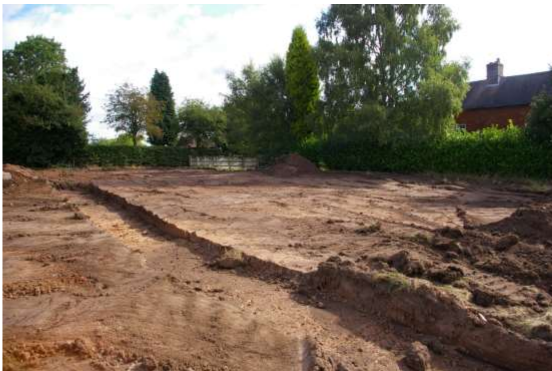
Figure 11 Reducing eastern part of site to formation level Looking north-east
