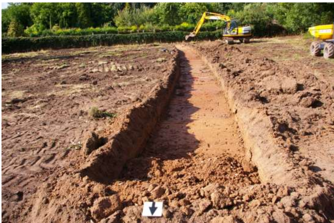
Figure 6 Trench A after excavation Looking south
