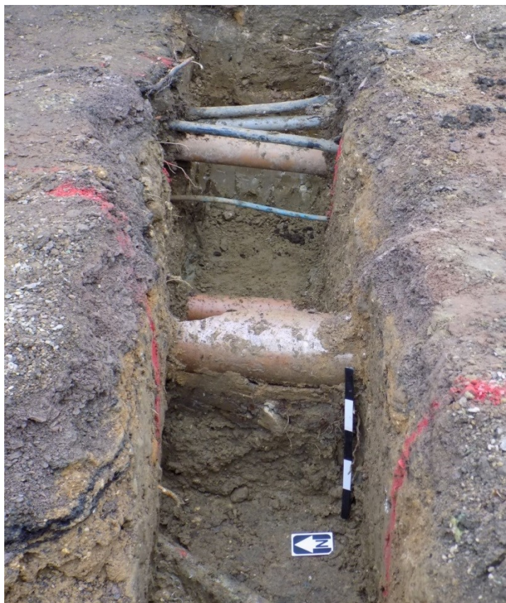
Figure 7 Southern trench showing extent of modern disturbance.
