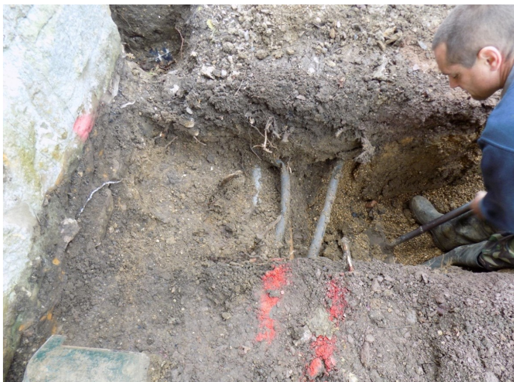
Figure 6 Southern trench showing pipes, drain and pea gravel, looking south.
