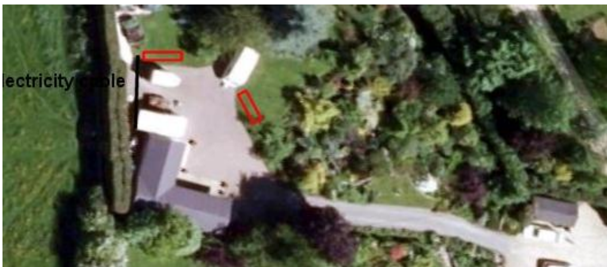
Figure 3: Vertical aerial view of Site showing trench locations.
