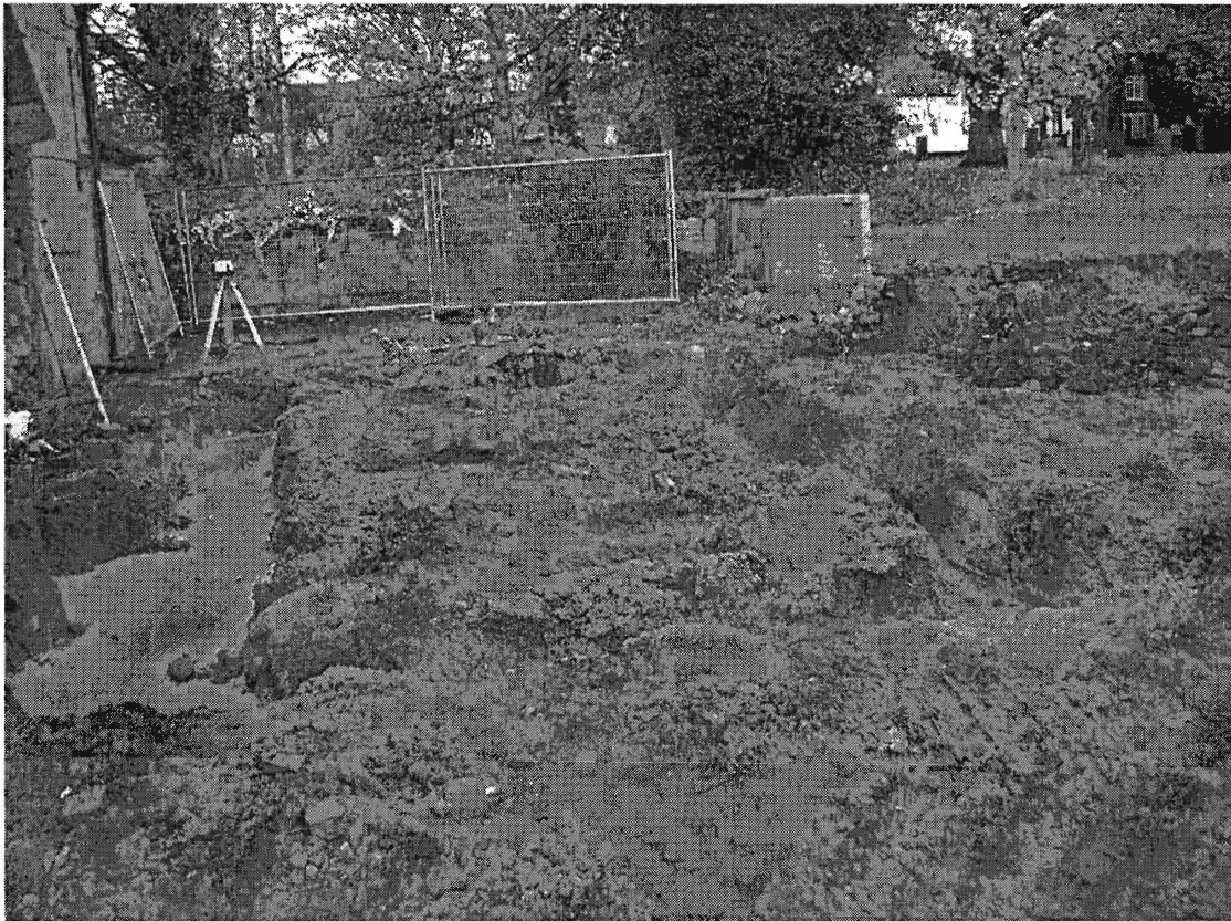
Illus 04 General view of foundation trenches to rear of High Street
