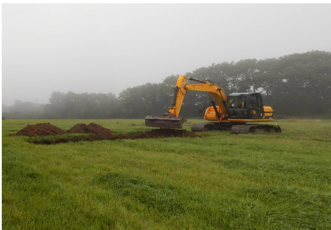
Plate 1: Work in progress, Field 1, looking south-east
