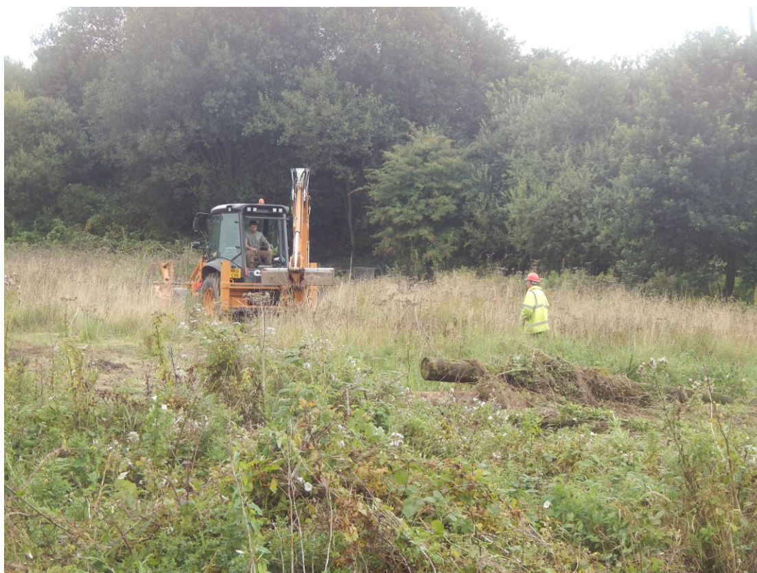
Plate 6: Work in progress, Field 2, looking south
