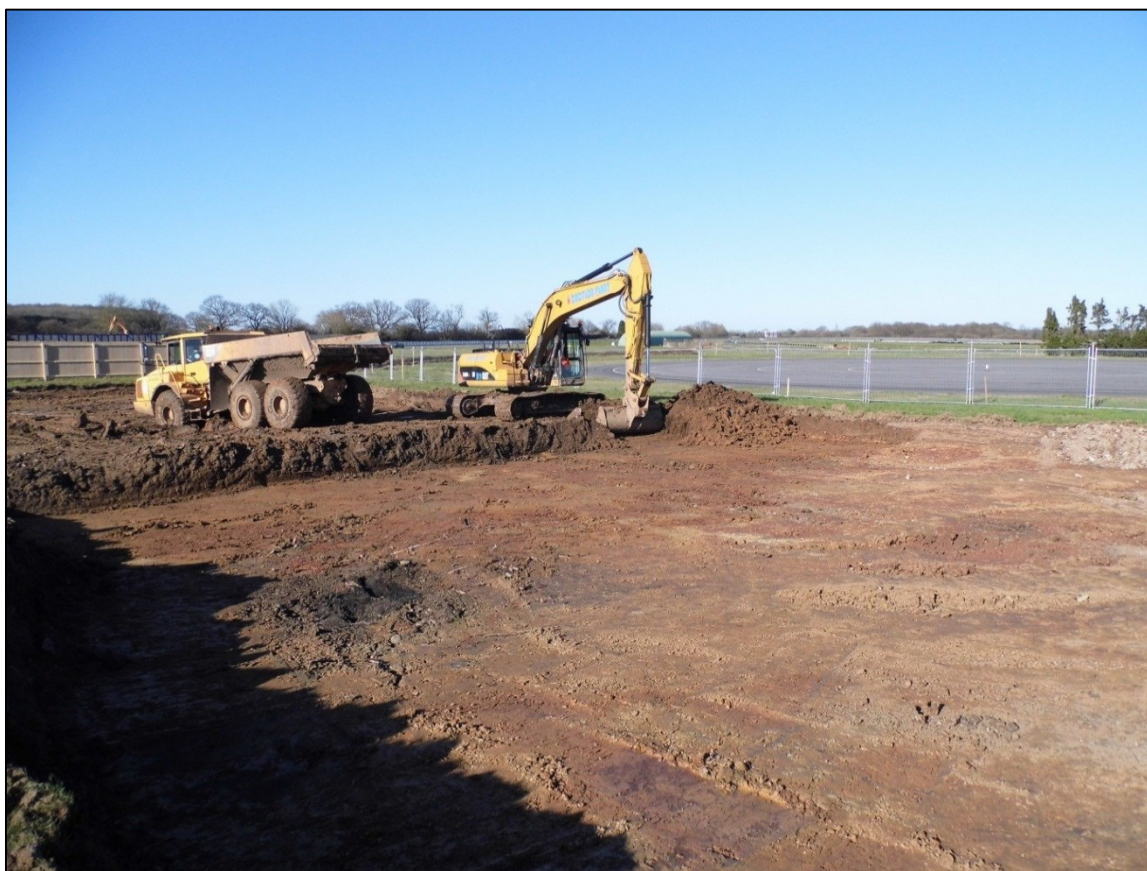
Figure 5: Machine stripping of building footprint, looking north
