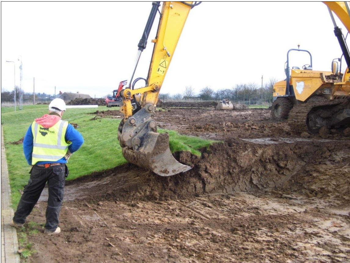
Figure 4: Machine removing turf/topsoil to reveal made ground immediately south-west of existing buildings (Phase 1).
