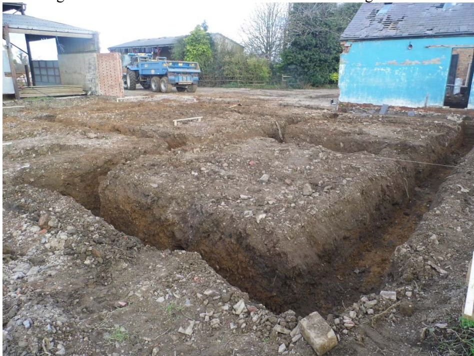
Figure 5: Foundation trenches looking north
