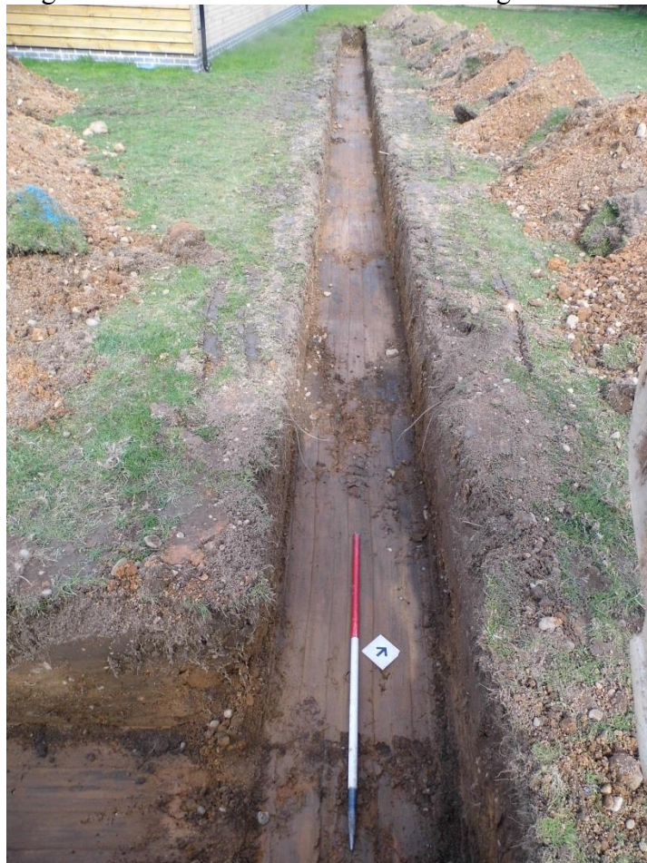
Figure 7: New foundation trench looking north-west
