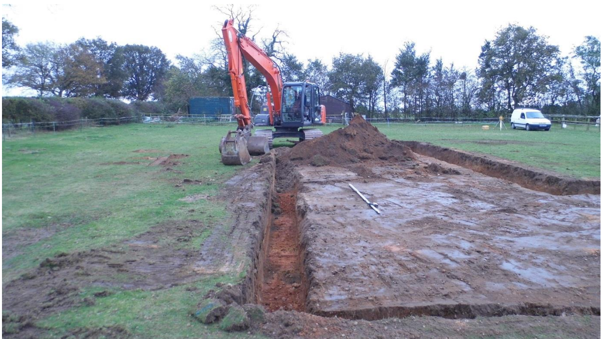
Figure 5: Reduced level of building interior
