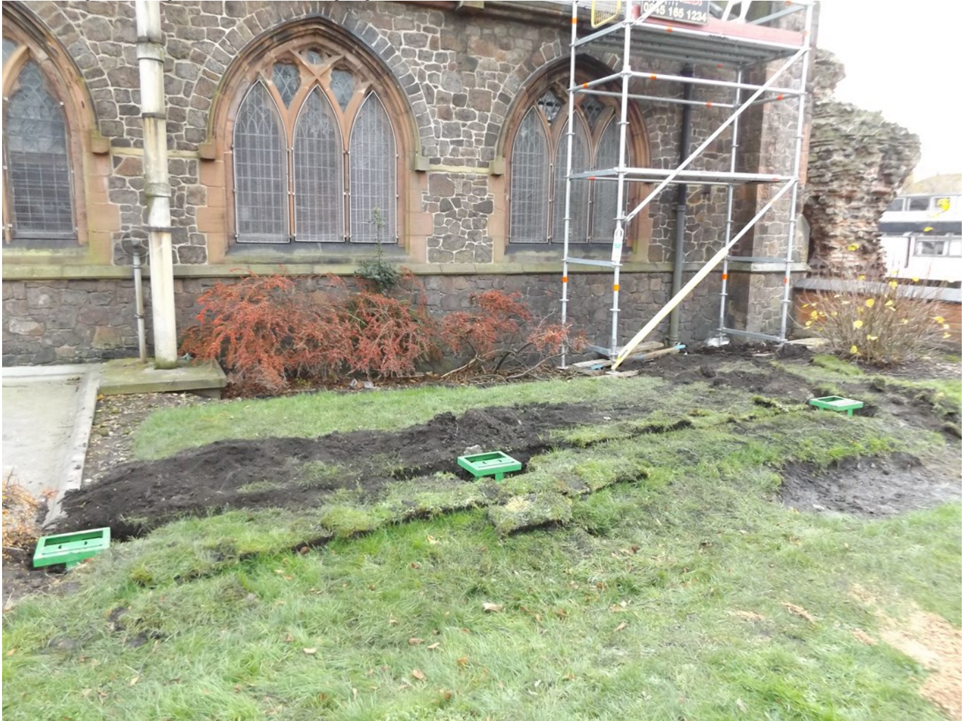
Figure 6: Showing the excavation of Trench 6 and the proximity to Jewry wall.
