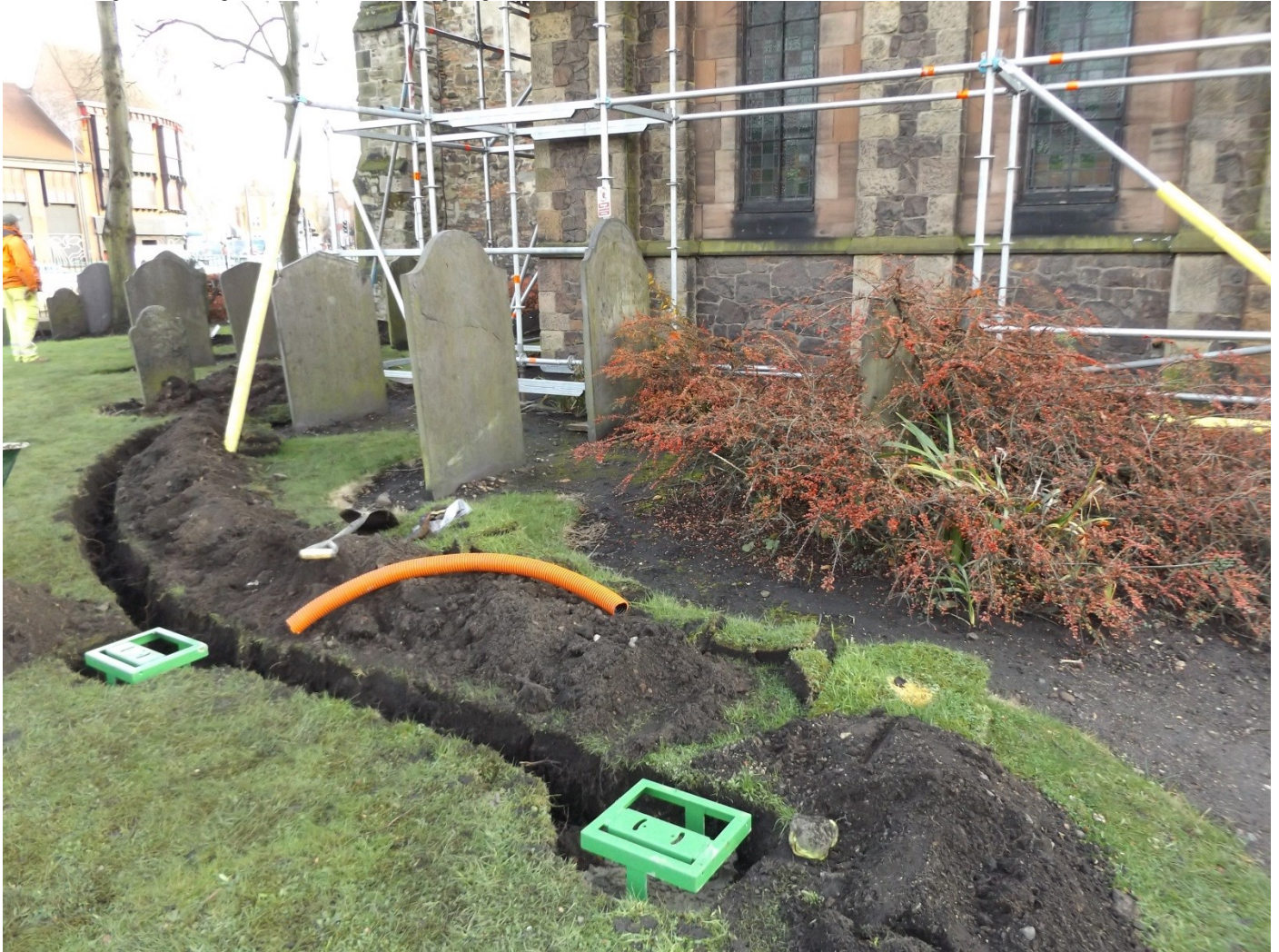
Figure 5: Showing the excavation of Trench 5.
