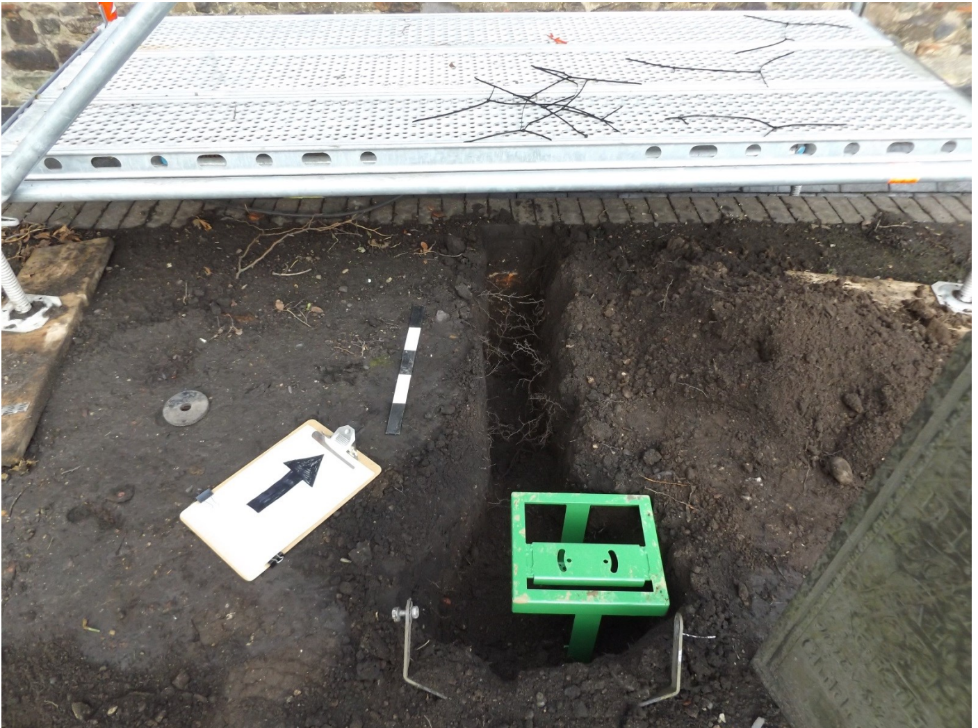
Figure 2: Showing Trench 1 from the southern side of the church.
