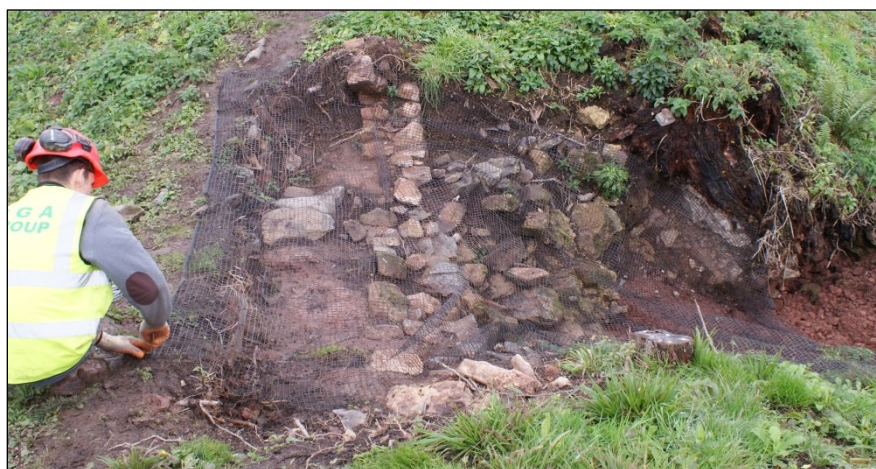
Figure 8. Installation of the GeoGrid membrane and so securing the bank core.
