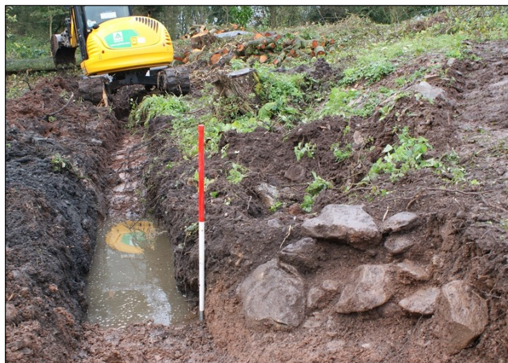
Figure 6. Masonry observed in section at mid- point of trenching looking west.
