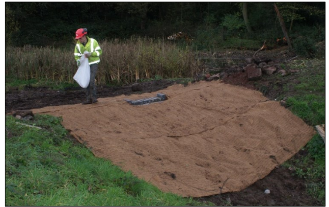
Figure 9. Creation of the spillway looking south west. Covering of gel membrane to the left and laying of coconut mesh around brick spillway to the right.
