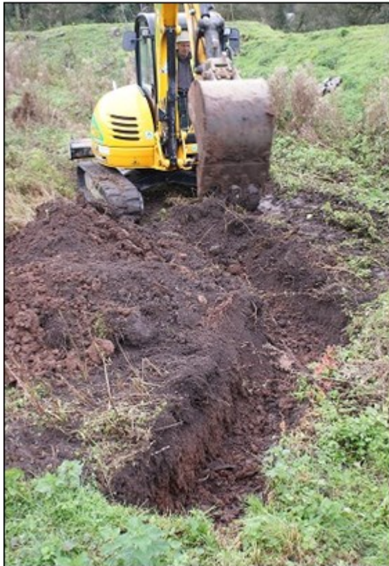
Figure 4. Outset of trenching looking west
