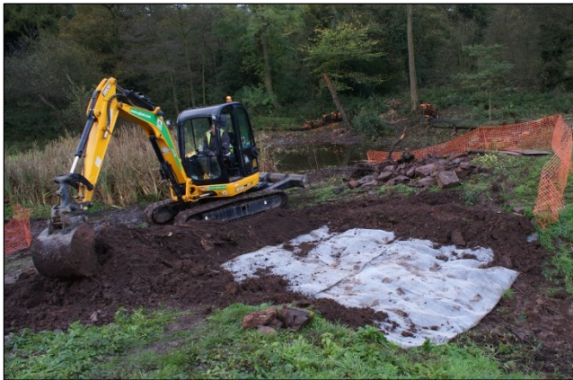
Figure 9. Creation of the spillway looking south west. Covering of gel membrane to the left and laying of coconut mesh around brick spillway to the right.
